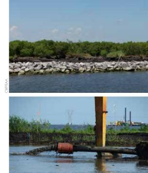
The simplicity of many coastal restoration ideas – build a rock barrier to keep waves from washing away a shoreline, or pipe sediment into shallow water until land emerges – belies the complexity of their execution. Over the years CWPPRA projects have tested approaches and techniques to answer myriad how-to and why questions and advance the science and engineering of coastal restoration.
