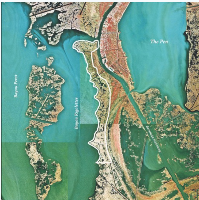
Barataria Basin Landbridge Shoreline Protection, Phase 4 (BA-27d).
