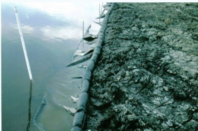
Sediment Containment System for Marsh Creation Demo (LA-09)
