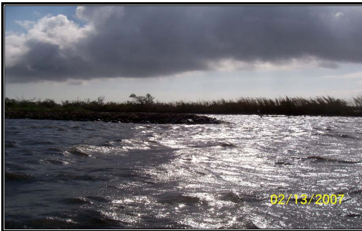
Photo No.8 – (BA-27 CU#6) – end of the rock dike along the east bank of Bayou Rigolettes.
