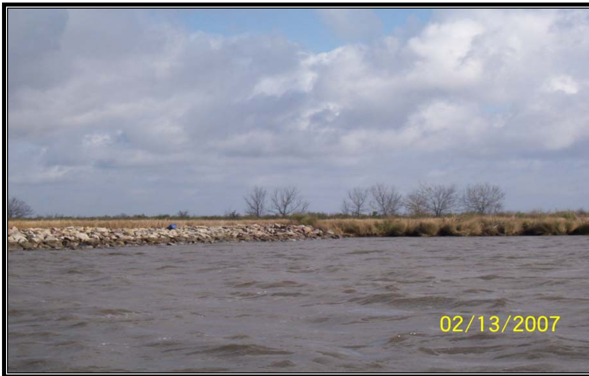
Photo No. 5 – (Ba-27 CU#3) – end of rock dike located on the east bank of Little Lake.
