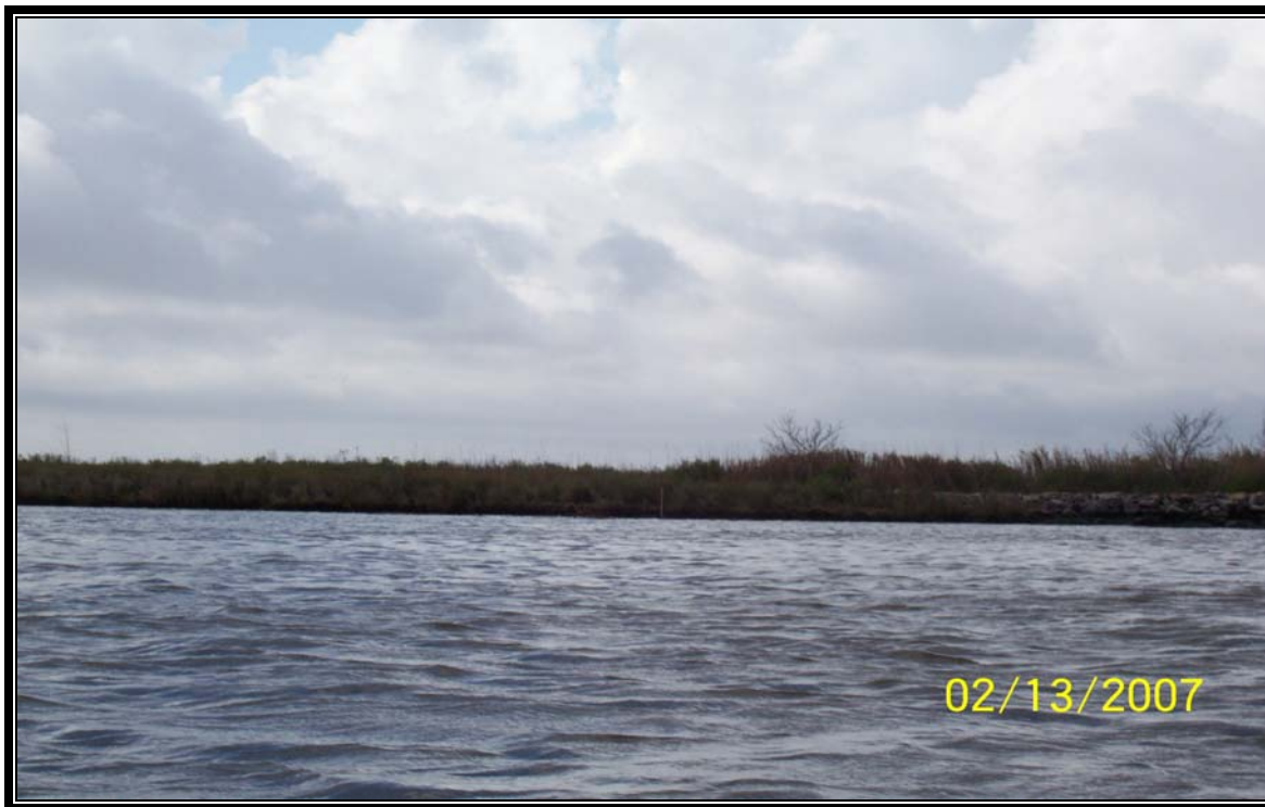
Photo No. 3 – (BA-27 CU# 3) - beginning of rock dike located along the south bank of Bayou Perot.
