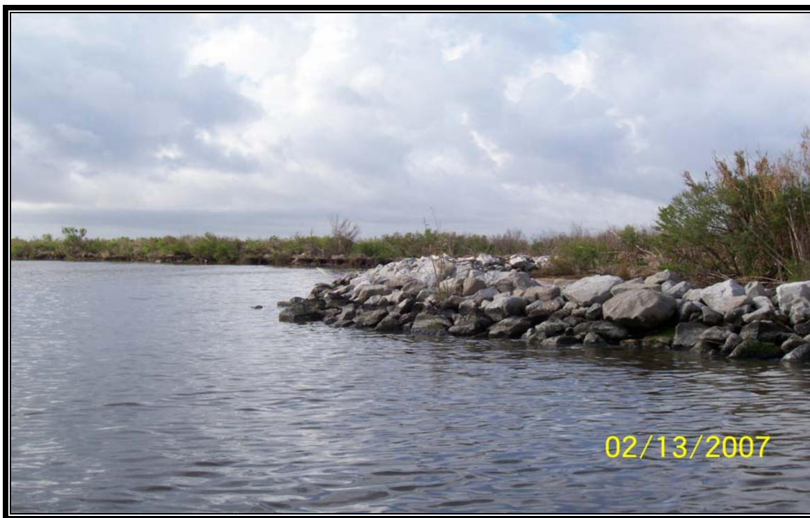
Photo No. 2 – (BA-27 CU#2) – rock dike beginning the west reach in an existing location canal.
