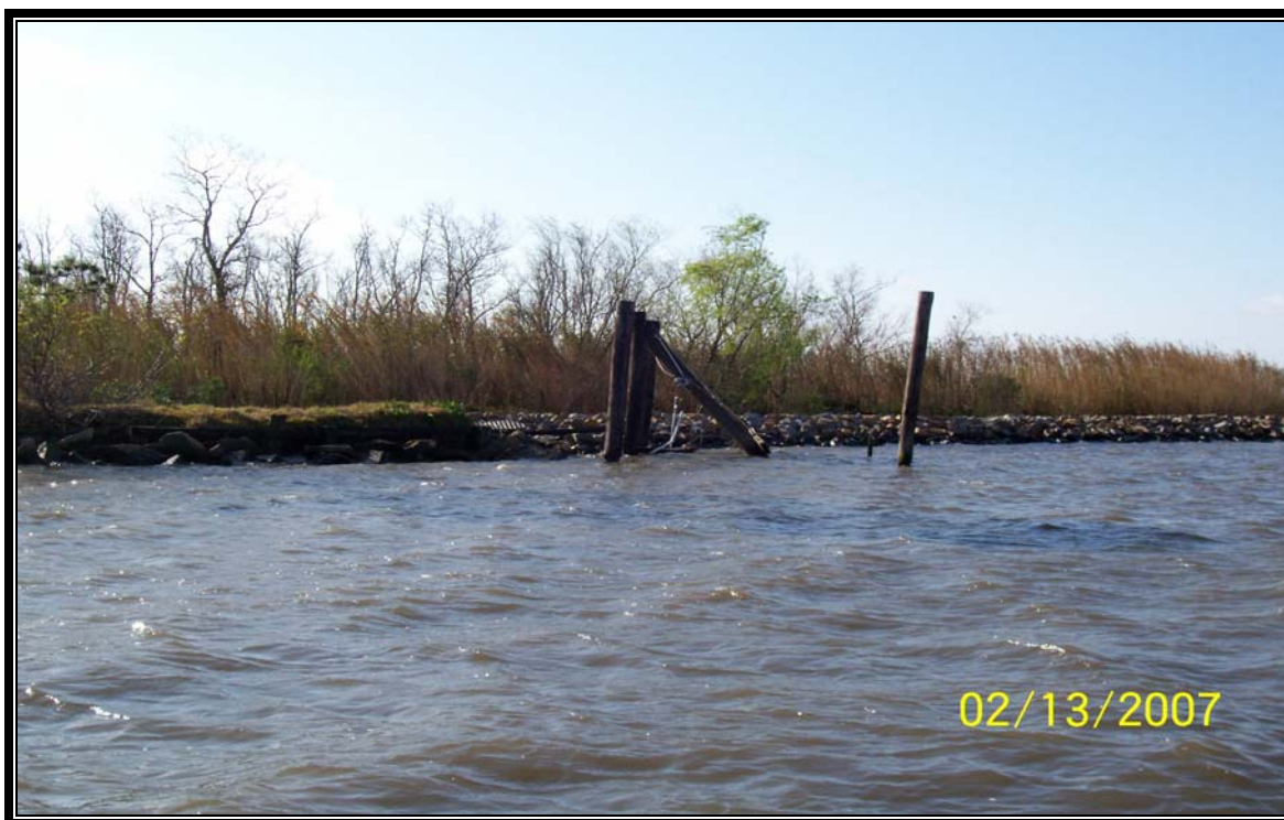
Photo No.6 – (BA-27 CU#6) – rock dike tie-in on the north end of the project near the Barataria Waterway.
