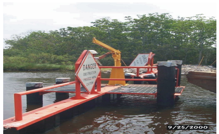
This winch which is permanently attached to the variable crest, water control structure located right off Briton Canal, will help to configure the structure according to a pre-determined water management plan.
