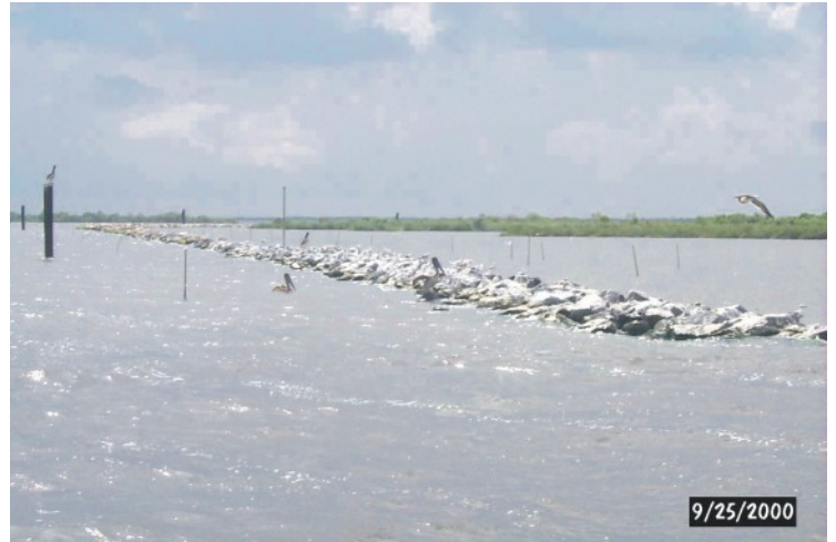
The constructed rock breakwater located in Bay L'Ours will assist in reducing wave energies before they impact the shore and will also arouse the curiosity of local waterfowl such as these pelicans.
