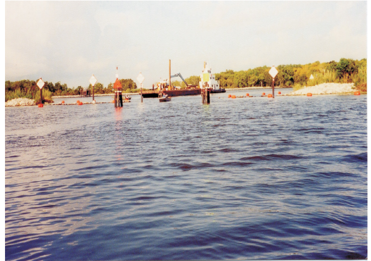
Weirs constructed with a boat bay aid in the effective management of hydrology while still allowing the passage of small boats and vessels.
