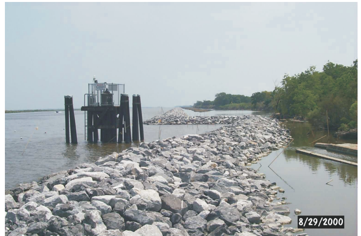
Where existing structures were encountered, such as the crossing of the freshwater delivery system to Grand Isle pictured above, the alignment of the structure was altered.
