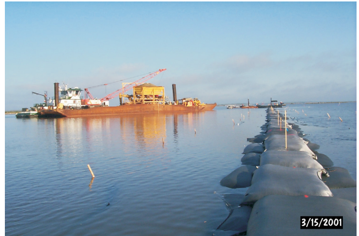
Geo-textile fabric bags were filled with a lightweight aggregate and then sewn closed. These bags act as the supporting core of the shoreline stabilization structure.
