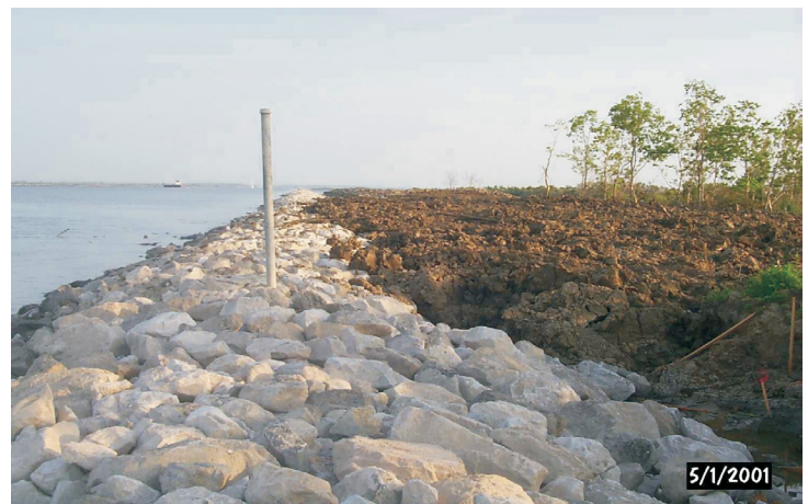
This completed rock riprap structure was placed adjacent to the existing shoreline to buffer it from the erosive forces of wake-induced wave energy.
