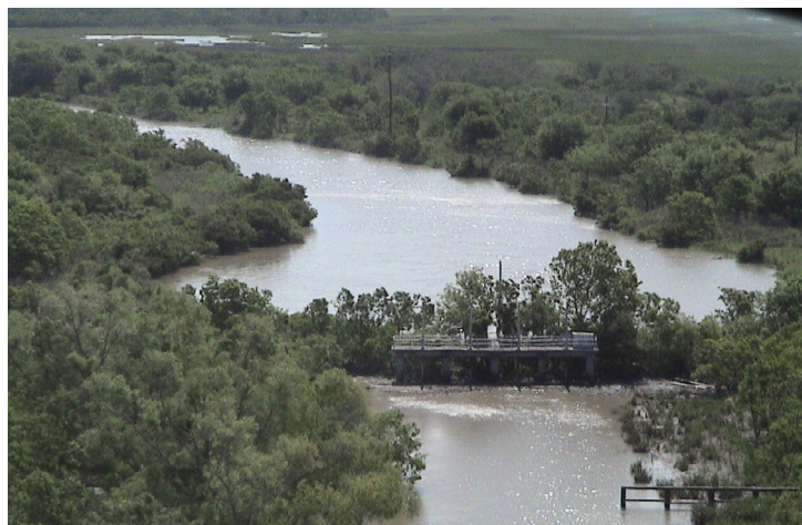
Freshwater diversion structures on Bayou Lamoque, which are in need of repair, will allow water from the Mississippi River to flow through the area's wetlands again when its gates and their mechanical operating systems are removed.
