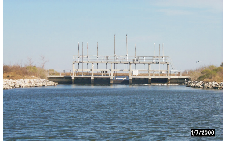
Structures such as this one help regulate the amount of salt water that enters the marsh, improving the health of wetland vegetation.
