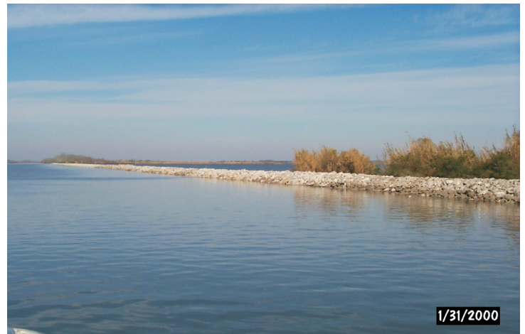
In some areas, the shoreline was non-existent, succumbing to the forces of wave erosion. A new barrier consisting of rock was constructed, ensuring a more natural water flow in the project area.
