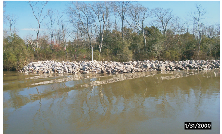
In order to prevent the GIWW from encroaching into the lakes, the thin, eroding shorelines were protected with rock riprap.
