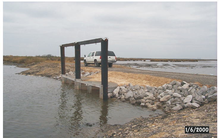
This structure allows the insertion of stop-logs within the openings to regulate water passage. During certain times, such as storms or hurricanes, stop-logs are removed to prevent damage to the structure and adjoining embankments from high water levels.
