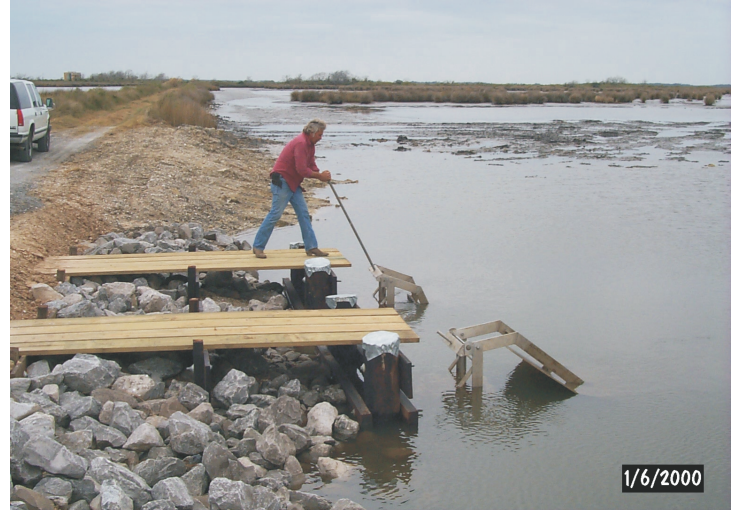
Flap gates on this structure are automatically operated and are opened when salinities allow according to a water management schedule.
