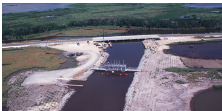
Looking west at the Hog Island Gully water control structure on the Sabine National Wildlife Refuge. The structure has four large 7.5-ft wide by 8-ft deep bays and two smaller 3.5-ft wide by 8-ft deep bays with slide gates. LA Hwy 27 is in the background. The West Cove structure is similar, but with three bays instead of four.
