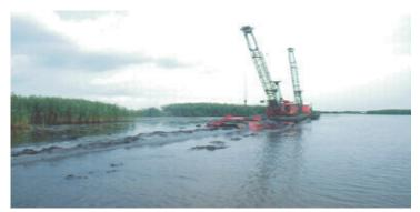
Even though two large pieces of equipment were required to tow the plow through the water, efforts during project implementation showed this method to be less time consuming than utilizing traditional equipment such as a bucket-type dragline.
