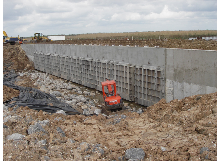
The construction of Black Bayou Culverts included ten 10 foot by 10 foot concrete box culverts under Highway 384 to help with drainage from Black Bayou to the Calcasieu River. The construction of Highway 384 had altered and effectively blocked the original drainage system.
