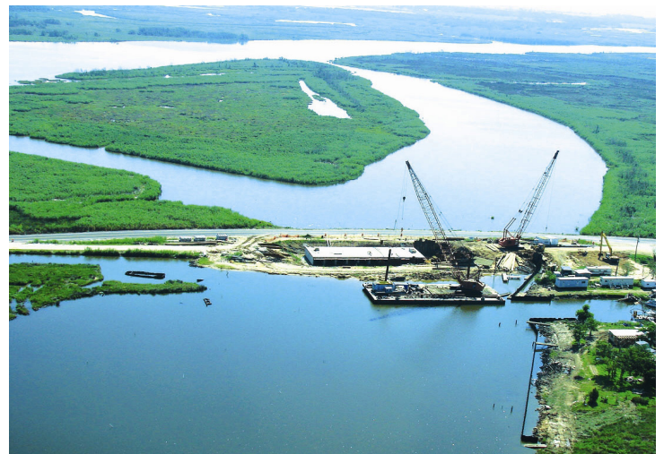
The construction of the Black Bayou Culverts will help the flow of floodwater out of the Calcasieu-Sabine basin while preventing saltwater intrusion from Calcasieu Lake.
