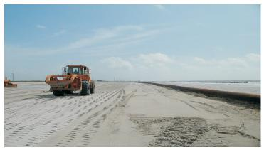
This photo shows the sand material being "dressed" and shaped by mechanical equipment. The required elevation for the "plateau" of the new beach fill is about 5 feet above mean sea level.
