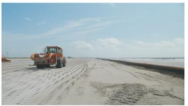
This photo shows the sand material being "dressed" and shaped by mechanical equipment. The required elevation for the "plateau" of the new beach fill is about 5 feet above mean sea level.
