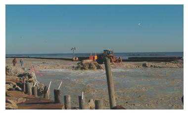
This photo shows delivery of sand material via the pipeline from the dredge "Beachbuilder" and the placement and dressing of the material by bulldozer equipment. The dredge is digging the sand material from the designated borrow area that is located approximately 5 miles offshore.
