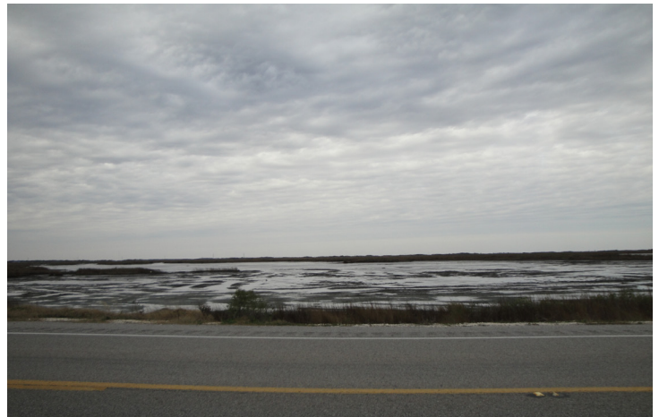
Interior marsh loss along Louisiana Highway 27 exposes the areas only hurricane evacuation route to increased storm impacts. features.
