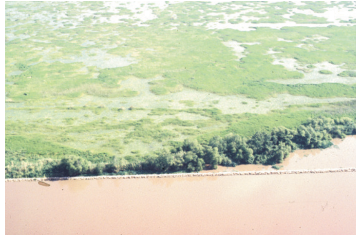
The shoreline protection dike running along the northern shore of the GIWW, Gulf.
