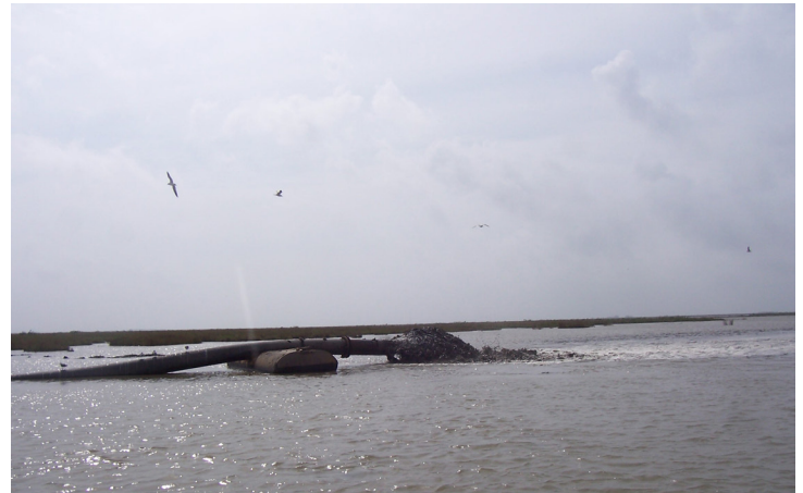
This dredge pipe is rebuilding marsh by depositing sediment dredged from a nearby borrow area. The placed sediment will reach an elevation conducive for growing and sustaining marsh vegetation.
