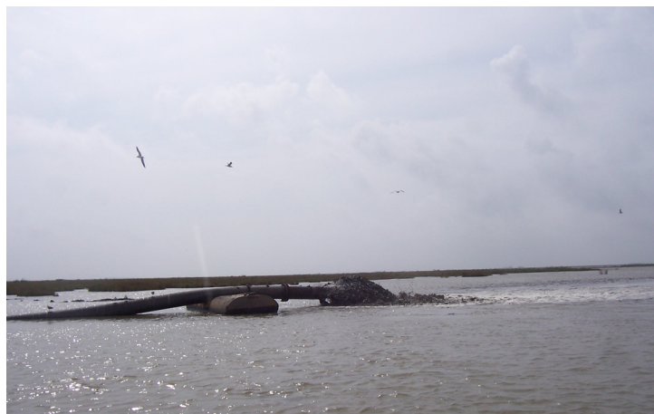
This dredge pipe is rebuilding marsh by depositing sediment dredged from a nearby borrow area. The placed sediment will reach an elevation conducive for growing and sustaining marsh vegetation.
