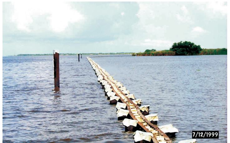
This sheet-pile structure provides protection to the eroding shoreline. Metal caps were placed on the pilings to prevent the rotting of the wood.
