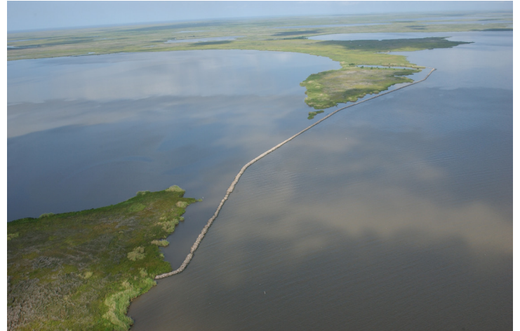
Project features include shoreline protection, canal closures, and isolation of Lake Sand from Vermilion Bay with a rock dike on the northeastern edge of Marsh Island. View is looking west.
