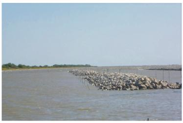
Segmented rock dikes were constructed approximately 200 feet off the shoreline to intercept wave energy before it impacted the beach and caused erosion.
