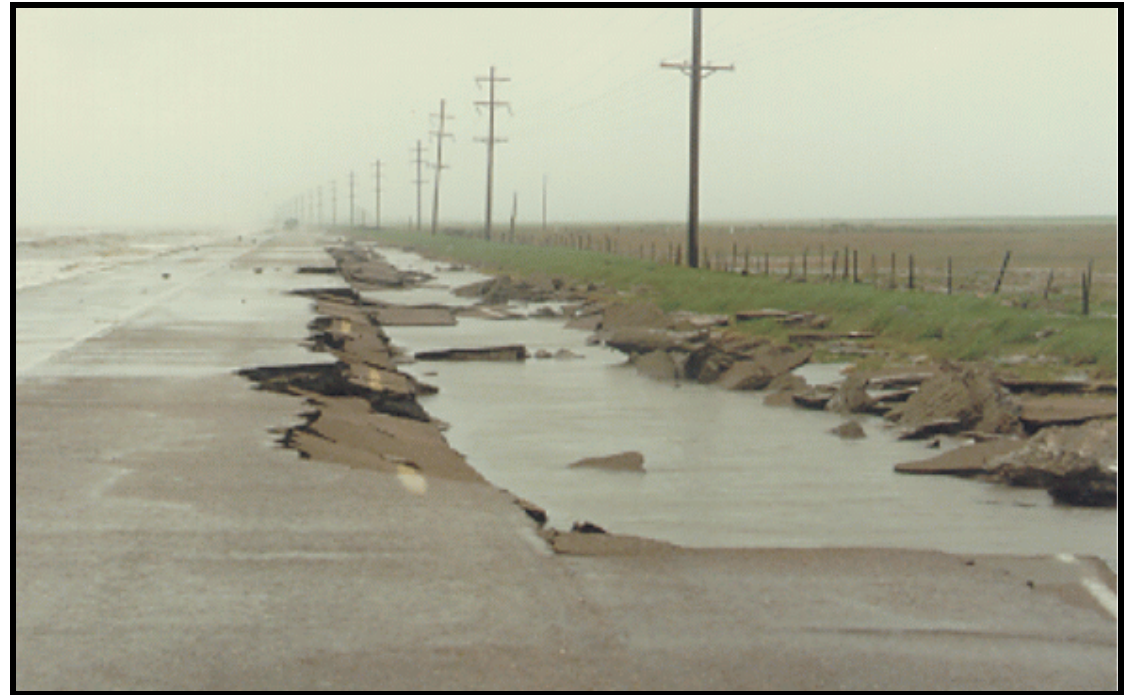
Figure 4. Wave over-wash of the La. Hwy. 82 revetment and roadway during an extreme high tide event showing collapse of the embankment and roadbed beneath the westbound lane of the highway. Image from Underwood et al. (1999).
