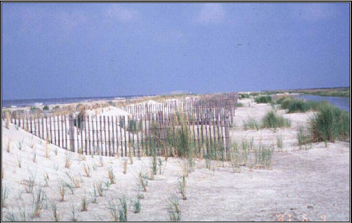
Figure 2. Typical sand fencing with perpendicular spurs at Timbalier Island Plantings Demonstration (TE-18) project (photo taken at Site A, July 1996, looking northwest).
