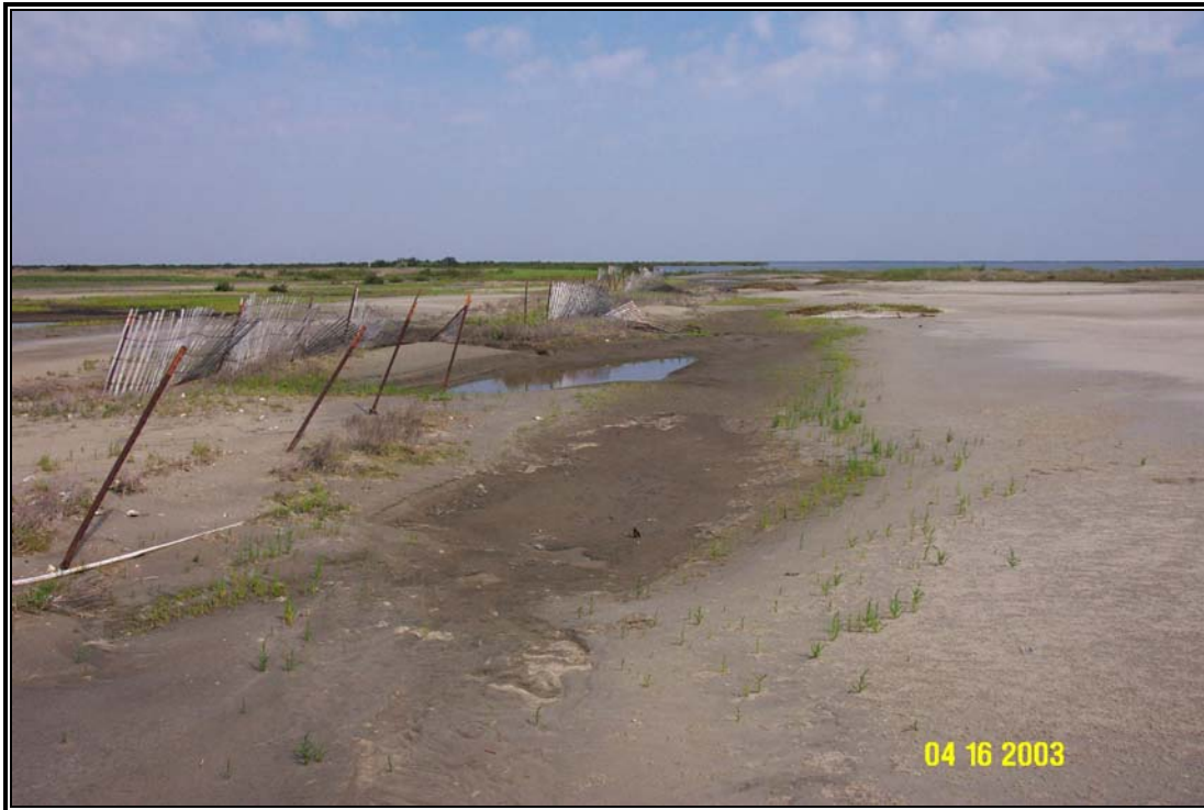
Figure 29. Scour along a sand fence not parallel to shore, on Whiskey Island, LA (LDNR photo, taken April 2003).
