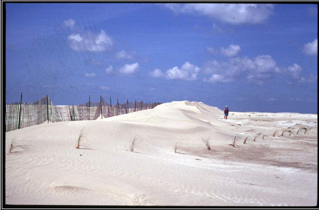
Figure 30. Dune building approximately 1 year after fence installation at East Island Restoration (TE-20) project. Note lower dune in foreground due to bottom of the fence being above sediment surface allowing winds to continue to move sand. (LDNR photo, taken June 1999).
