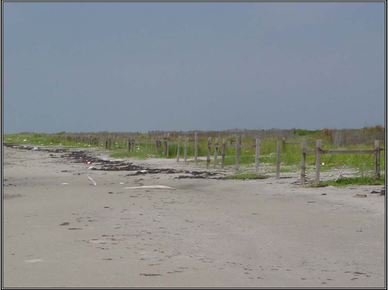
Figure 15. Eastern end of fence at Site B after impacts from storm waves and debris at the Timbalier Island Plantings Demonstration (TE-18) project (LDNR photo, taken September 2001).
