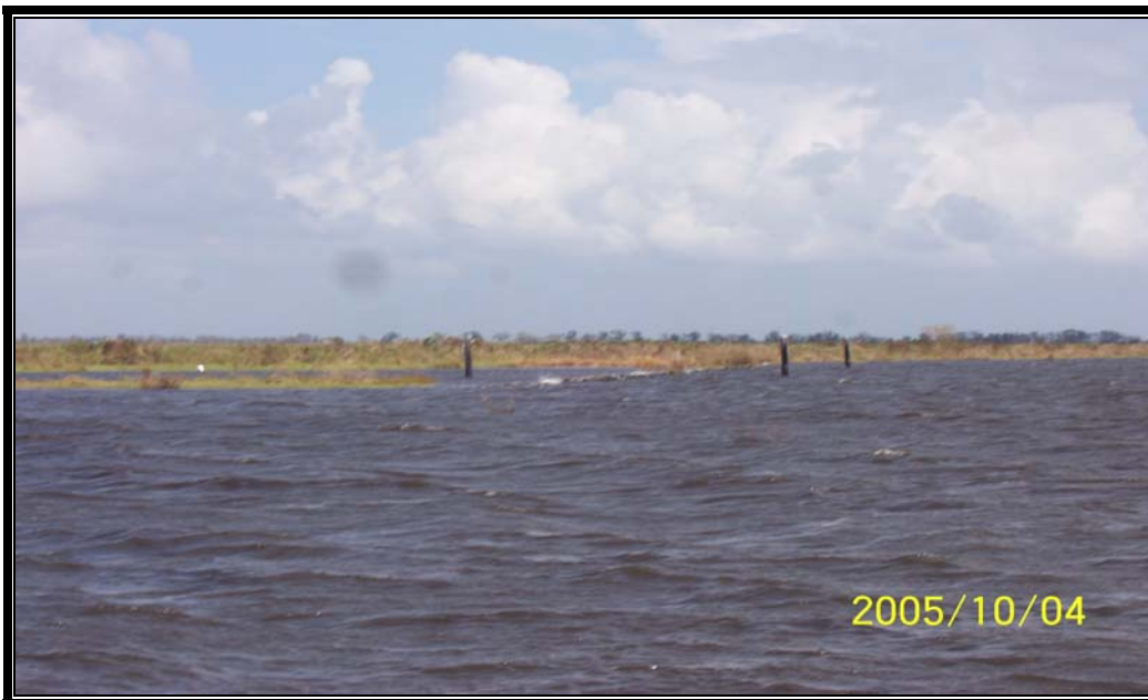
Structure 4A&B – large section of marsh eroded around the south side of the existing rock plug creating a breach allowing unimpeded flow behind structure looking north.
