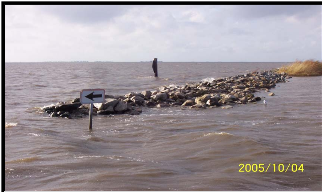
Structure 14A – displaced rock along rock weir south end of barge bay (Post Hurricane Rita). Water level reading at time of inspection was approximately +2.25' NAVD.
