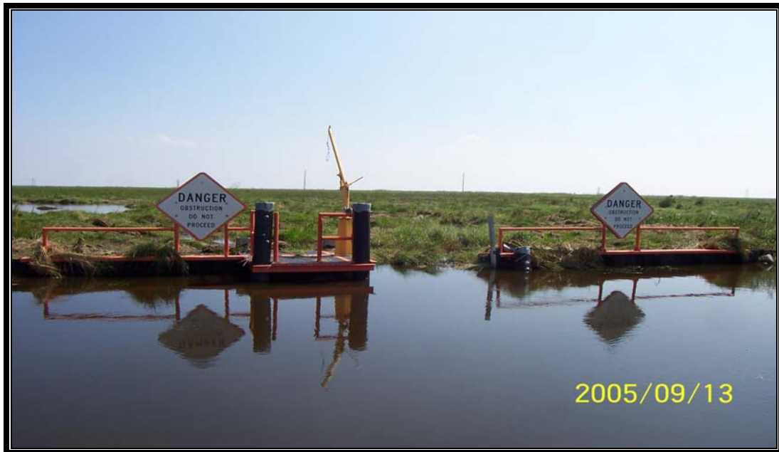
Structure #35 – movement of marsh behind structure blocking flow through structure (Post Hurricane Katrina). Water level at time of photo was approximately 1.5' NAVD.
