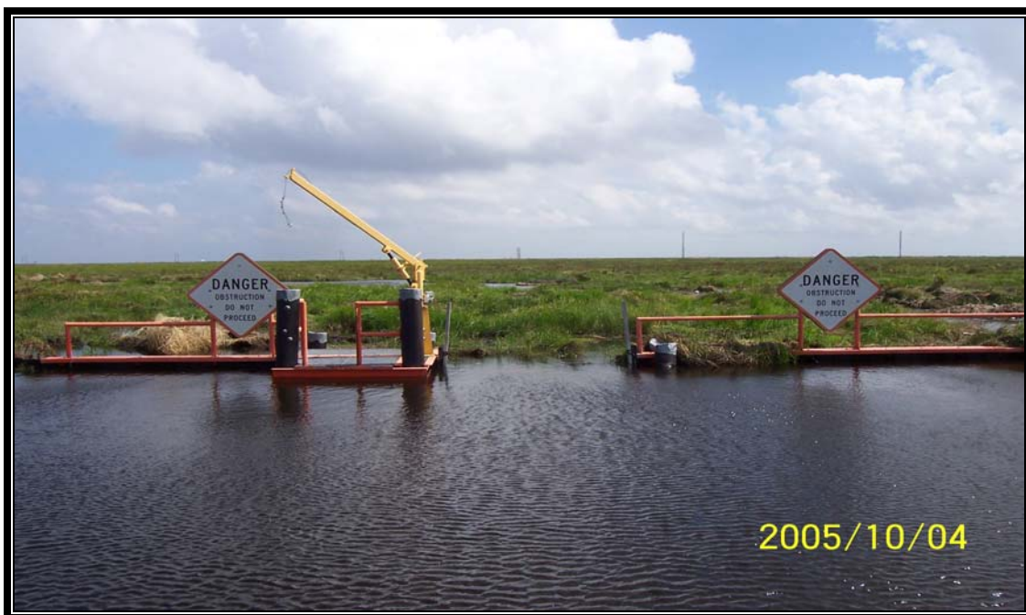
Structure #35 – movement of marsh behind structure blocking flow through structure (Post Hurricane Rita). Water level at time of photo was approximately 1.5' NAVD.
