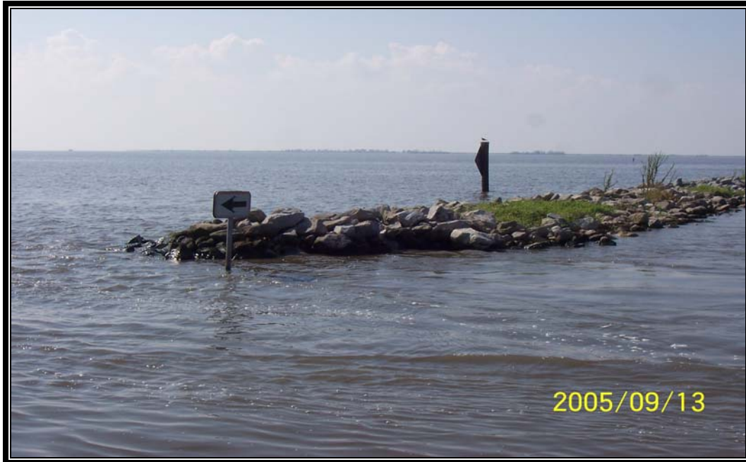
Structure 14A – displaced rock along rock weir south end of barge bay (Post Hurricane Katrina). Water level at time of photo approximately 1.6' NAVD.
