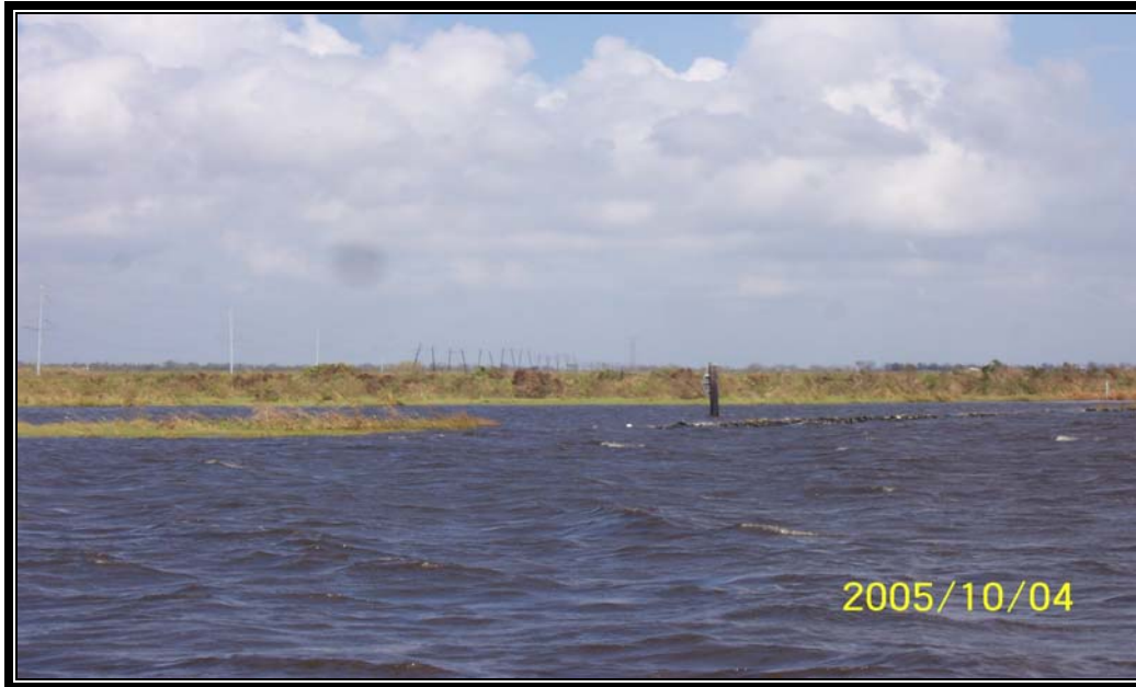
Structure 4A&B – large section of marsh eroded around the south side of the existing rock plug creating a breach allowing unimpeded flow behind structure looking northwest.
