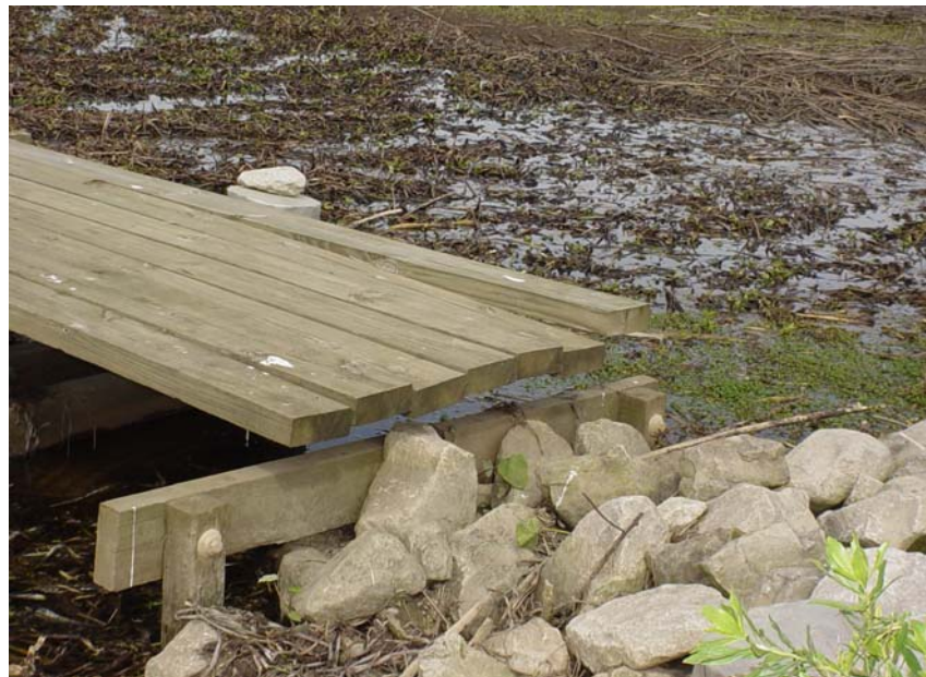
Photo # 2 Site 13 (view 2) This photo is from the 2005 Inspection. The entire structure along with rock closure, gate and walkway are covered with storm debris.
