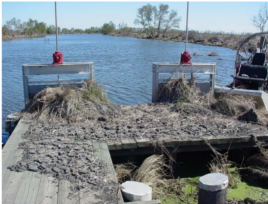
Photo # 16 Site 54 (view 2) This view taken from the structure looking west. The flow meter and all attachments were destroyed by the storm.
