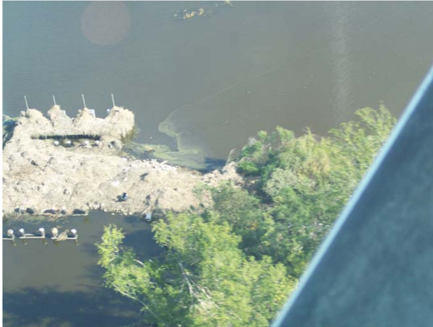
Photo # 5 Site 26 (view 1) Structure is entirely covered with storm debris.
