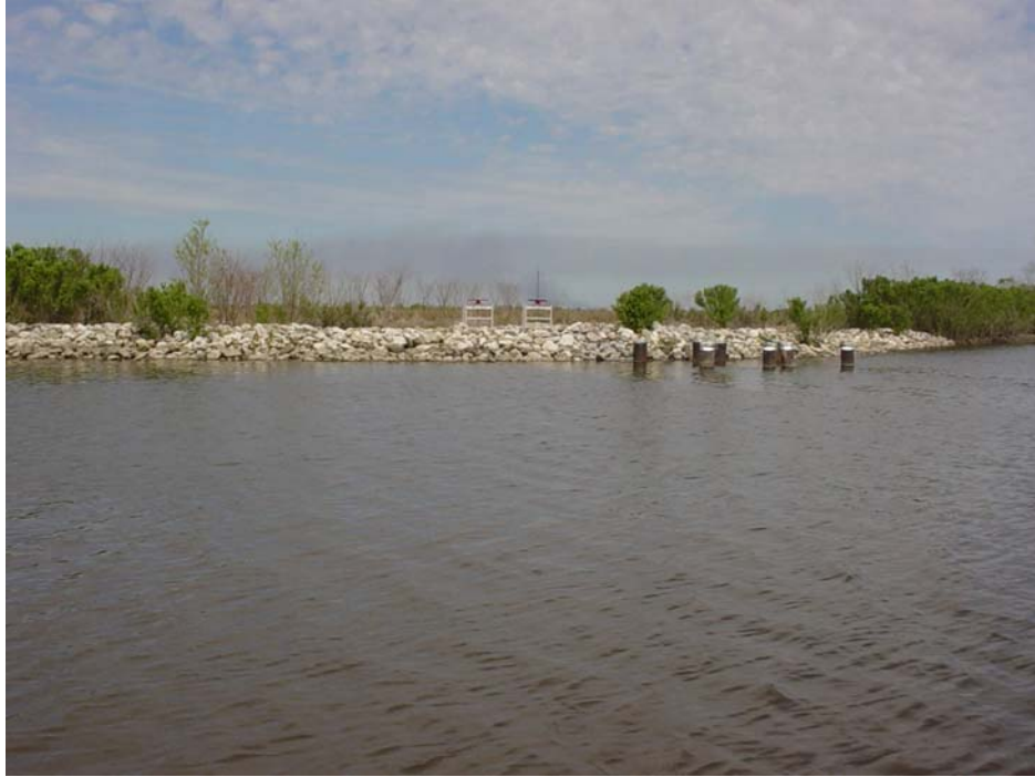
Photo # 21 Site 60 Entire structure is in excellent condition in this 2005 inspection photo; however, the entire structure is covered with storm debris.
