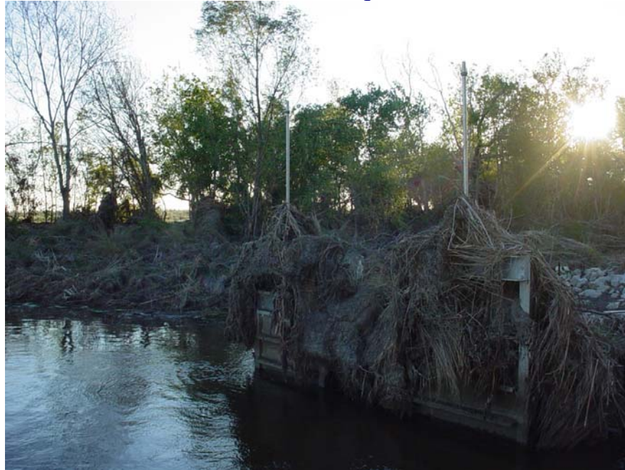
Photo #4 Site 25 (view 2) View from the structure looking South. As noted, the entire structure, including the rock closure is covered with storm debris.
