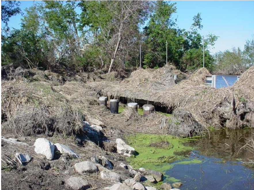
Photo # 6 Site 26 (view 2) A flow meter was installed on this structure. The recorder box was also located on one of the piling. None of the equipment was recovered.
