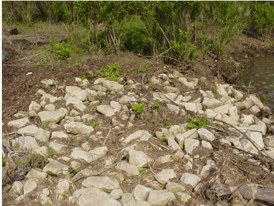
Photo #12 Site 50 (view 2) Slight erosion is evident on both sides of the rock plug where it ties into the earthen embankment.
