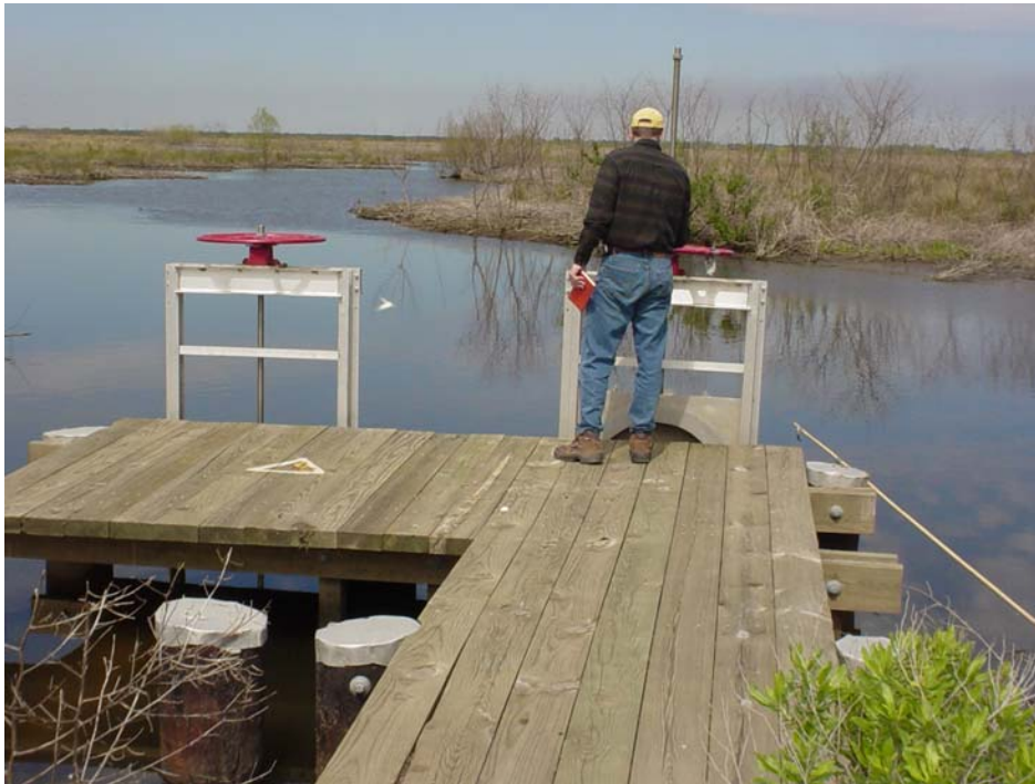
Photo # 22 Site 60 The decking at the structure site is in excellent condition in this 2005 inspection photo. The entire structure and inflow channel are inundated with storm debris and floating marsh balls.
