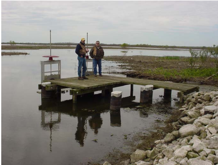
Photo # 13 Site 52 This photo is from the 2005 inspection The entire structure is now covered with storm debris. The culvert is completely blocked.
