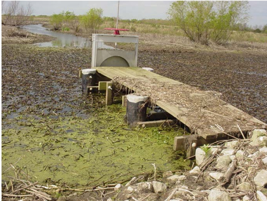
Photo # 11 Site 50 (view 1) This entire structure is covered with storm debris. The debris has blocked the 48” culvert.
