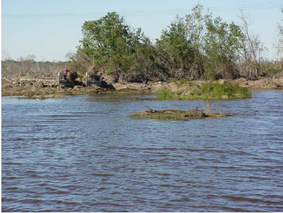
Photo # 9 Site 40 (view 1) Storm debris covers the entire structure and also completely blocked both culverts.
