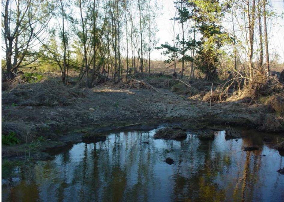
Photo # 19 Site 58 Selective erosion has progressed slightly in this 2005 inspection photo. The entire bank line is very badly eroded from the storm, and is covered with storm debris.
