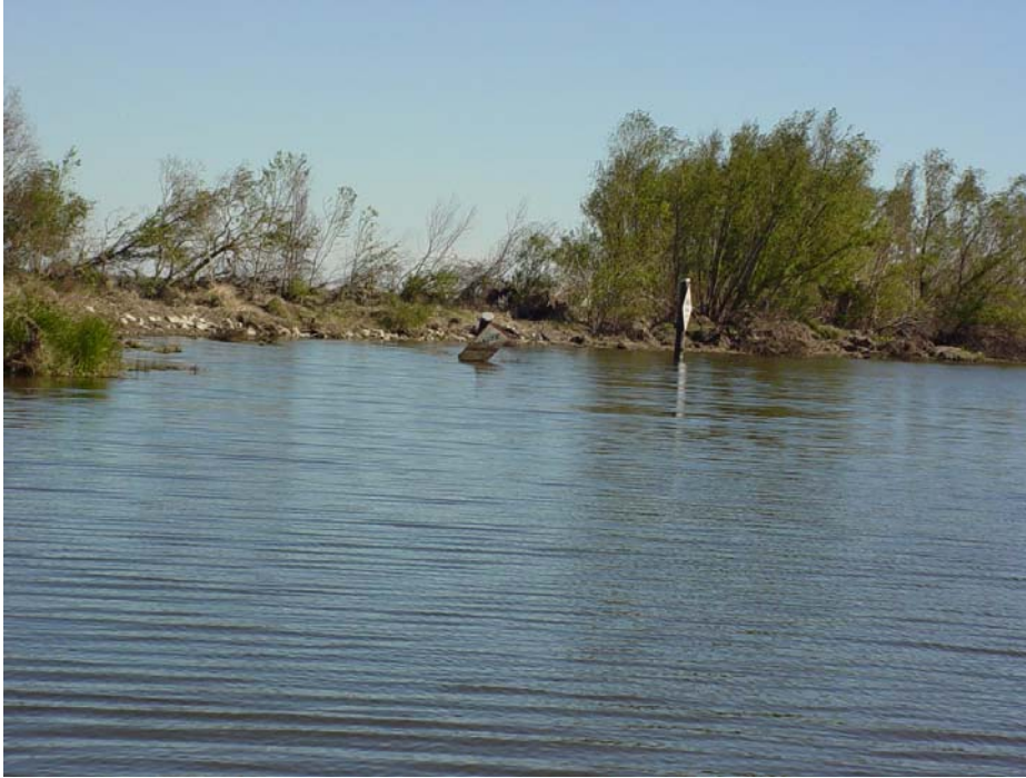
Photo # 17 Site 56 Overall condition of the canal rock closure appears to be good No appreciable subsidence has occurred since the 2005 inspection. The rock closure and the canal are completely covered with storm debris.
