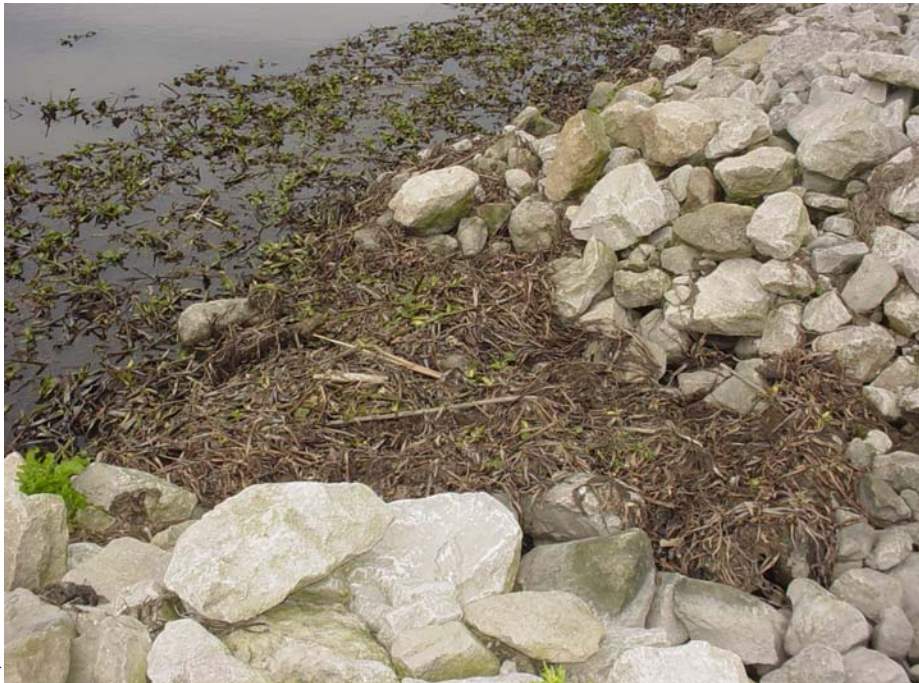
Photo # 8 Site 32 (view 2) This closer view shown that the removed rock was placed just adjacent to the opening.
