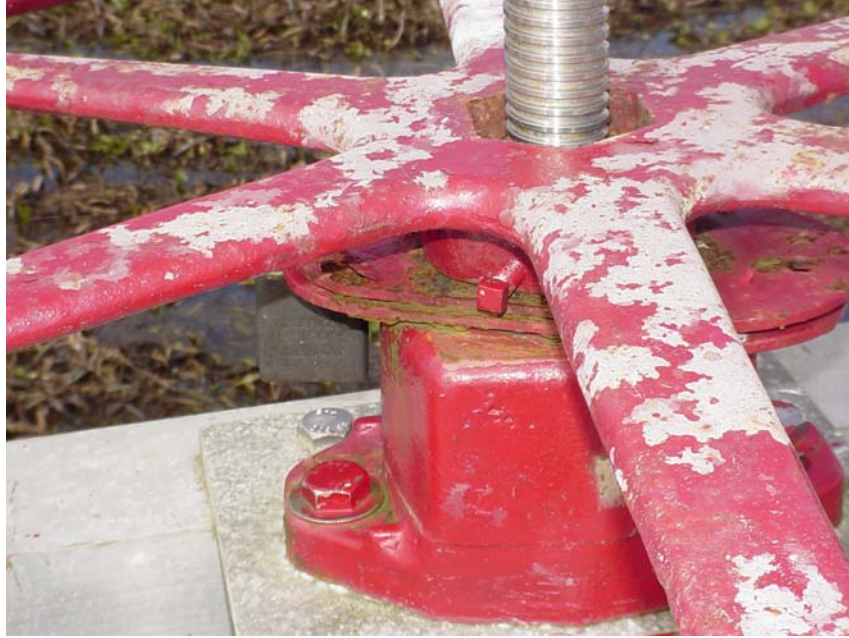
Photo # 1 Site 13 (view 1) Corrosion of locking plates caused them to separate making locking impossible.
