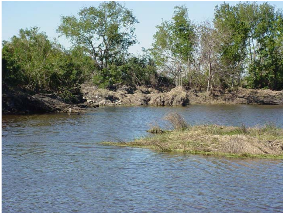
Photo # 18 Site 57 Embankment is covered with storm debris. It appears that it is also very badly eroded.
