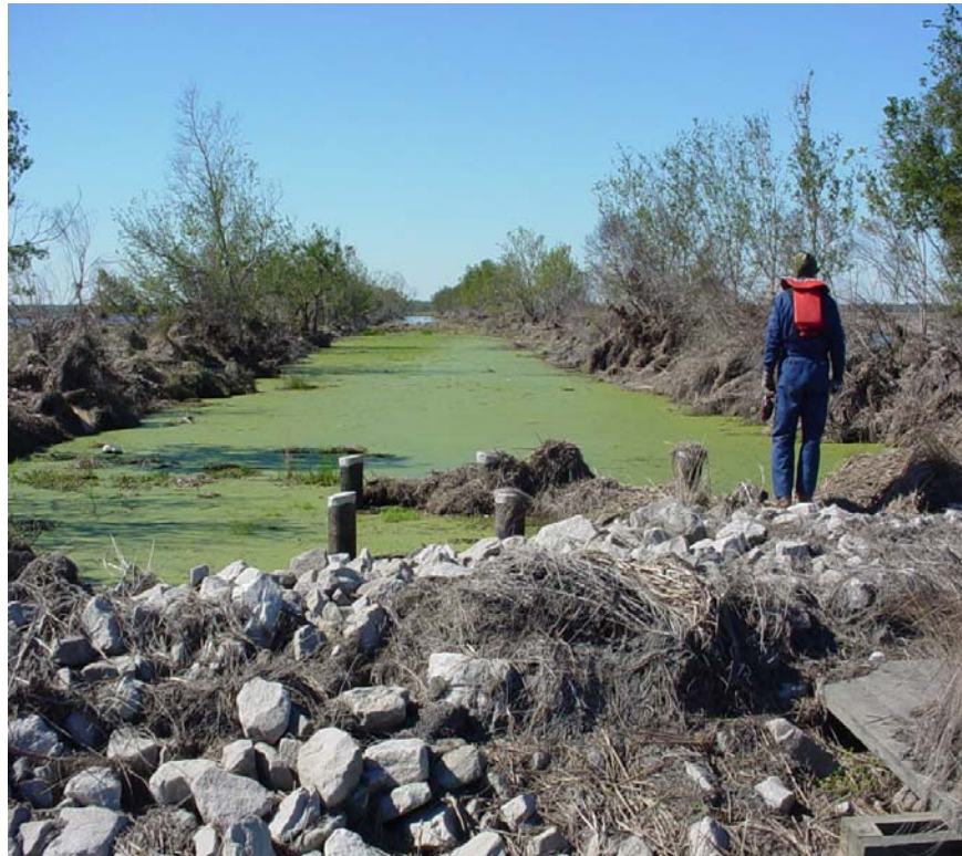
Photo # 15 Site 54 (view 1) Debris covers entire structure Culverts are also completely blocked.
