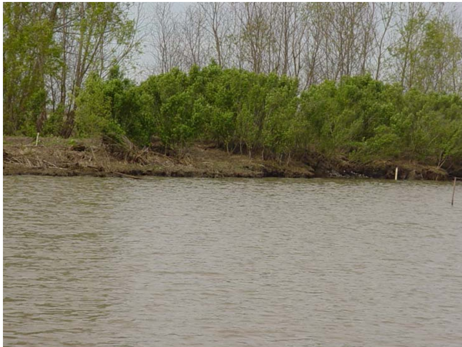
Photo # 20 Site 58 Selective erosion is in areas throughout snite; however, it is located in the slope and has not threatened the embankment crown.
