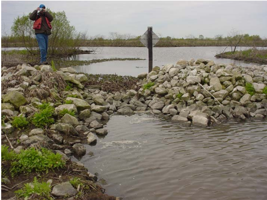
Photo # 7 Site 32 (view 1) This site was opened to the water line by vandals and was partially repaired by the 2003 inspection team. It was then vandalized again. This photo is from the 2005 inspection, debris now covers the structure.
