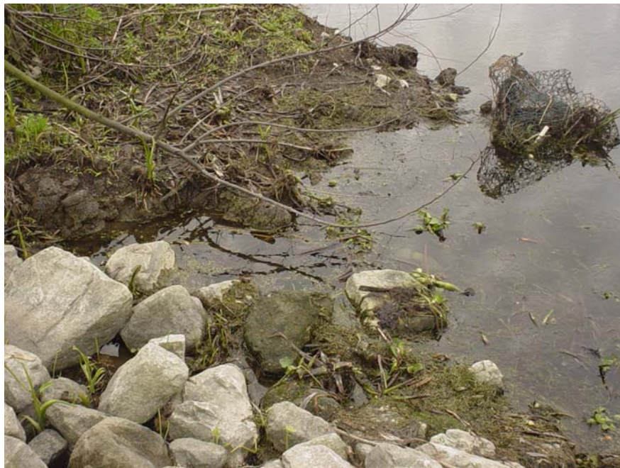
Photo # 14 Site 52 Slight erosion is evident in the areas where the rock closure ties into the earthen embankment in this 2005 inspection photo. Debris covers entire structure.
