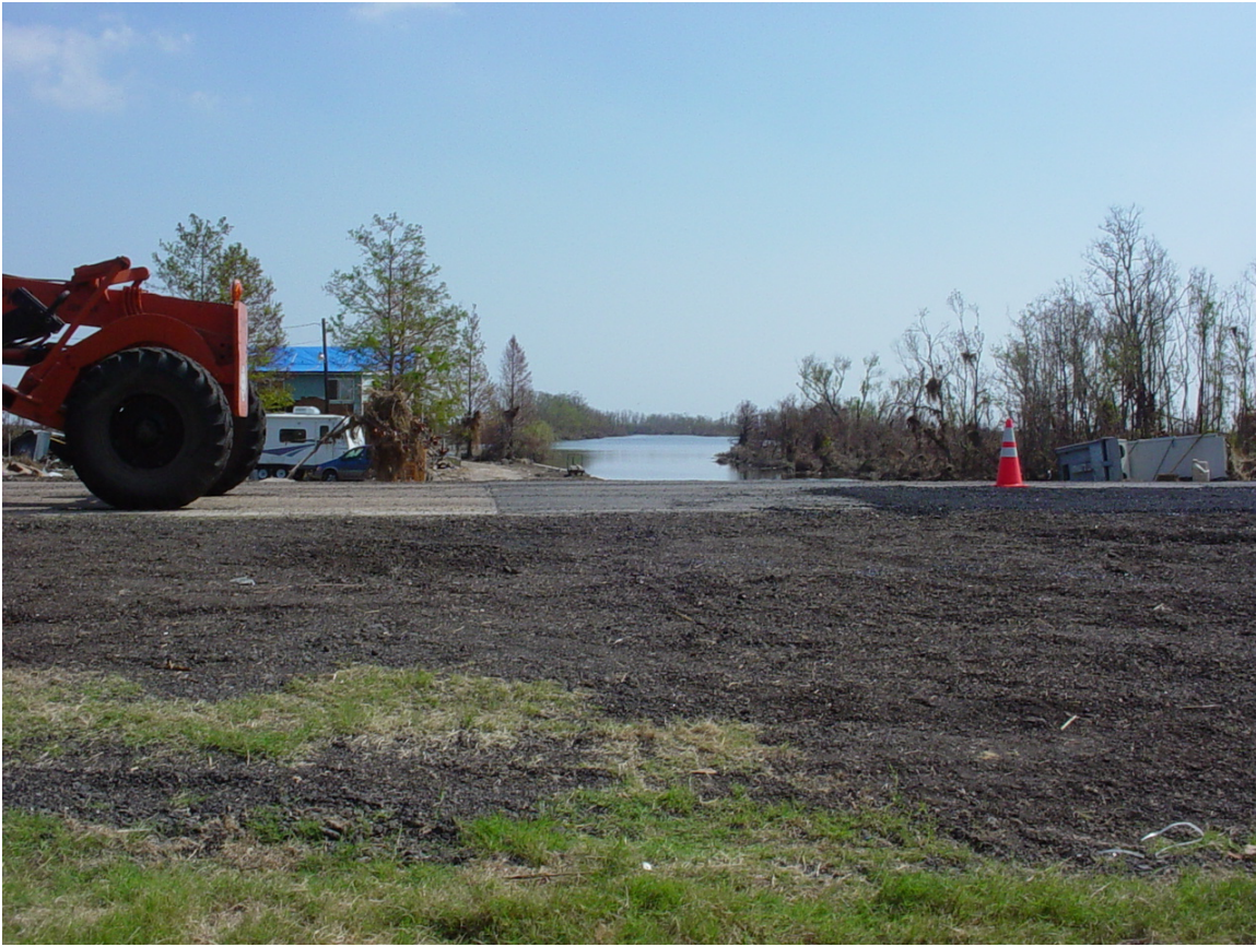
Photo #1 – Salt Bayou Culverts at Hwy 90. Looking East from inside the project area. Note the work being done to repair the damages to the road.
