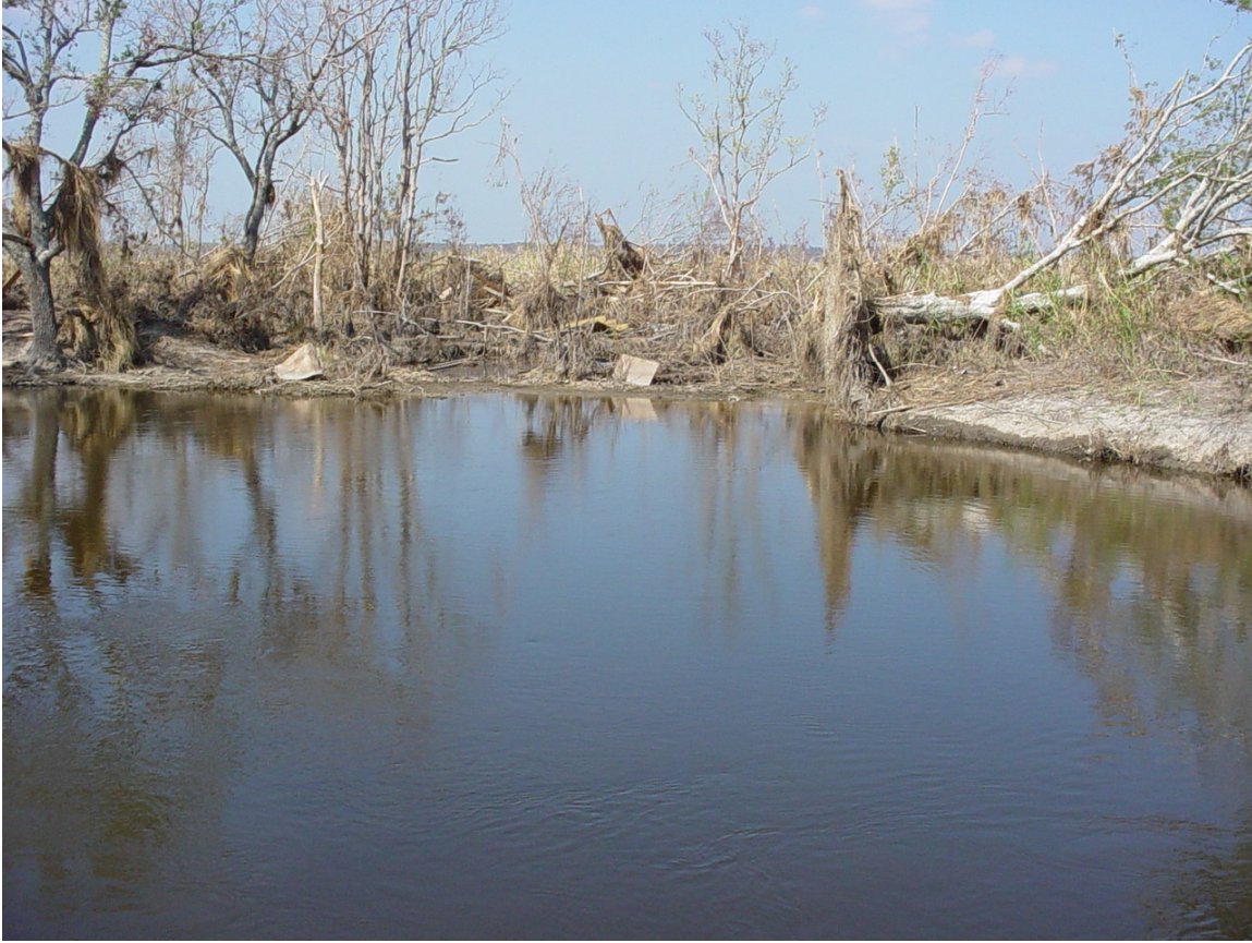
Photo #2 – Salt Bayou Scour. Looking at the north bank of Salt Bayou inside the project area from the Hwy 90 Culverts. Note the large section of bank which has been scoured out.
