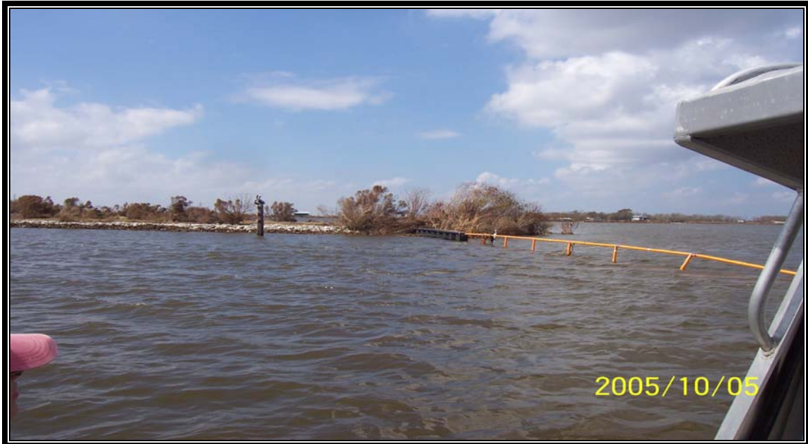
Structure #6 – photo of bent guard rail on the west side of barge bay.
