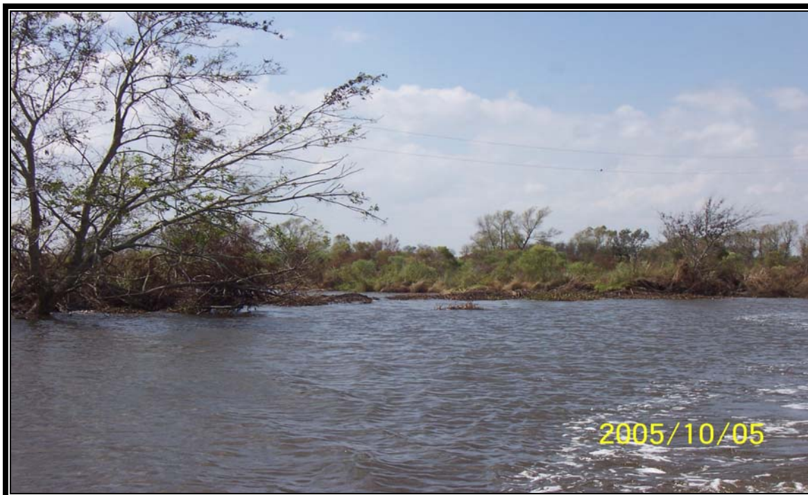
Photo of breach (approximately 20 ft. wide) located along east bank of Carencro Bayou.
