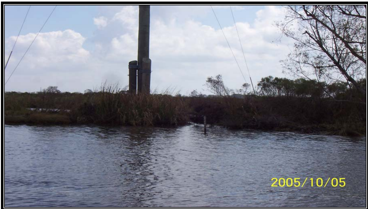
Photo of breach located along Carencro Bayou near electrical pole.
