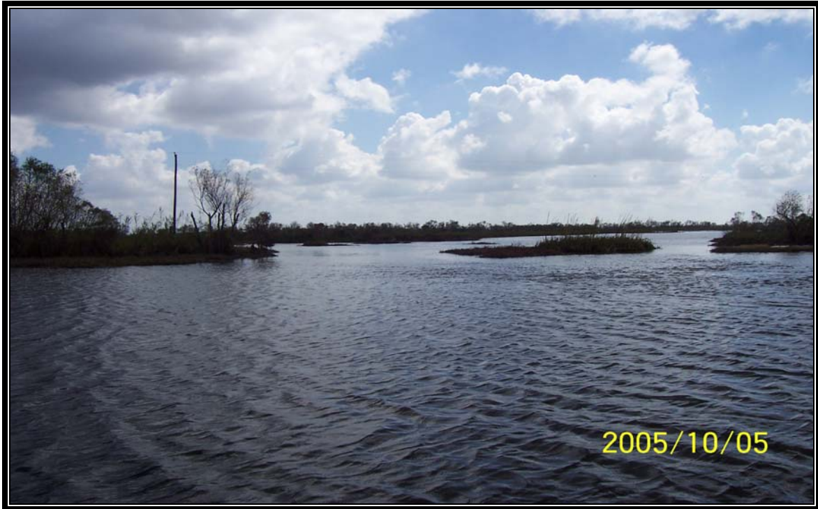
Photo of breach (approximately 80 ft wide) located along east bank of Little Carencro Bayou.
