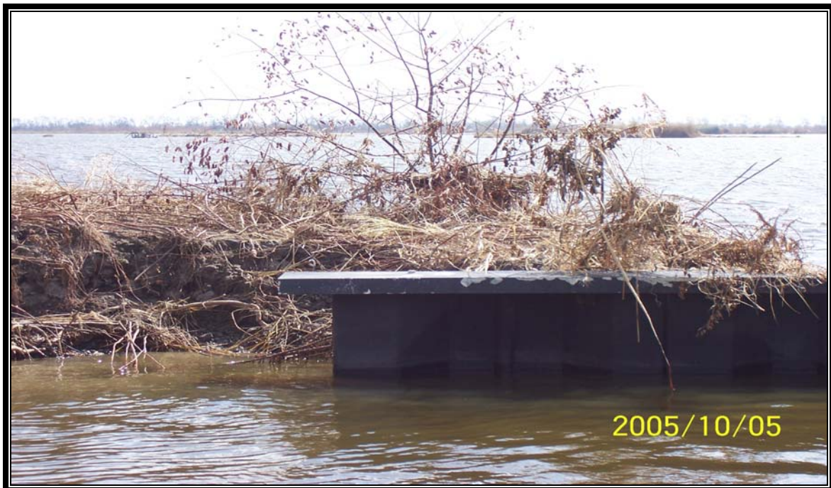
Structure #23 – significant erosion on the north side of the structure exposing the bulkhead.
