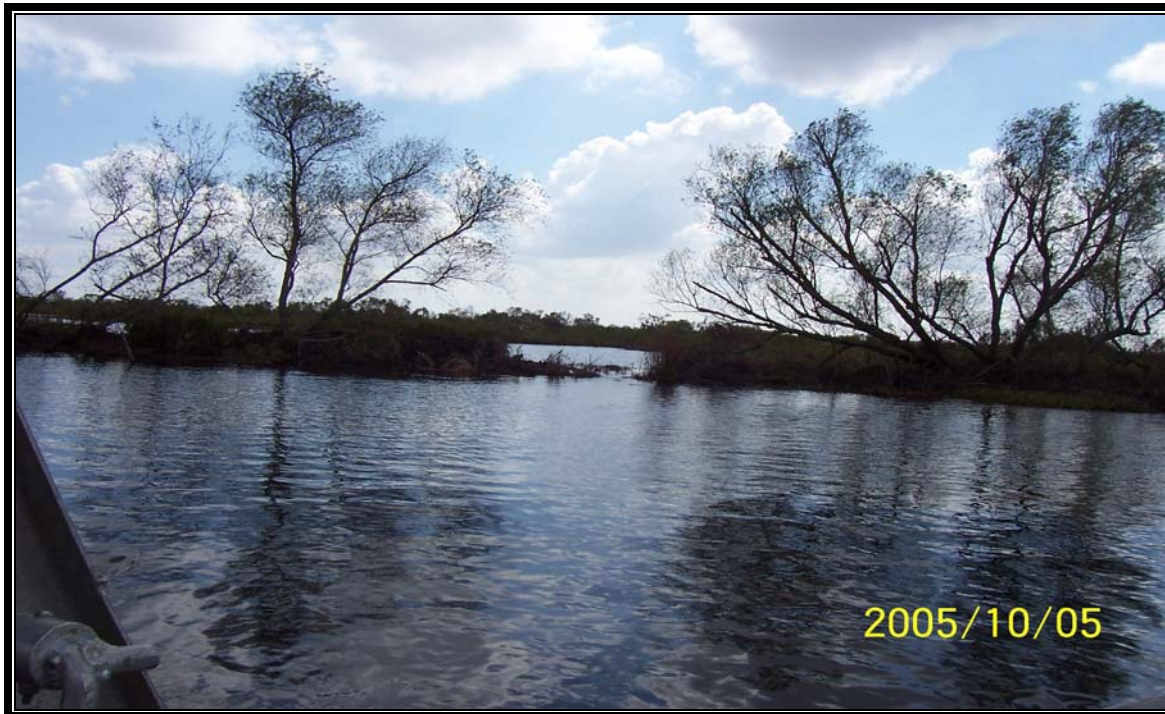
Photo of breach (approximately 25 ft wide) located along east bank of Little Carencro Bayou.
