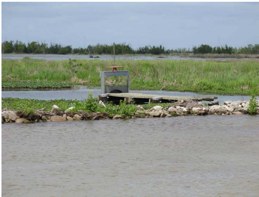
Photo # 2 Site 13 (view 2) The extent of blockage of the culvert due to storm debris is unknown. Note the high water stages, both in Bayou Mandeville and in the interior marsh.
