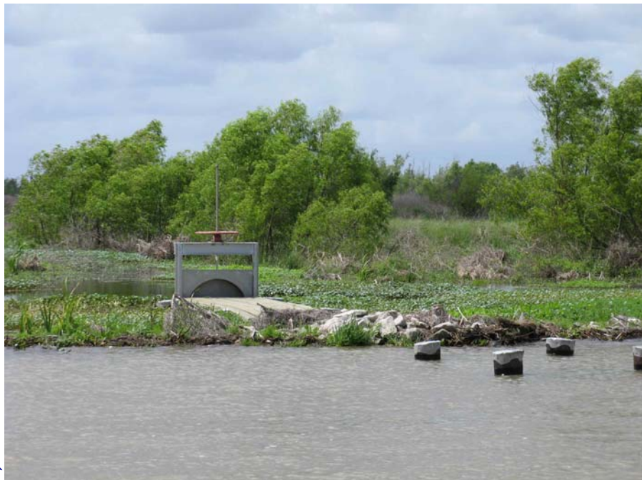
Photo # 8 Site 50 The extent of blockage of the culverts by storm debris is unknown. Slight erosion was evident on both sides of the rock plug where it ties into the earthen embankment. High flows such as this, allow water to flow around the structures to flood the marsh.
