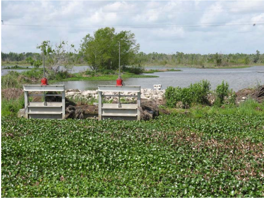
Photo # 7 Site 40 The structure remains covered with storm debris. The extent of blockage of the culverts by storm debris is unknown. The flowmeter was damaged but recovered. Note the high water stages from the structure westward to the Plaquemines east bank hurricane levee in the background.
