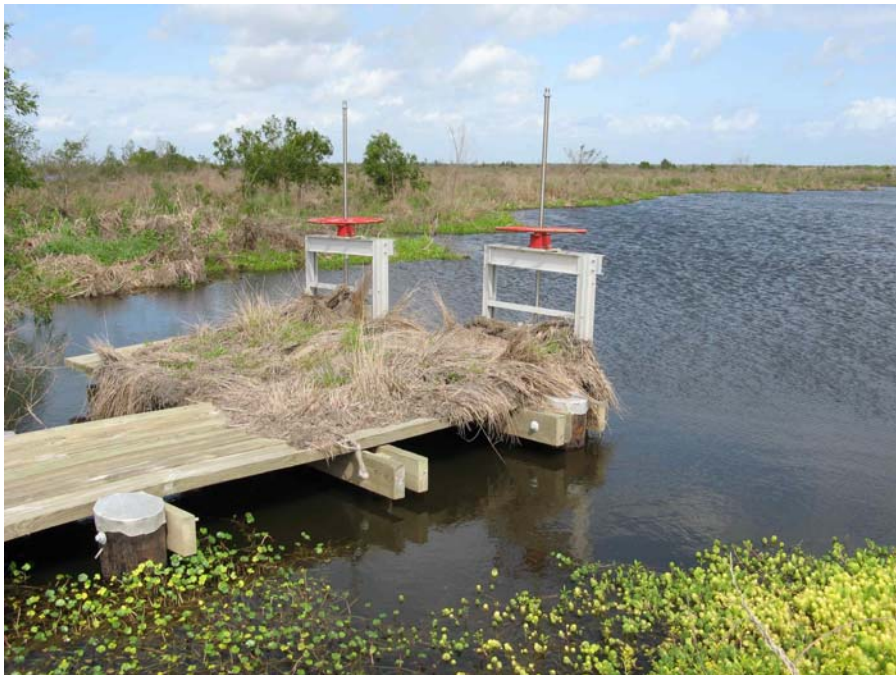
Photo # 20 Site 60 Storm debris remains on the structure. The extent of blockage of the culverts due to storm debris is unknown. Some flow was visible through the culverts.
