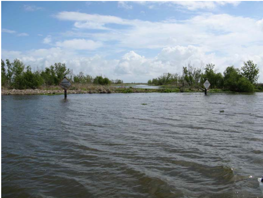
Photo #12 Site 56 The overall condition of the rock closure appears to be good. No appreciable subsidence has occurred since the post-storm inspection. Note the greater subsidence occurred at the center of the closure.
