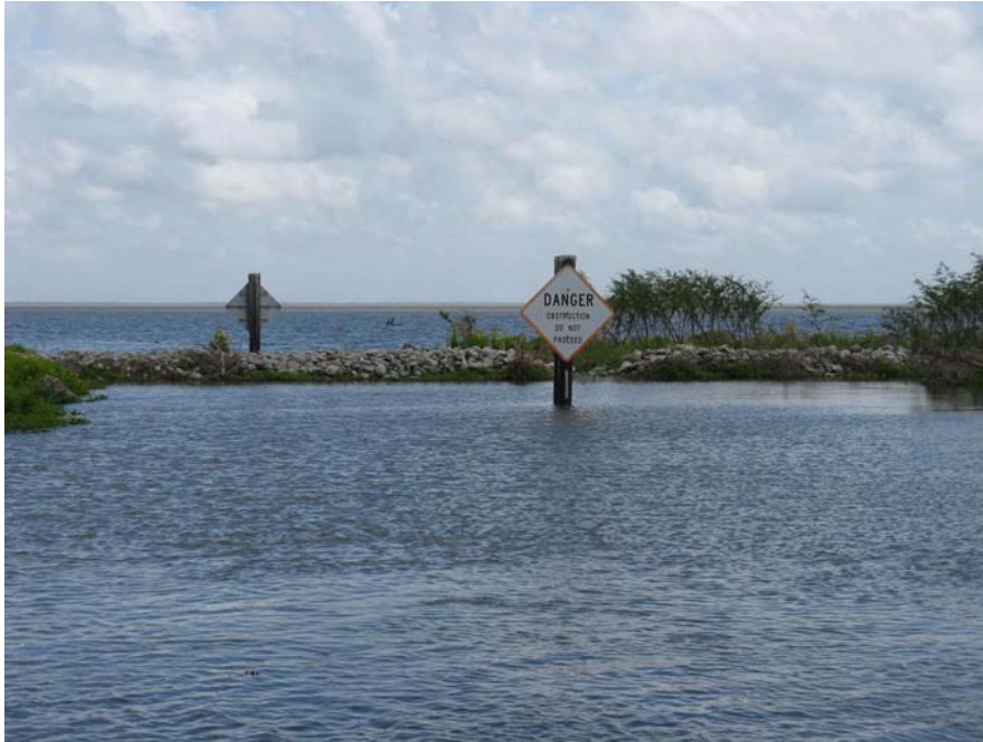
Photo # 5 Site 32 (view 1) This structure was opened to the waterline by vandals and was partially repaired by the 2003 inspection team. It was then vandalized again. Lake Leary is in background.
