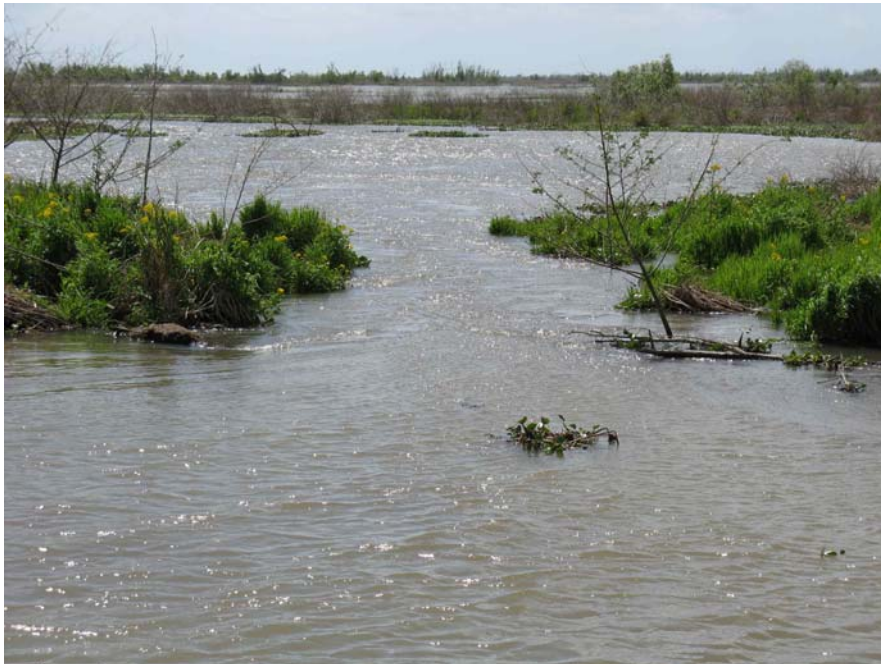
Photo # 10 Site 52 (view 2) This breach in the earthen embankment is approximately 100 yards to the west of the rock plug. Many of these breaches are evident throughout the outfall area allowing free flowage from the conveyance channels into the interior marshes.
