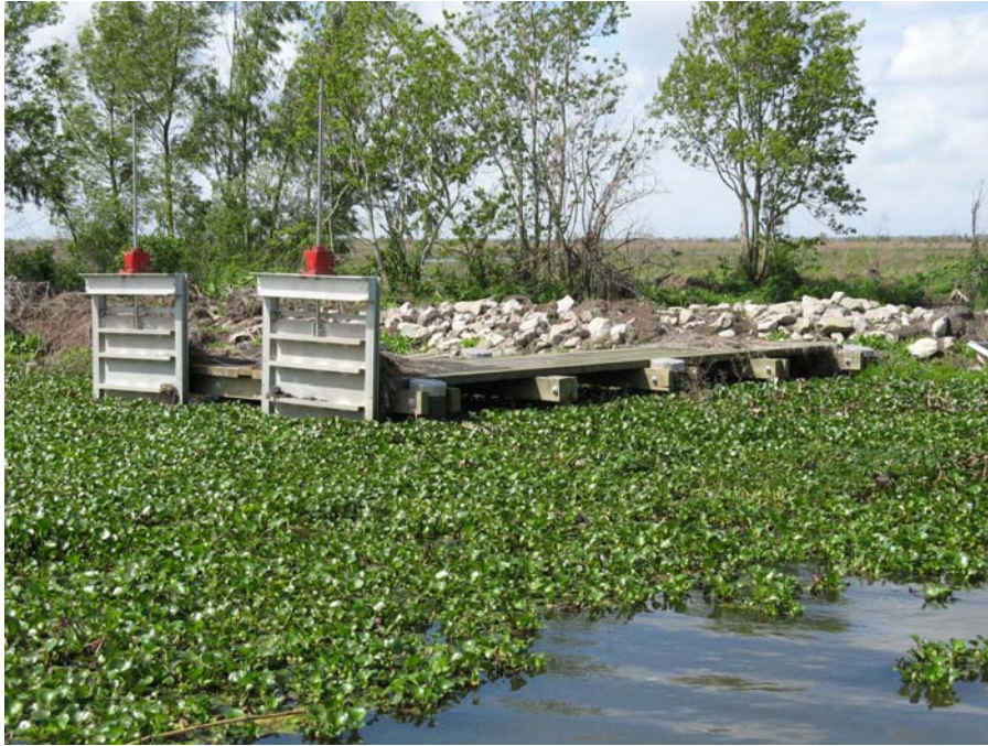
Photo # 11 Site 54 Some storm debris remains. The extent of blockage of the culverts by storm debris is unknown. The flowmeter and all attachments on this structure were destroyed by the storm.
