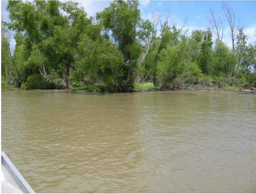
Photo # 17 Site 58 (view 1) Bayou Mandeville spoil bank. Many damaged trees along the bank line are being removed by the landowner.
