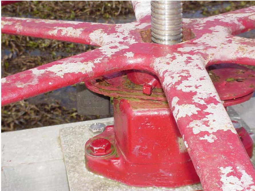
Photo # 1 Site 13 (view 1) Corrosion of locking plates caused them to separate making locking impossible. (Photo from 2005 inspection)
