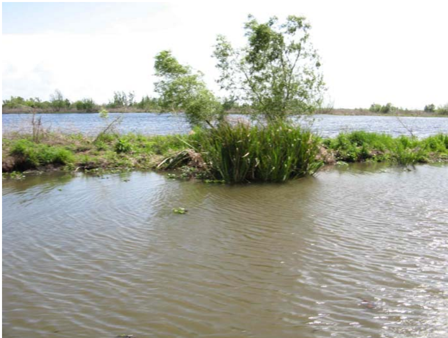
Photo # 14 Site 57 (view 2) Reggio Canal spoil bank. More recovering vegetation. Water levels in the marsh and the conveyance channel remains equal due to amount of damage to the spoil banks.
