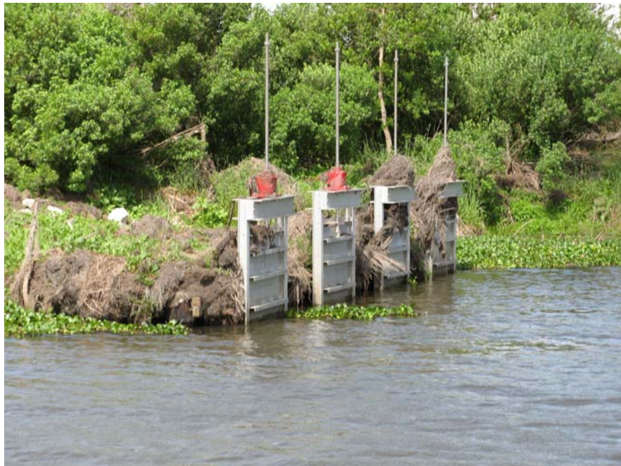
Photo #4 Site 26 The structure remains covered with storm debris. The extent of blockage of the culverts by storm debris is unknown. The flowmeter and all attachments were destroyed by the storm.
