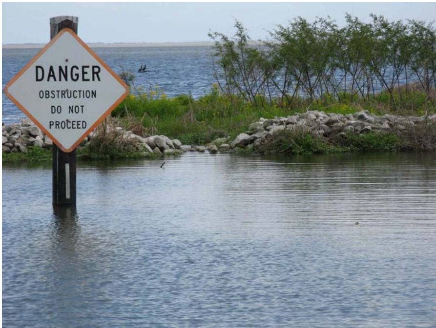
Photo # 6 Site 32 (view 2) Close up view of the vandalized area. Approximately 30% of the west lake rim was destroyed by the storms.
