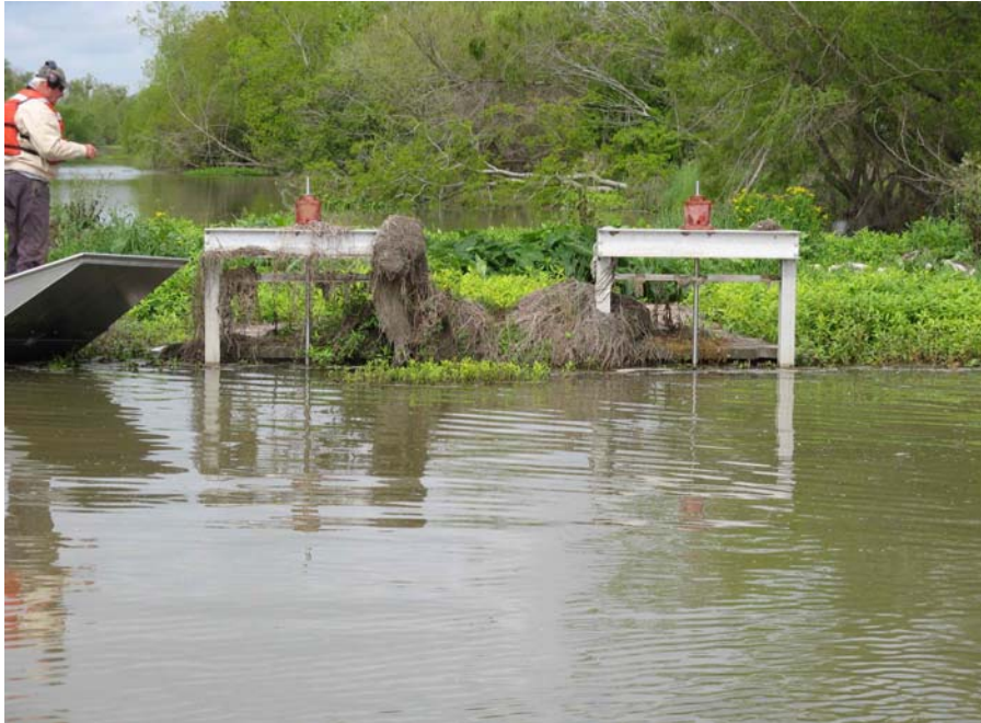
Photo # 3 Site 25 The structure remains covered with storm debris. Both of the gates remained closed to reduce flow to the Braithwaite area where the USACE is constructing an emergency levee contract.
