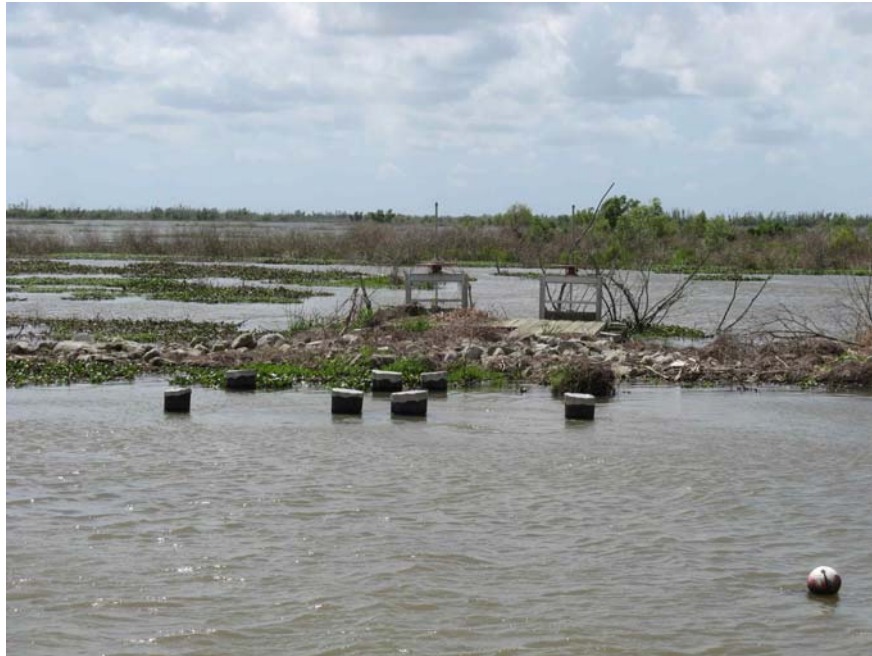
Photo # 9 Site 52 (view 1) Some storm debris remains. The extent of blockage of the culverts by storm debris is unknown. Slight erosion was evident on both sides of the rock plug where it ties into the earthen embankment.
