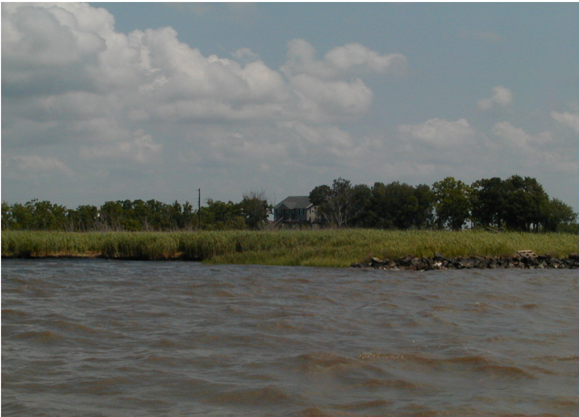
Photo 4 —south west tie-in of rock dike
