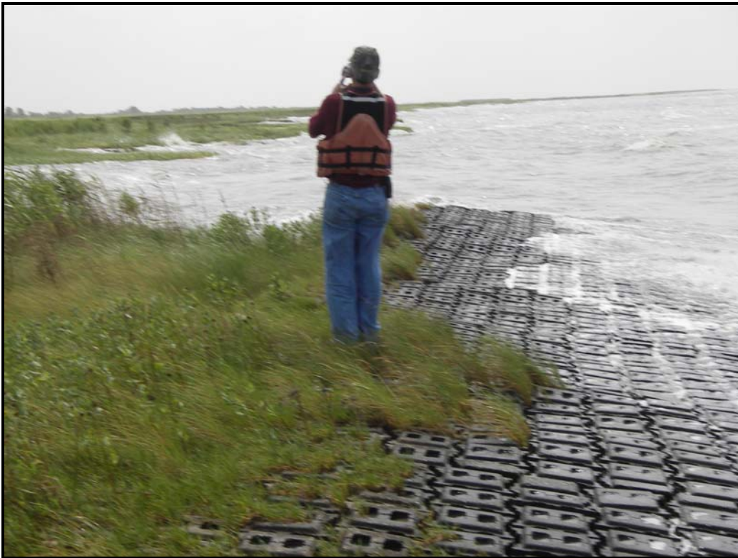
Photo 4, Area 2, East side of concrete mats. (June 19, 2007)
