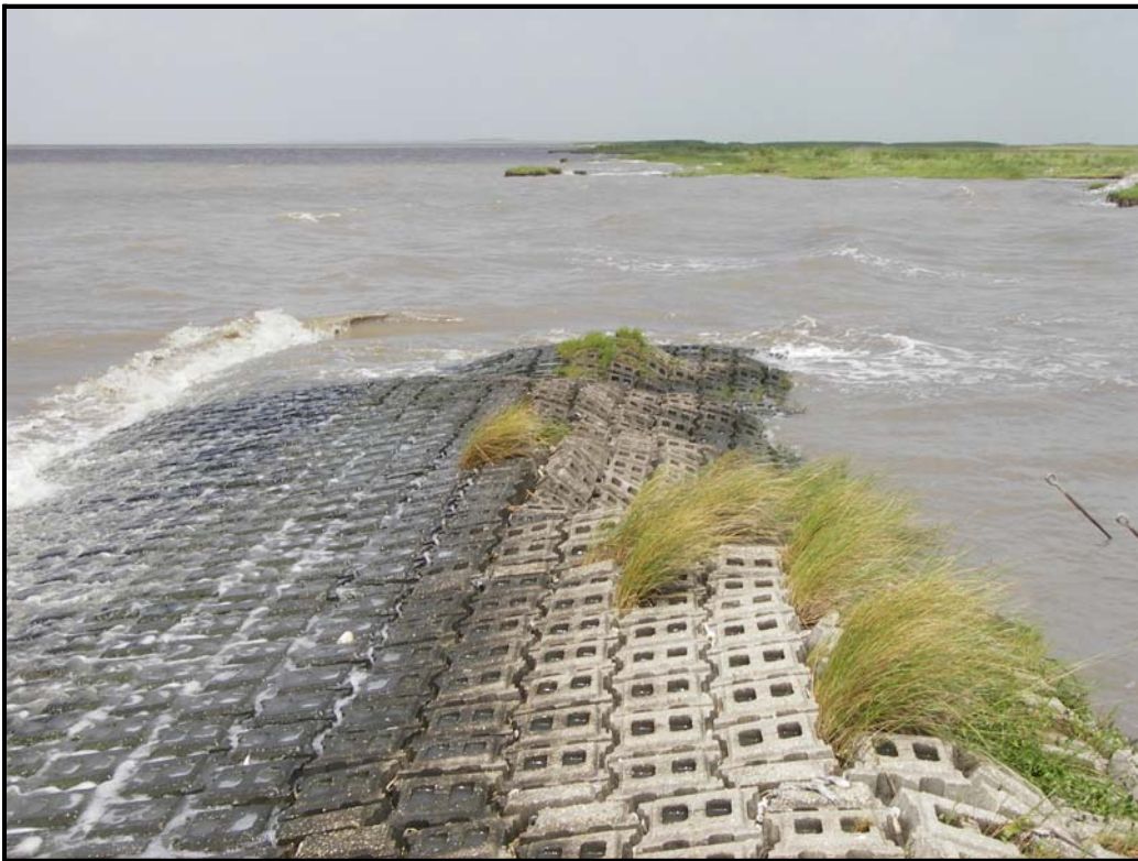
Photo 2, Area 2, West side of concrete mats. (June 19, 2007)
