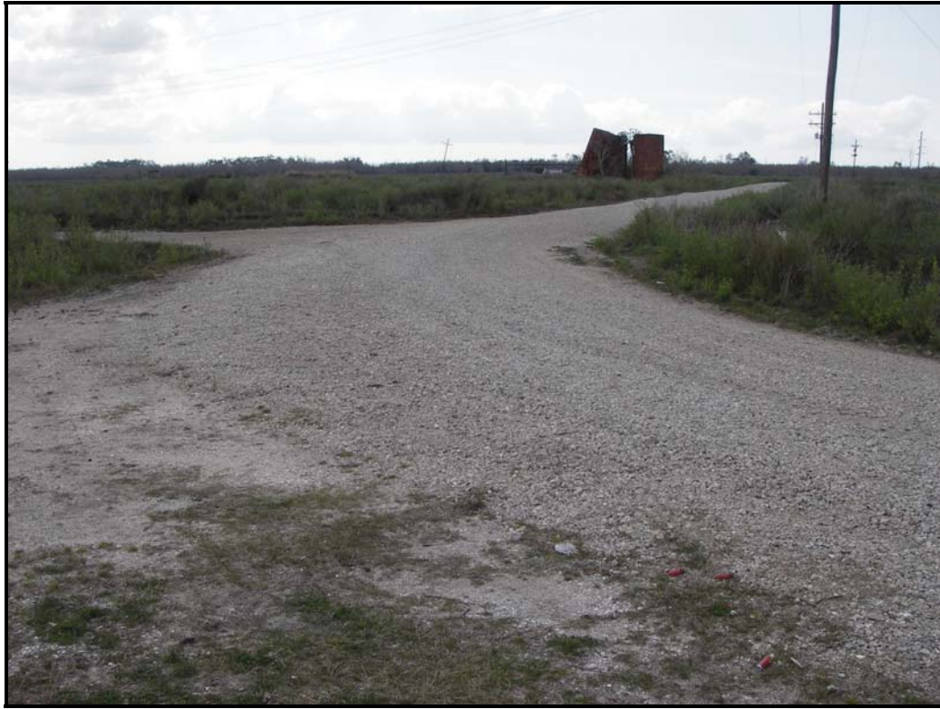
Photo 5. Access roadway to Structure No.1, recently repaired with recycled concrete. (March 8, 2007)
