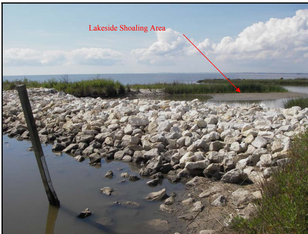
Photo 10. Rock plug at Structure No. 8. (March 8, 2007)
