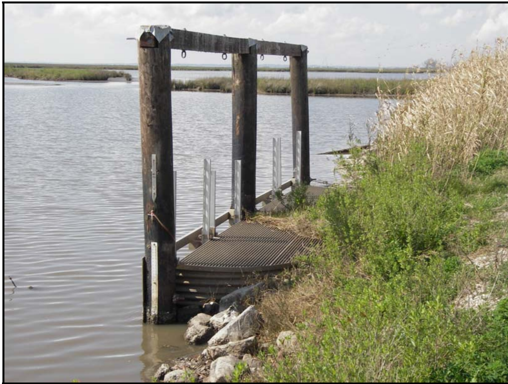
Photo 6. Inlet side of Structure No. 12. (March 8, 2007)
