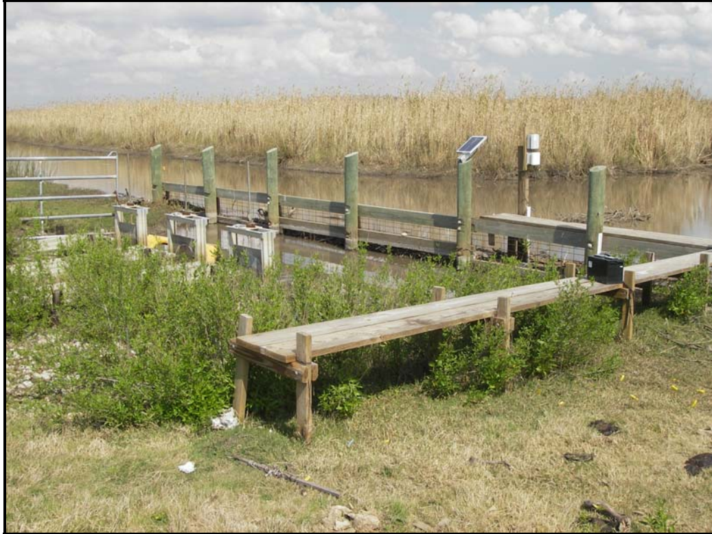
Photo 1. View showing hyacinth fence and sluice gates at Structure No. 1. (March 8, 2007)
