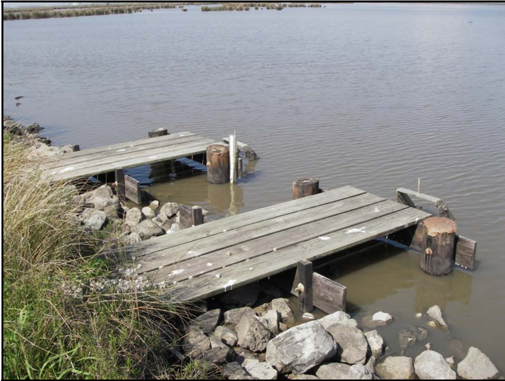
Photo 7. Outlet pipes for Structure No. 12. (March 8, 2007)
