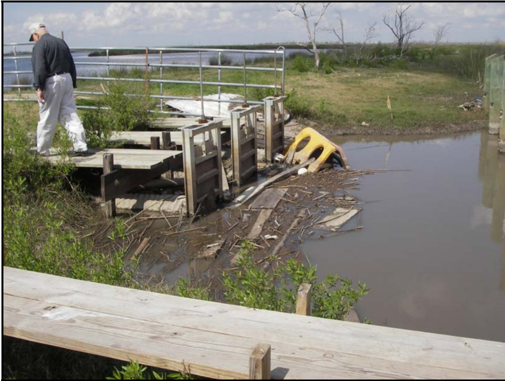
Photo 3. View showing trash and debris within hyacinth fence that needs to be removed. (March 8, 2007)
