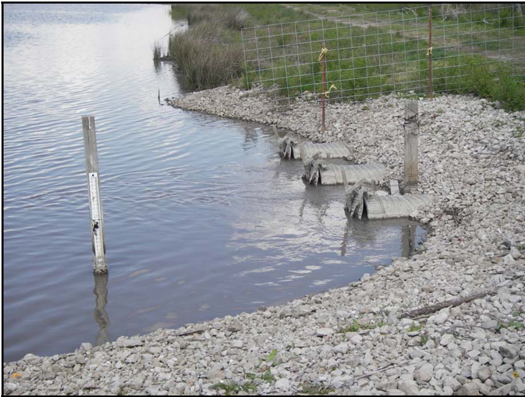
Photo 4. Outlet side of Structure No. 1. (March 8, 2007)
