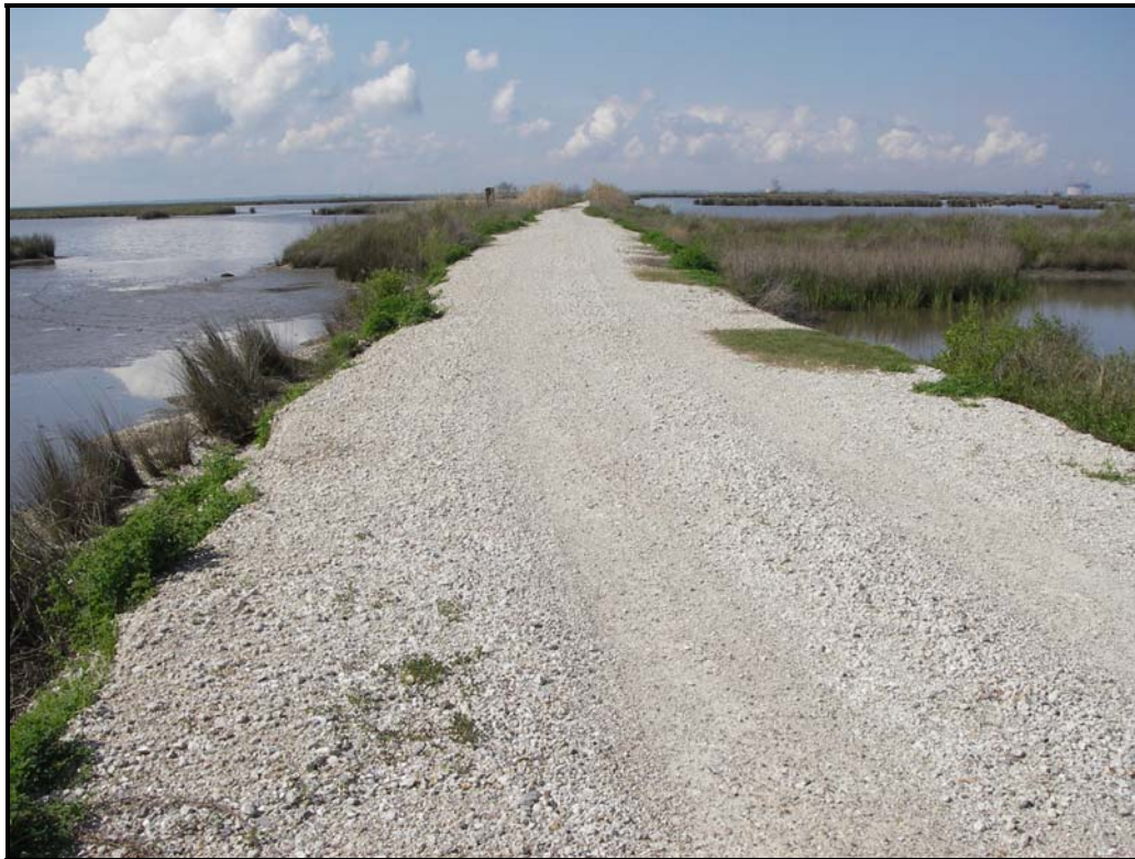
Photo 9. Access roadway to Structure No. 12, recently repaired with recycled concrete. (March 8, 2007)
