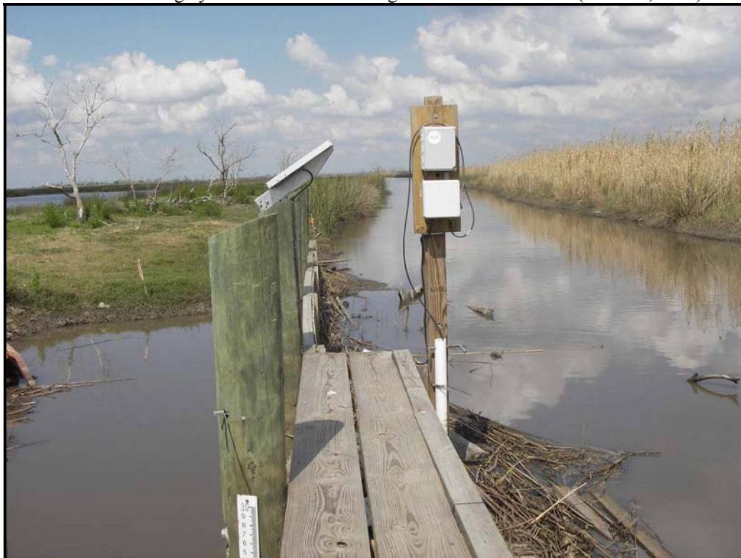
Photo 2. View showing Portable Multi-Parameter Water Quality Troll 9500 (29r) with wooden boardwalk at Structure No. 1. (March 8, 2007)
