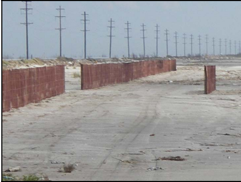
Photo 4, Start of new fence installation, east end of project. (10-30-2006)
