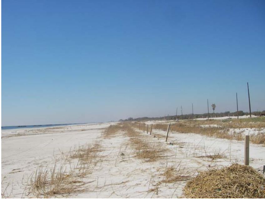
Figure 7c. View of a section of the sand fencing and vegetation plantings taken October 2005. The photograph is facing west.
