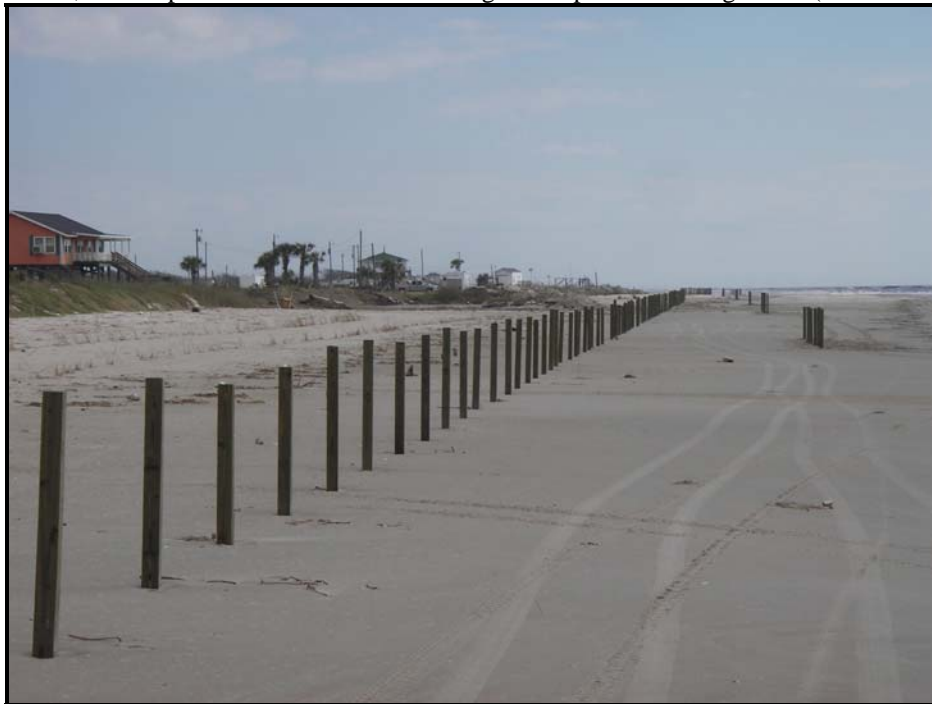
Photo 3, View of fence posts installed along primary fence alignment. (10-30-2006)
