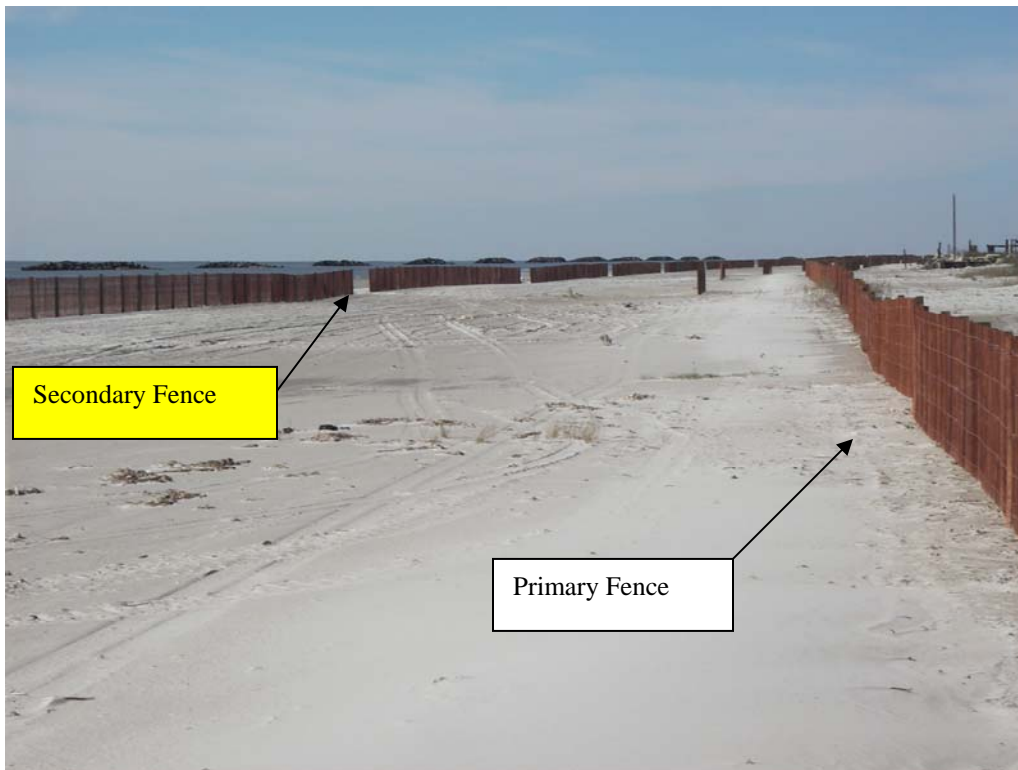
Photo 5, View of primary and secondary fence alignments, looking west. (12-1-2006)
