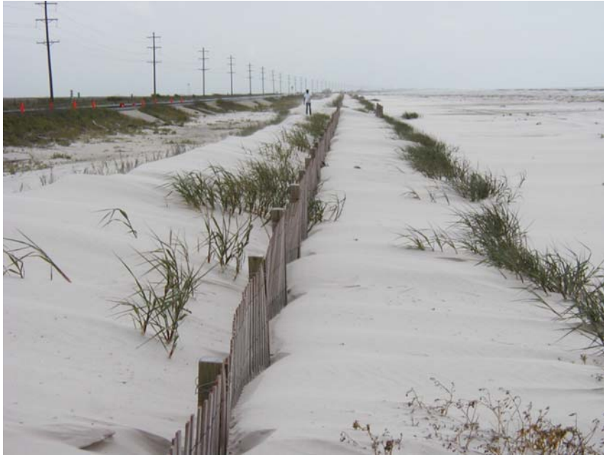
Figure 7a. View of the sand fencing and vegetation plantings at Station CS31-108 taken in April 2004. Note the dune formation almost covering the fences. The photograph is facing east.
