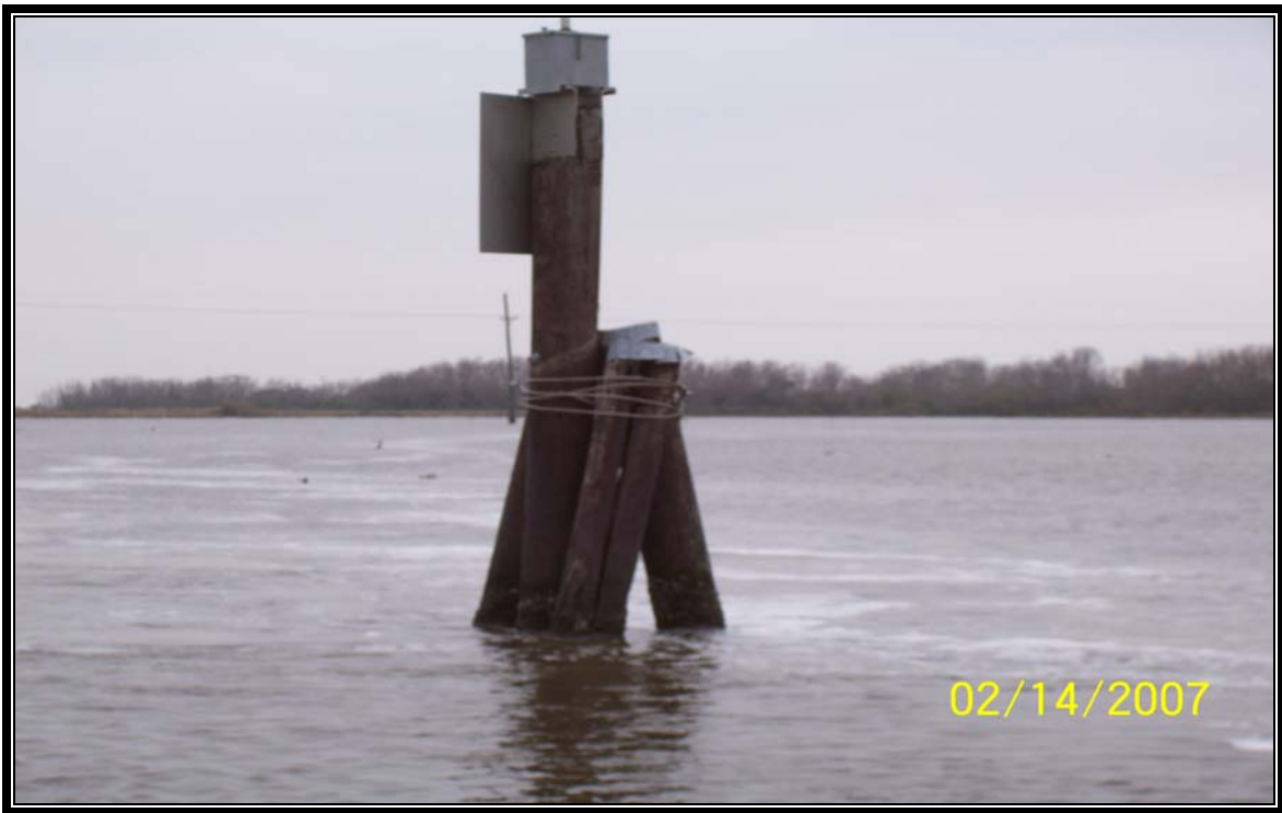
Photo 5 – (Structure 6) – damaged timber pile cluster on the southwest side of structure 6.
