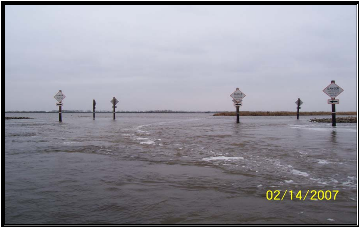
Photo 9 – (Structure 10) – rock lined channel located along Voss Canal.
