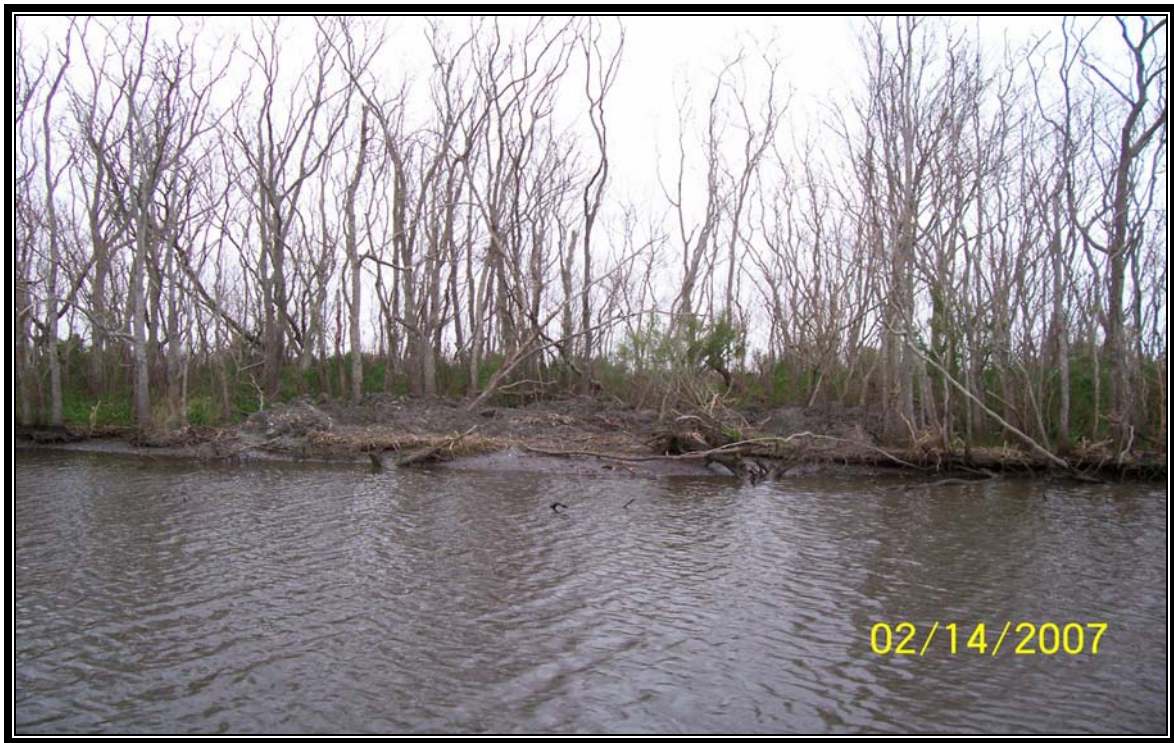
Photo 21 – Breach repair located along Breach 7 completed in 2006 by Apache Corporation.
