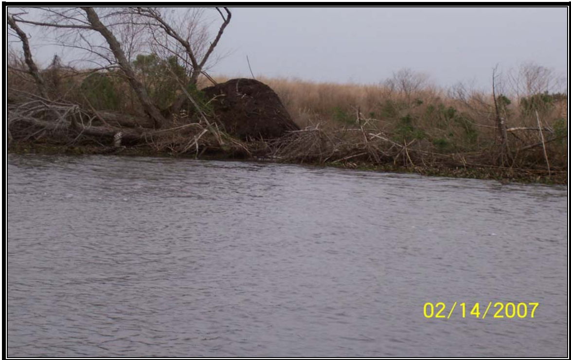
Photo 36 – Newly discovered breach along Carencro Bayou uprooted tree.
