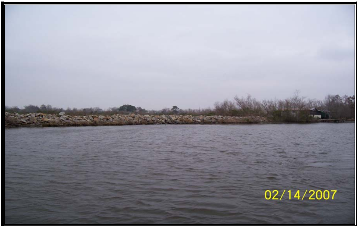
Photo 20 – (Breach Repair 7) – rock dike along location canal off of Superior Canal completed in 2003.
