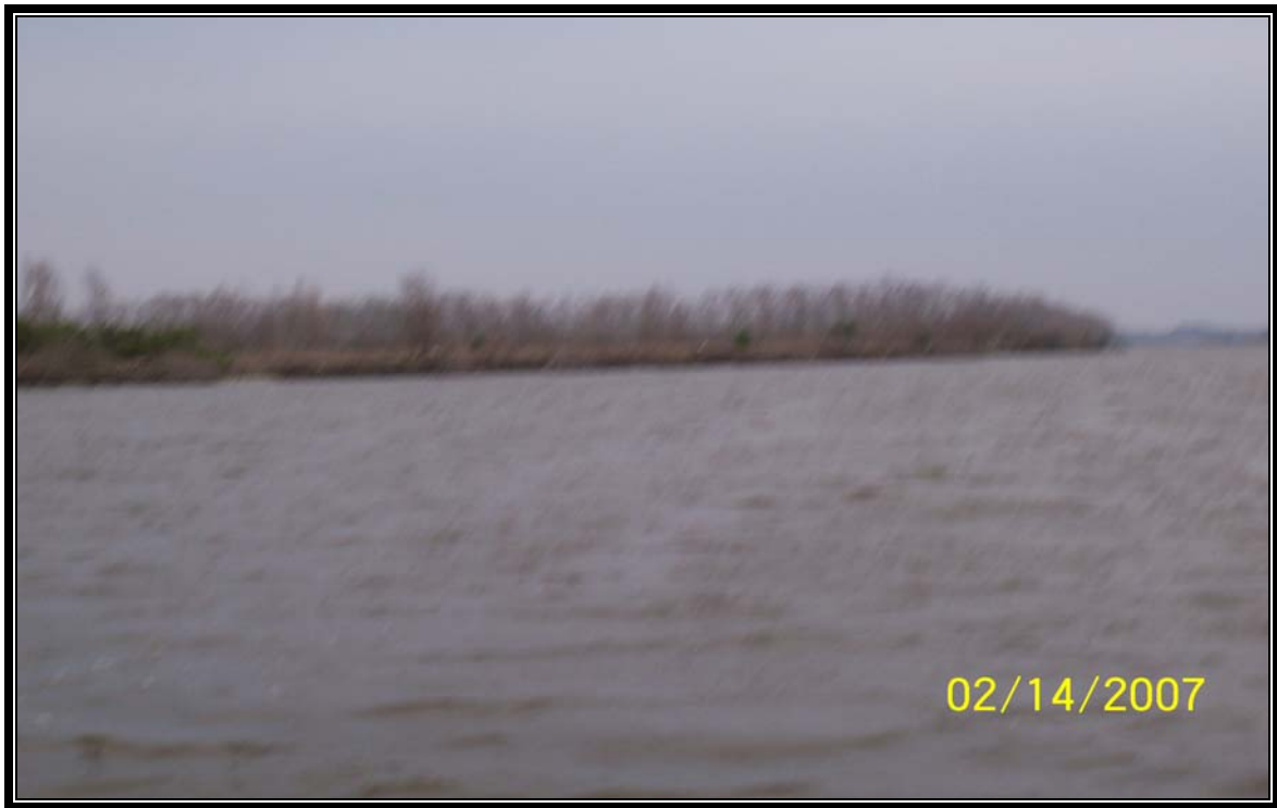
Photo 19 – (Breach Repair 5 and 6) – Levee refurbishment along Turtle Bayou completed in 2003.
