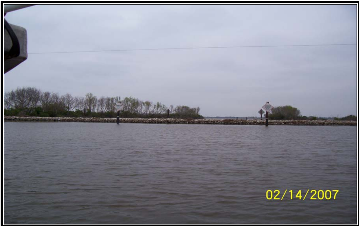
Photo 6 – (Structure 7) – rock channel plug located along the north bank of Bayou Decade.
