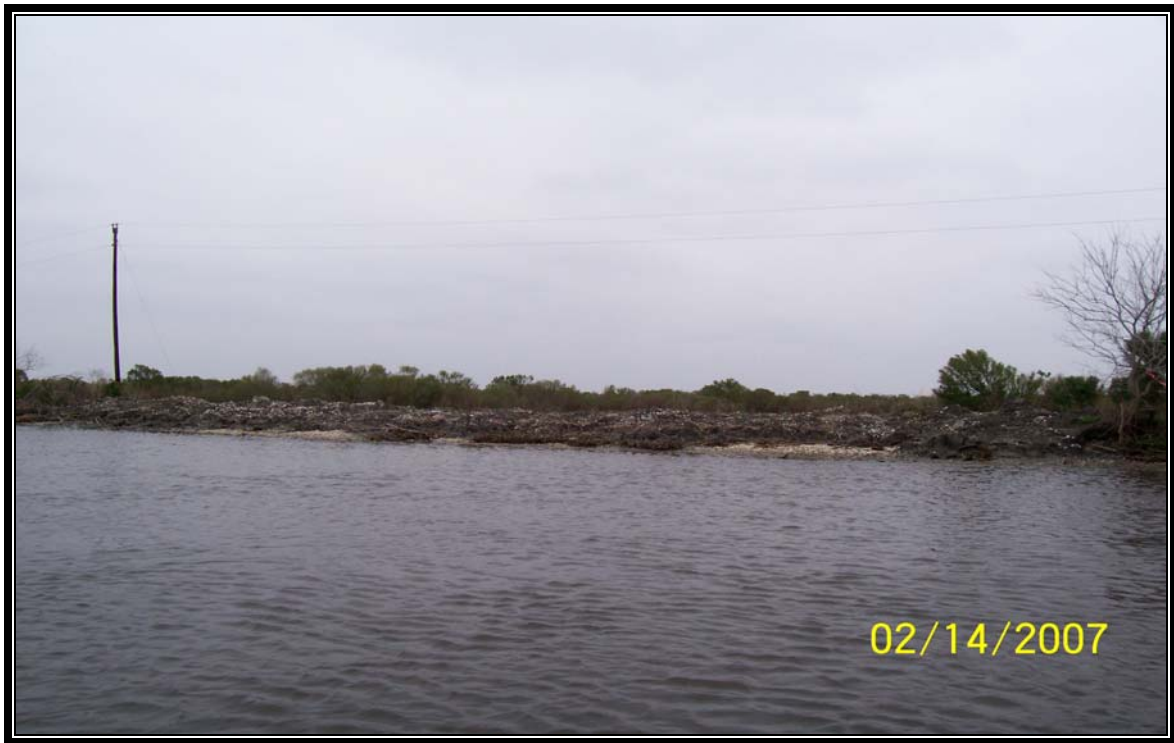
Photo 27 – Breach repair completed in 2006 by Apache Corporation along Carencro Bayou.
