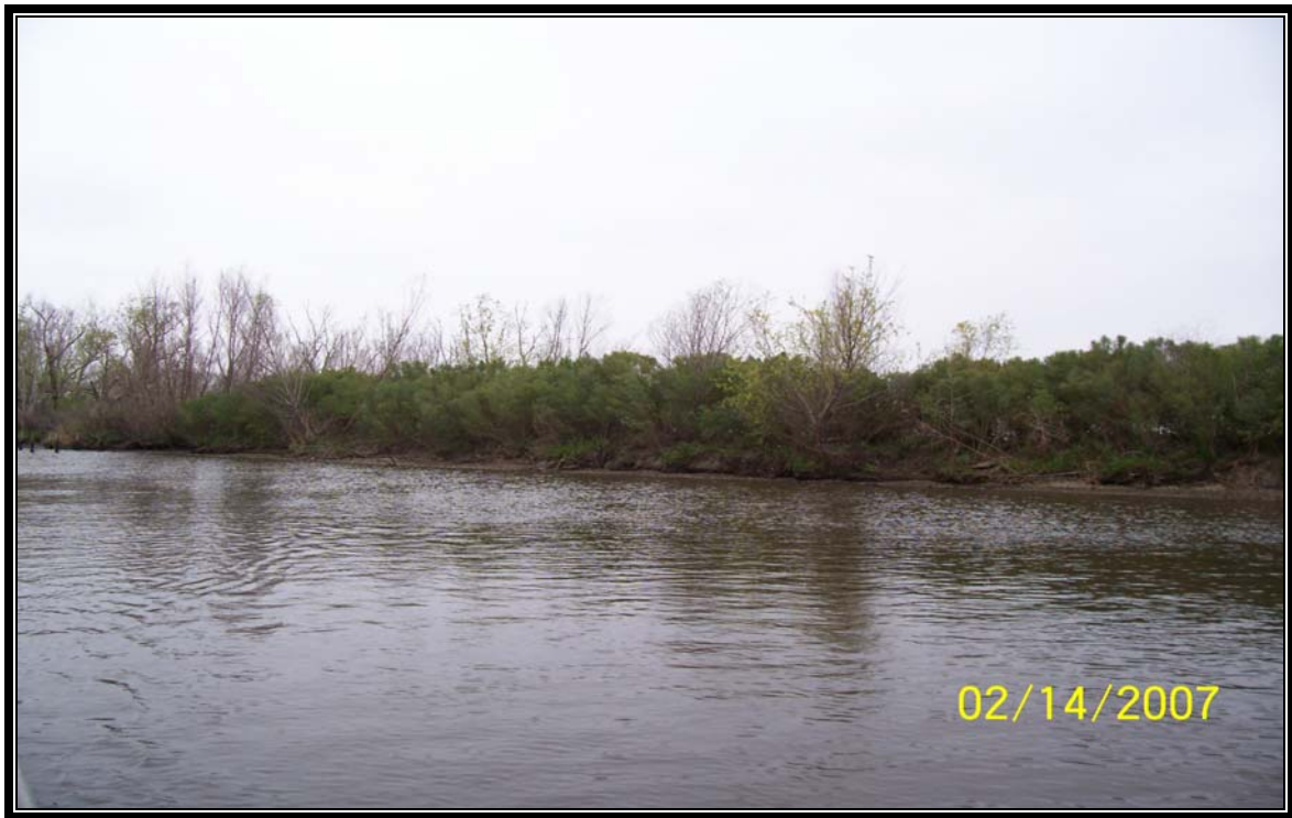
Photo 23 - (Breach Repair 9) – levee refurbishment along Superior Canal completed in 2003.
