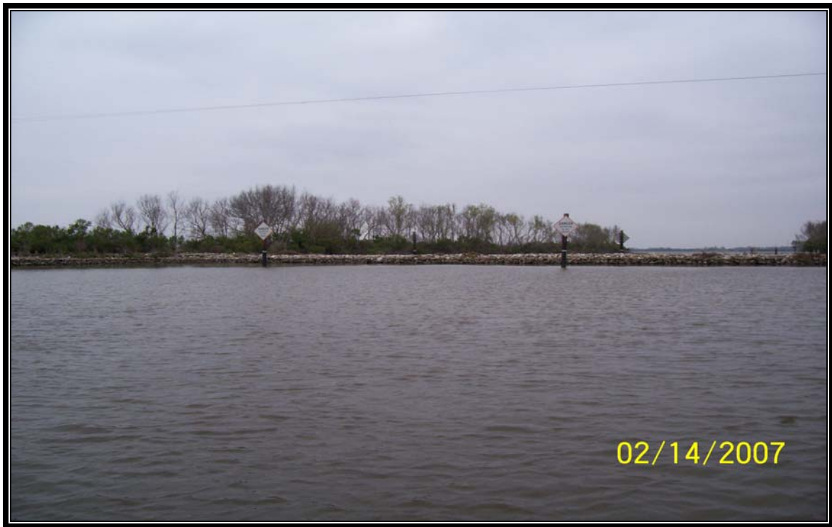
Photo 7 – (Structure 7) – rock channel plug located on the north bank of Bayou Decade.
