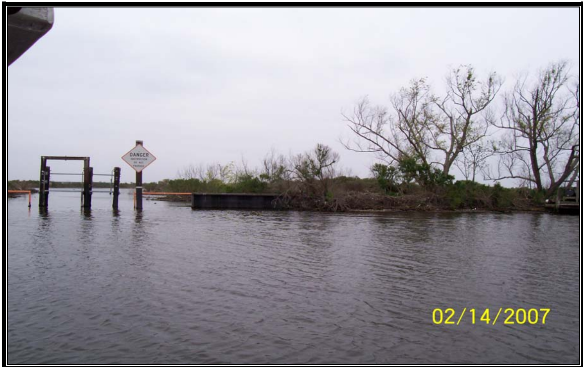
Photo 10 – (Structure 14) – southern tie-in of variable crest weir structure along Carencro Bayou.
