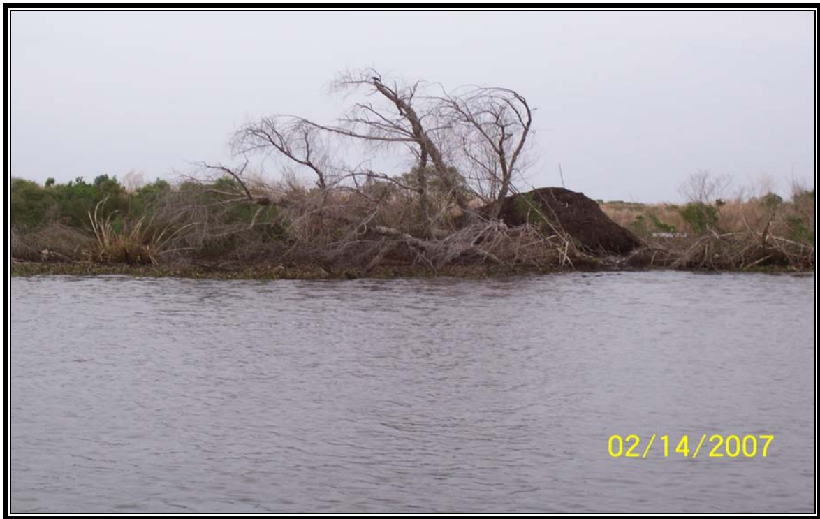
Photo 35 – Newly discovered breach along Carencro Bayou caused by uprooted tree.
