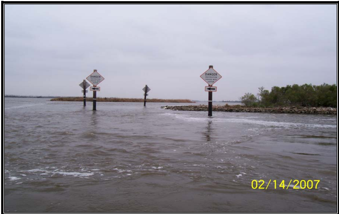
Photo 8 – (Structure 10) – south bank of rock lined channel along Voss Canal.
