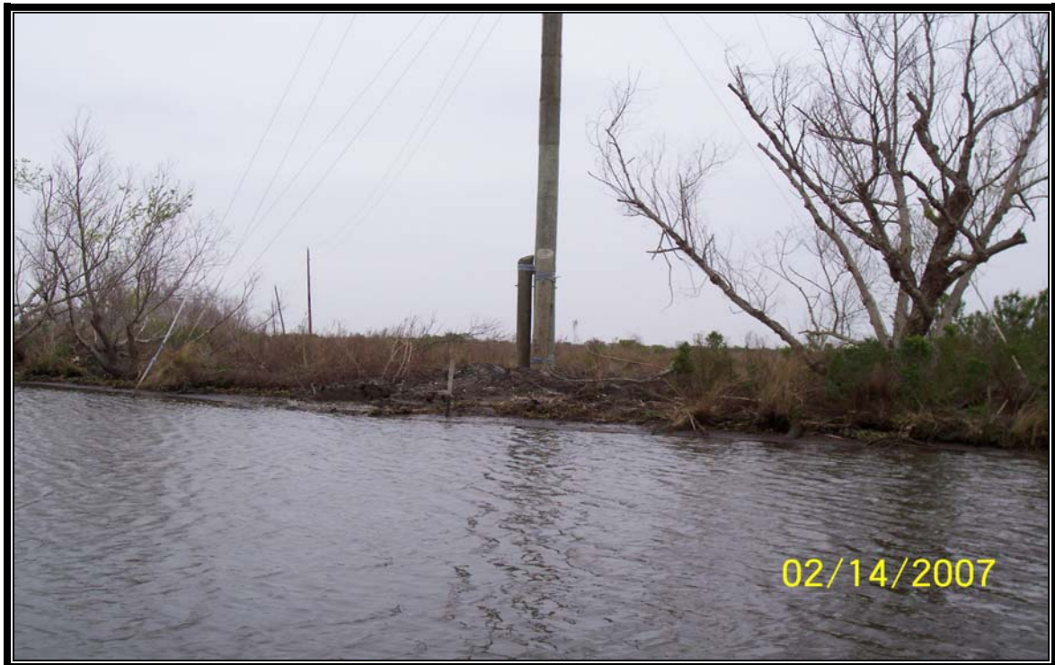
Photo 26 – Breach repair located along Carencro Bayou adjacent to power lines near camp sites.
