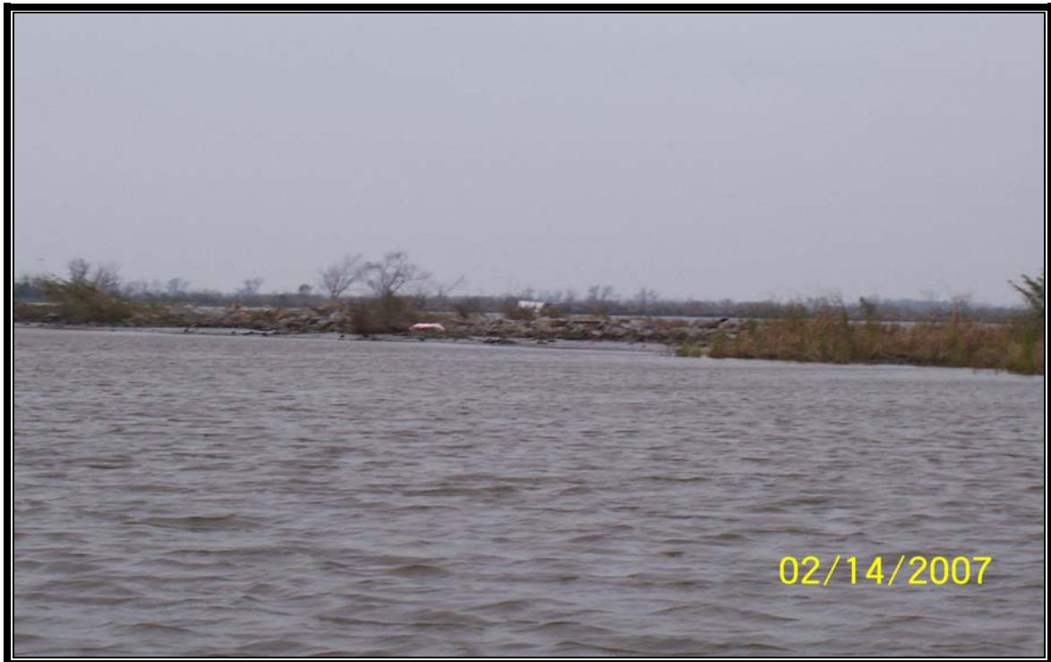
Photo 16 – (Breach Repair 1 through 4) - rock dike constructed in 2003 to close large openings in the bank.
