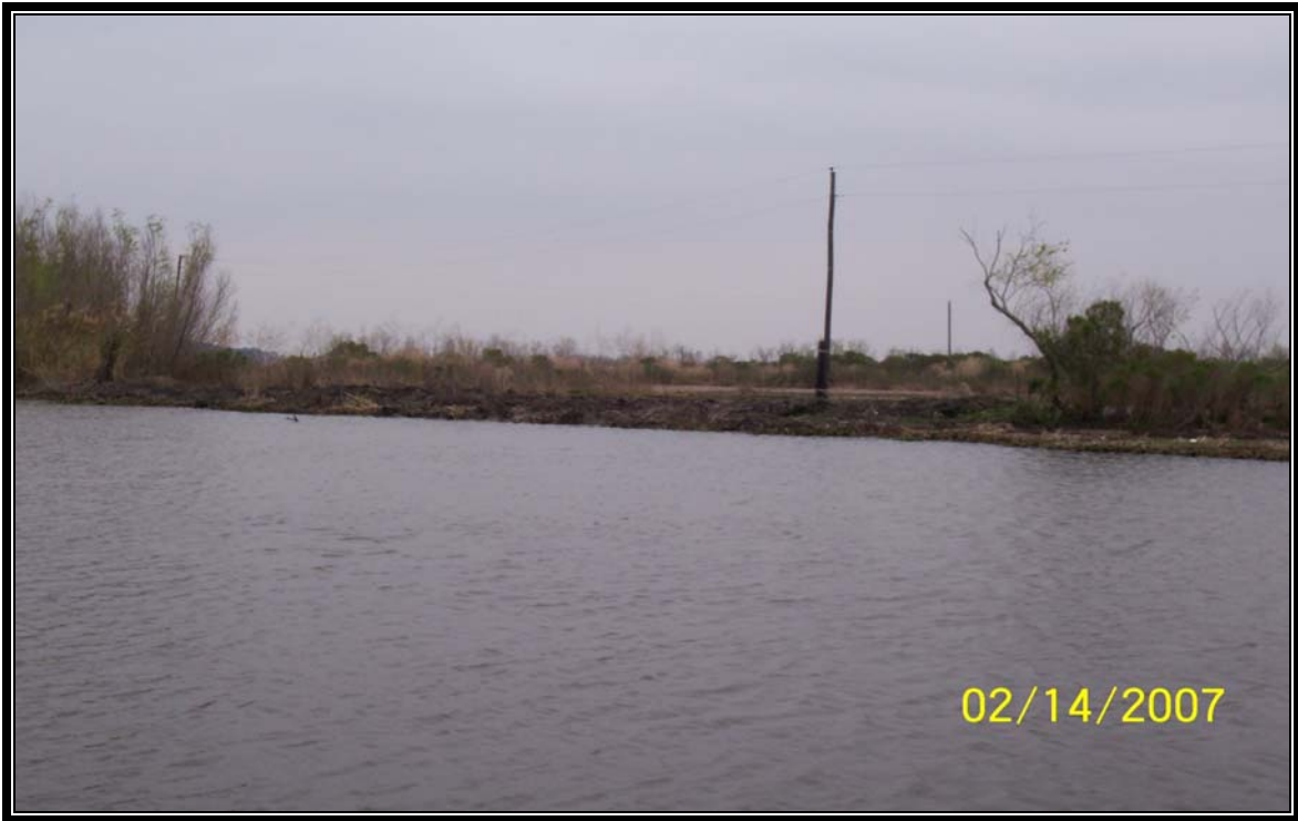
Photo 31 – Breach repair completed in 2006 by Apache Corporation along Brady Canal near the Bayou Penchant and the Apache Camp.
