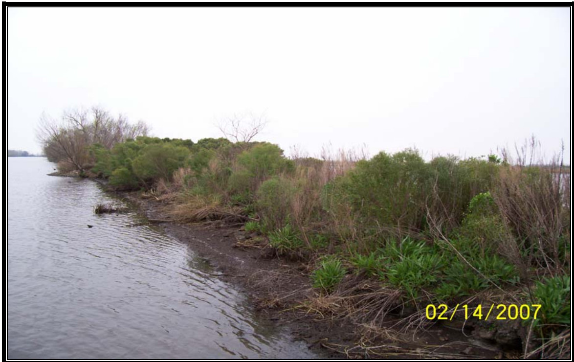
Photo 24 – (Breach Repair 9) – levee refurbishment along Superior Canal completed in 2003.
