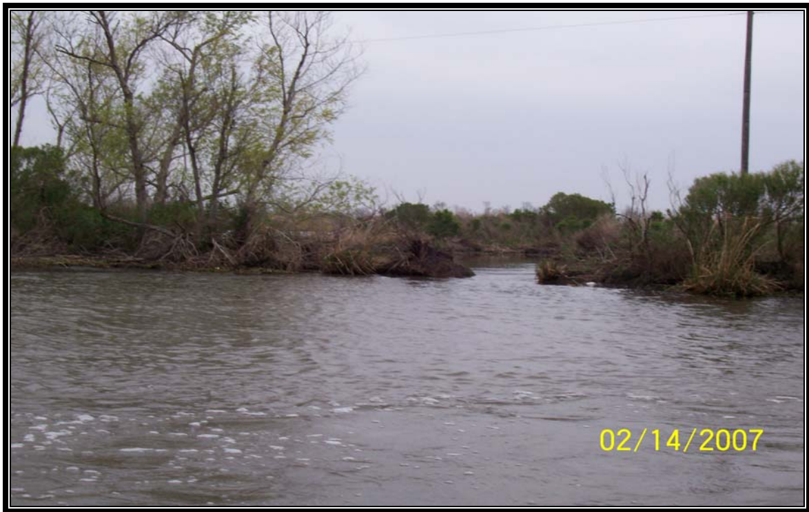
Photo 37 – Newly discovered breach along the south bank of Brady Canal on the northern boundary of the project.
