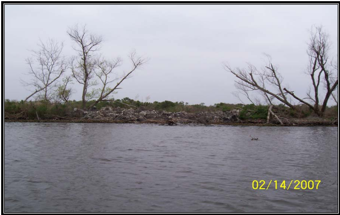
Photo 29 – Breach repair completed in 2006 by Apache Corporation along Carencro Bayou.
