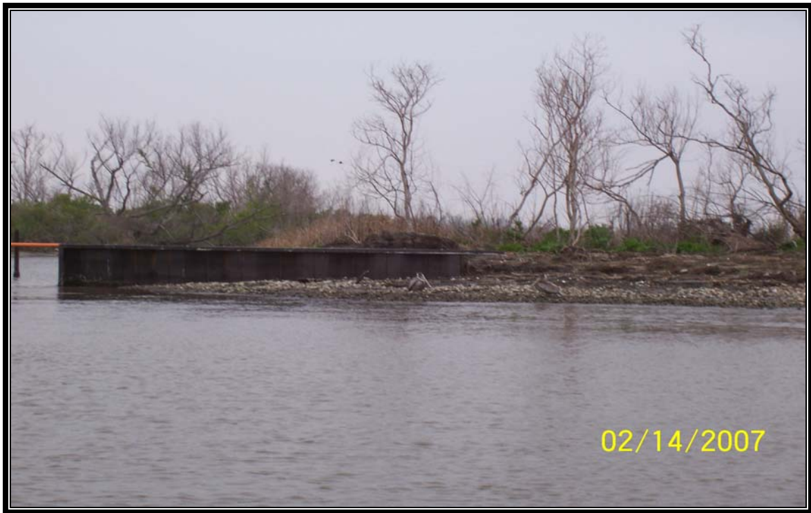
Photo 13 – (Structure 21) – earthen embankment tie-in on the north side of the structure.
