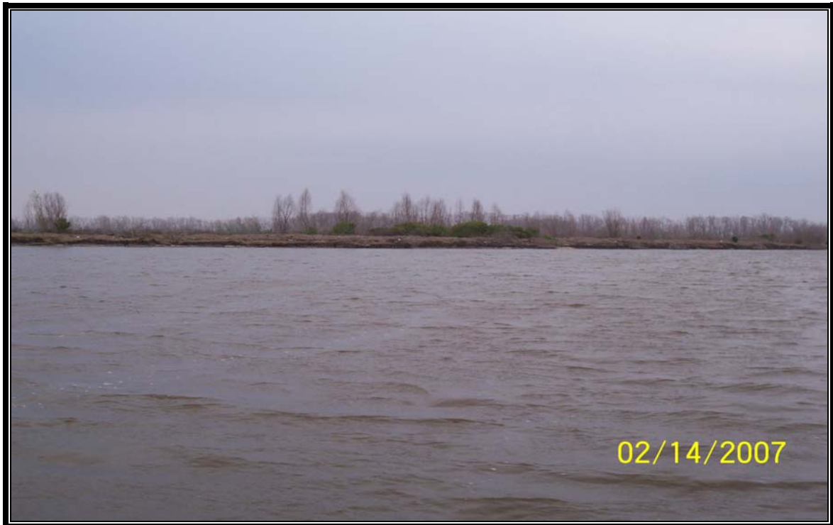
Photo 18 – (Breach Repair 5 and 6) – Levee refurbishment along Turtle Bayou completed in 2003.
