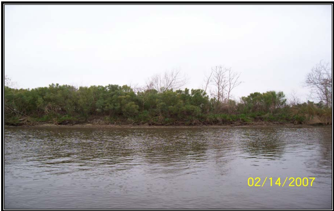
Photo 22 – (Breach Repair 8) – levee refurbishment along Superior Canal completed in 2003.
