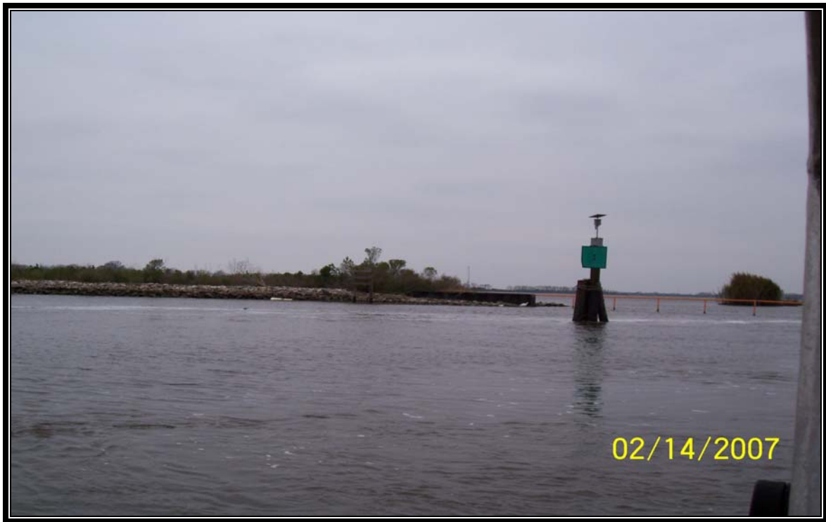
Photo 3 – (Structure 6) – southwest bank tie-in of structure 6.
