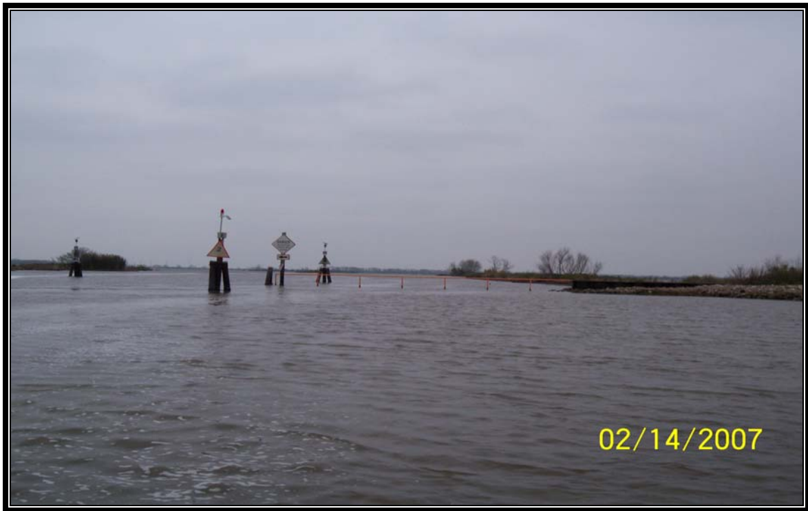
Photo 1 – (Structure 6) – fixed crest weir with barge bay along the north bank of Bayou Decade.
