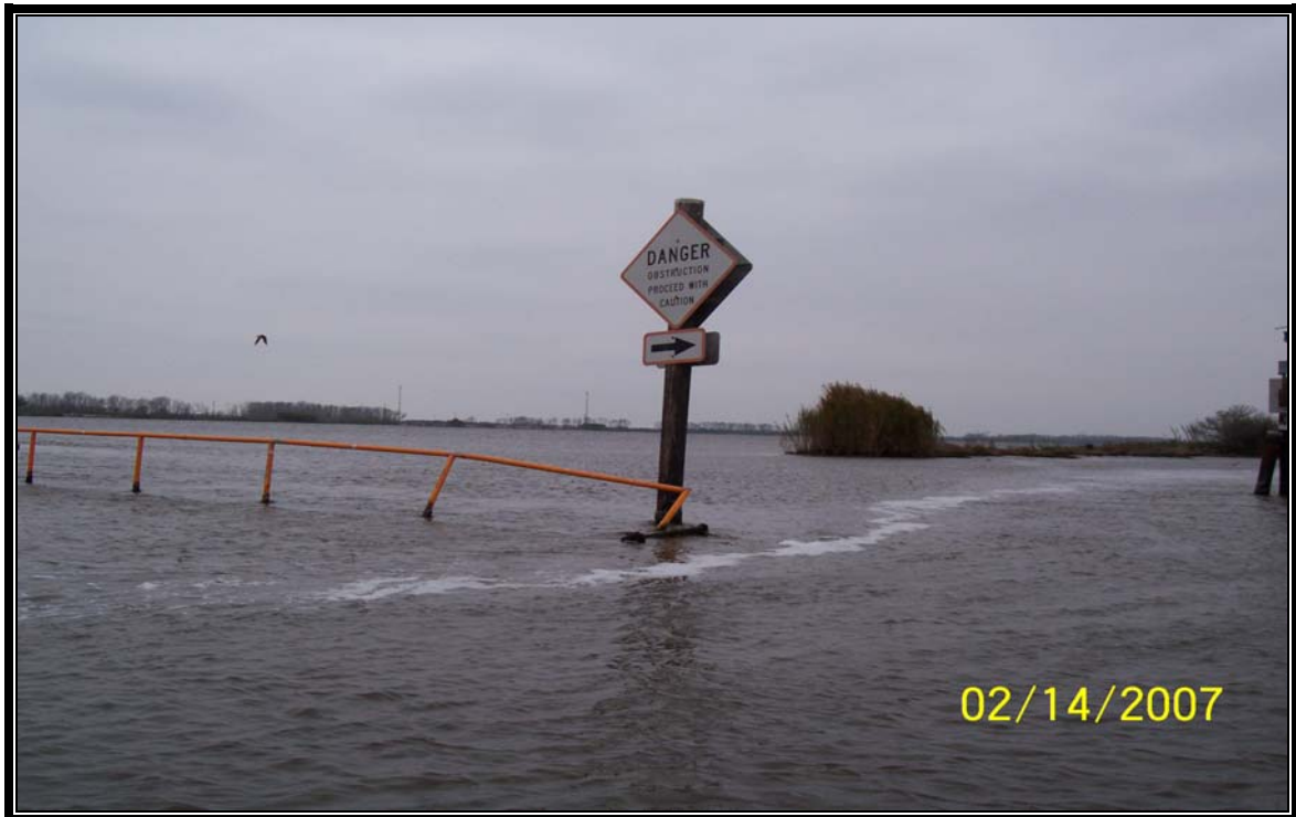
Photo 4 – (Structure 6) – location of missing timber piling and damage to guardrail on bulkhead.
