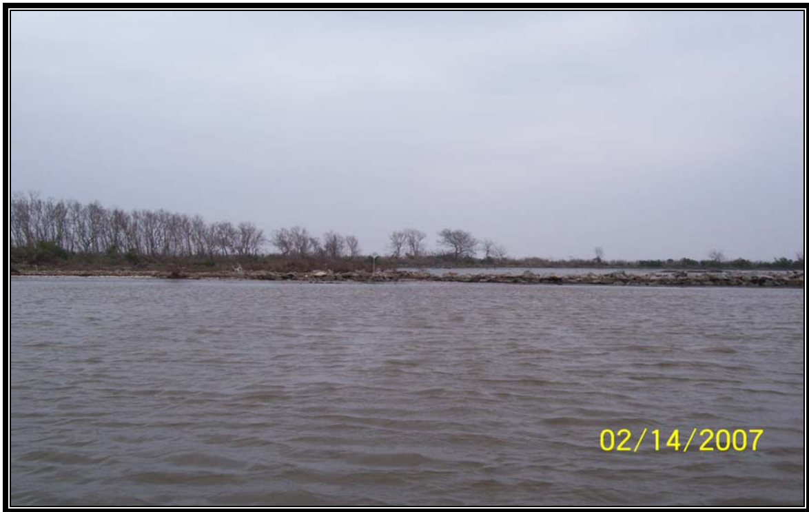
Photo 17 – (Breach Repair 1 through 4) – rock dike constructed in 2003 to close large openings in the bank.
