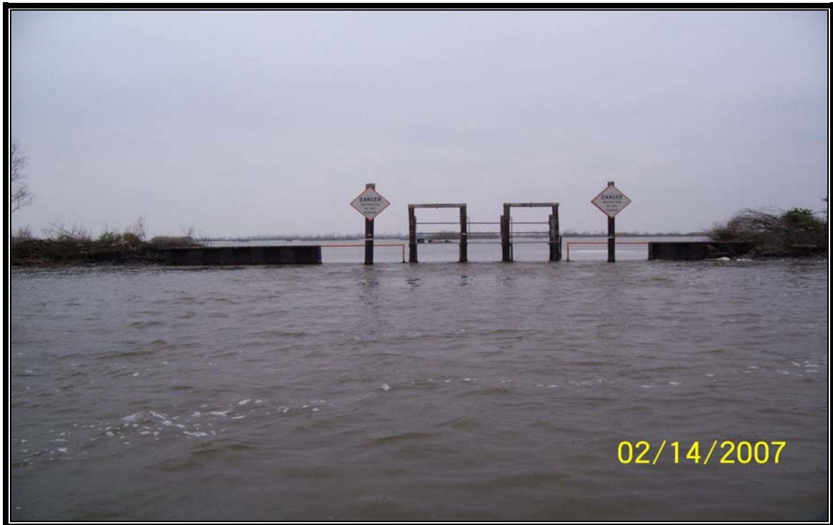
Photo 14 – (Structure 23) – variable crest weir located along the northeast bank of Jug Lake.
