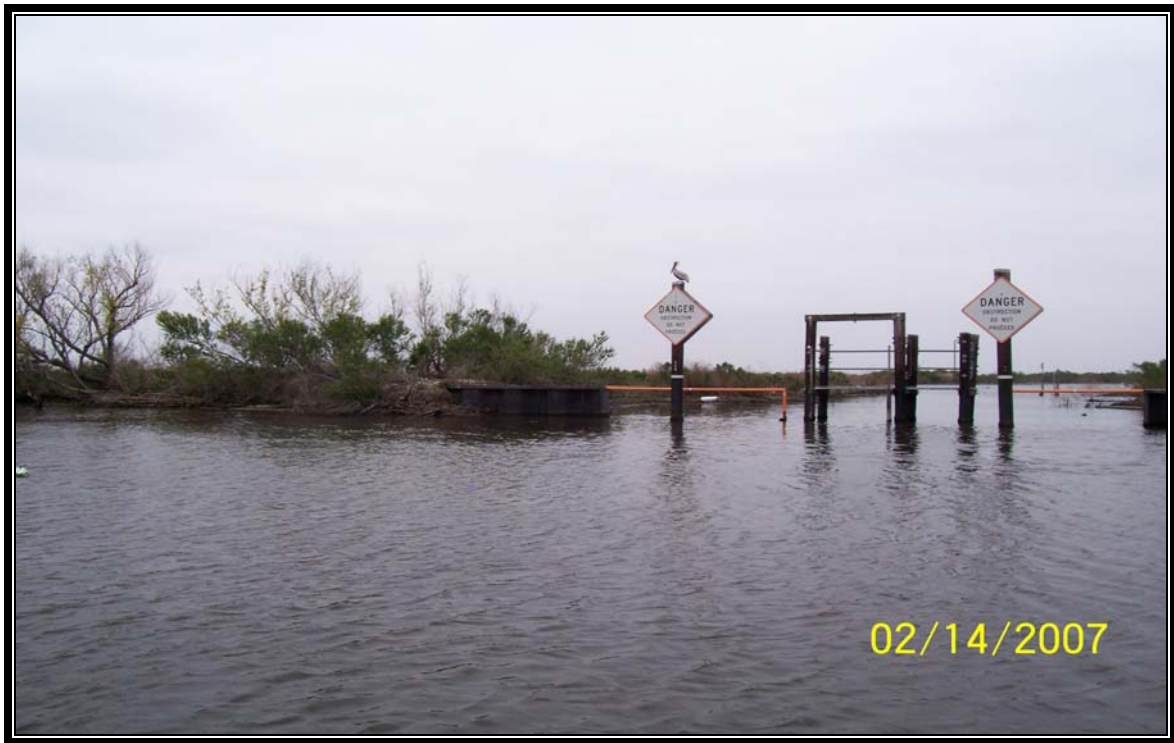
Photo 11 – (Structure 14) – northern tie-in of variable crest weir along Carencro Bayou.
