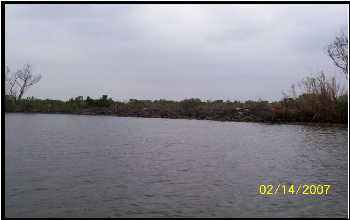
Photo 30 – Breach repair completed in 2006 by Apache Corporation along Carencro Bayou.
