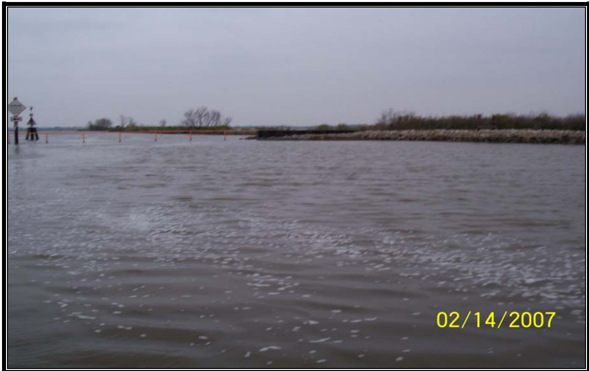
Photo 2 – (Structure 6) – northeast bank tie-in of structure 6.
