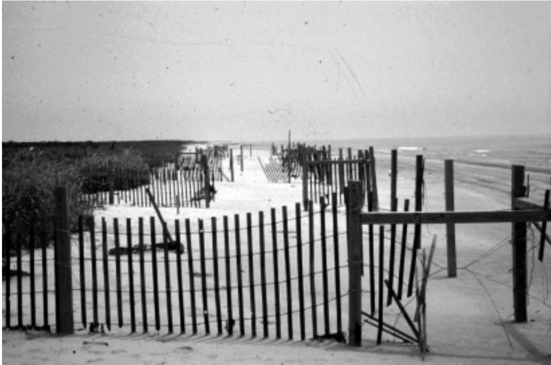
Figure 4. Typical destruction of fencing and vegetation at Timbalier Island Plantings (TE-18) Demonstration project (photo taken August 1997).
