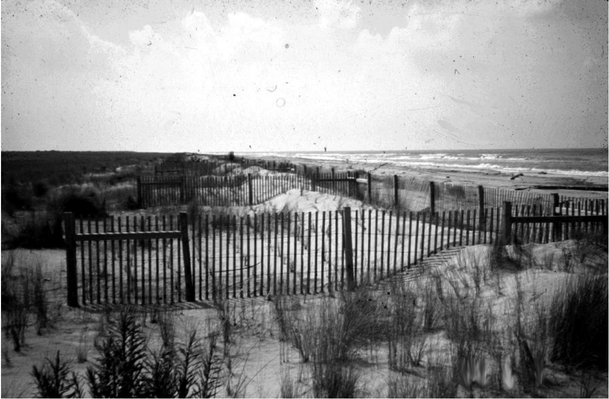
Figure 2. Typical sand fencing with perpendicular spurs at Timbalier Island Plantings (TE-18) Demonstration project (photo taken August 1996).
