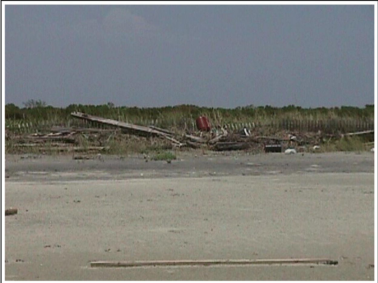
Figure 7. Typical fences after impacts from storm waves and debris at Timbalier Island Plantings (TE-18) Demonstration project (photo taken July 1998).
