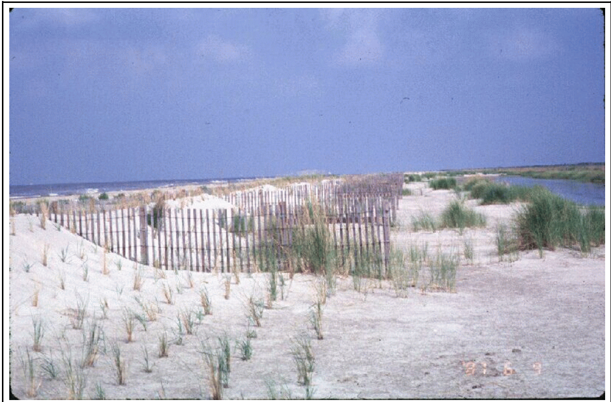
Figure 2. Typical sand fencing with perpendicular spurs at Timbalier Island Plantings (TE-18) Demonstration project (photo taken July 1996).
