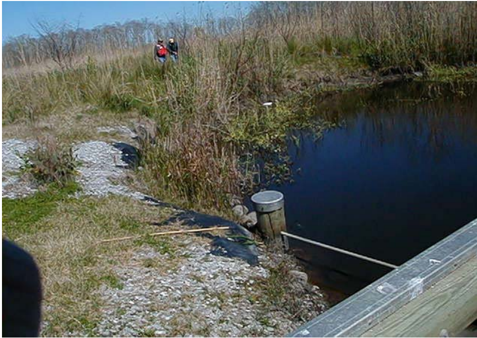
Photo 3—exposed cloth around structure
