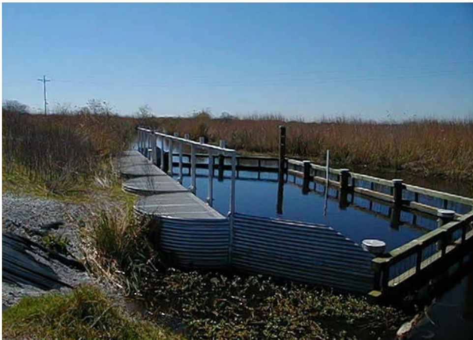
Photo 4—inlet side of structure and hyacinth guard
