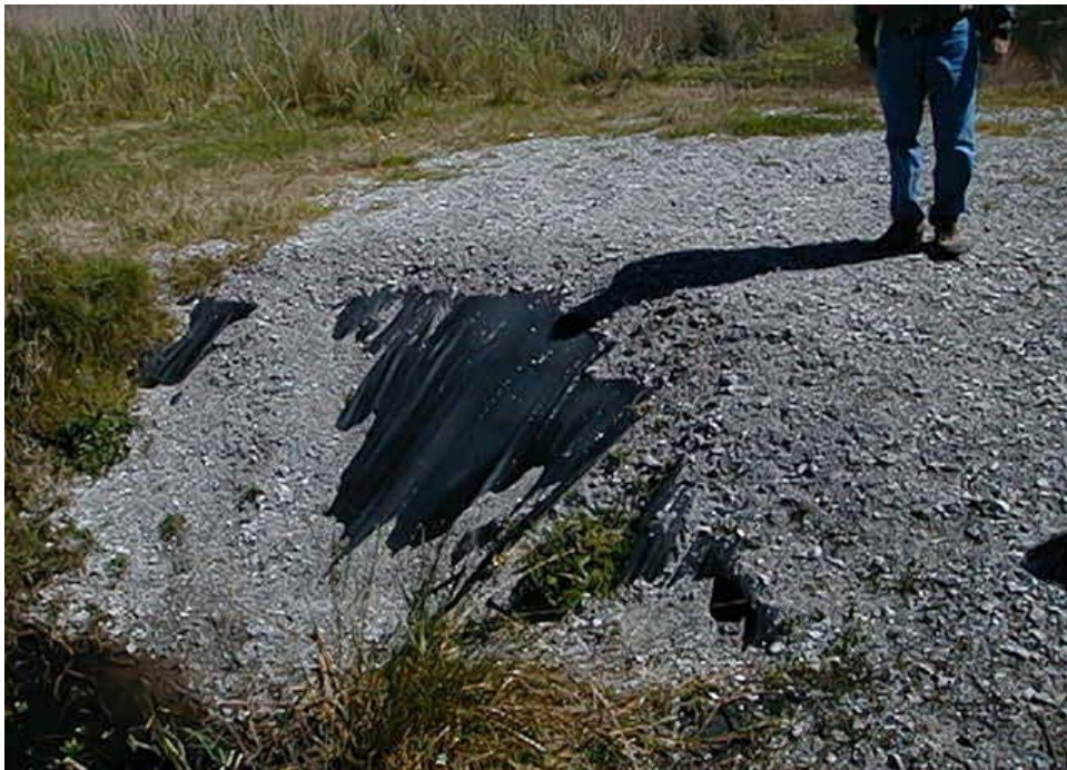
Photo 2—sloughing rock around structure
