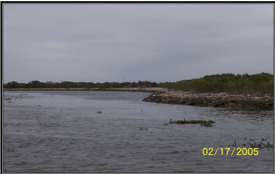
Shoreline Protection – earthen embankment with rock revetment located along Voss Canal south of Structure No.10. (Photo 67, looking north)
