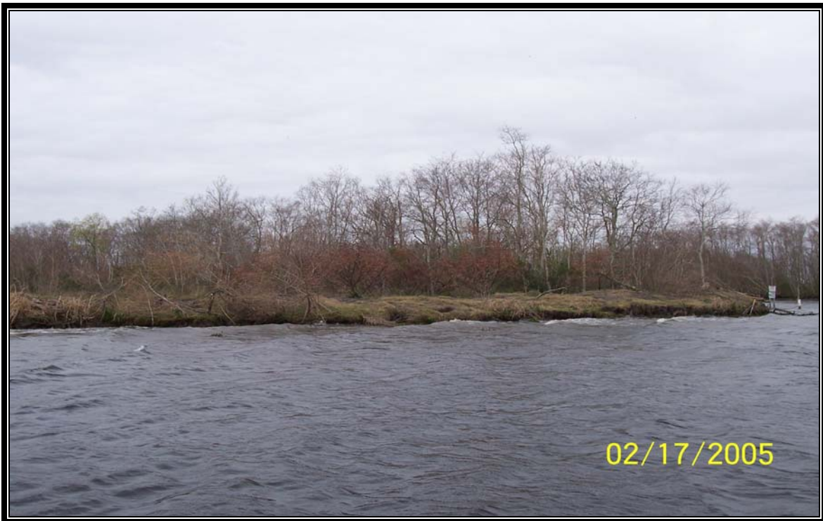
Breach 5&6 – Levee refurbishment along Turtle Bayou beginning near Superior Canal and commencing 1,500' southward completed under the 2003 Maintenance Project. (Photo 13, looking west)
