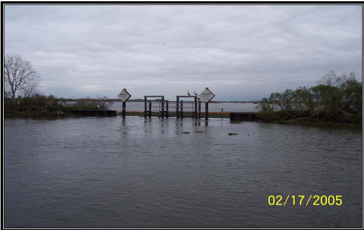
Structure No.23 – Fixed crest weir structure with two (2) variable crest weir sections located along the north shoreline of Jug Lake (Photo 30, looking northeast)
