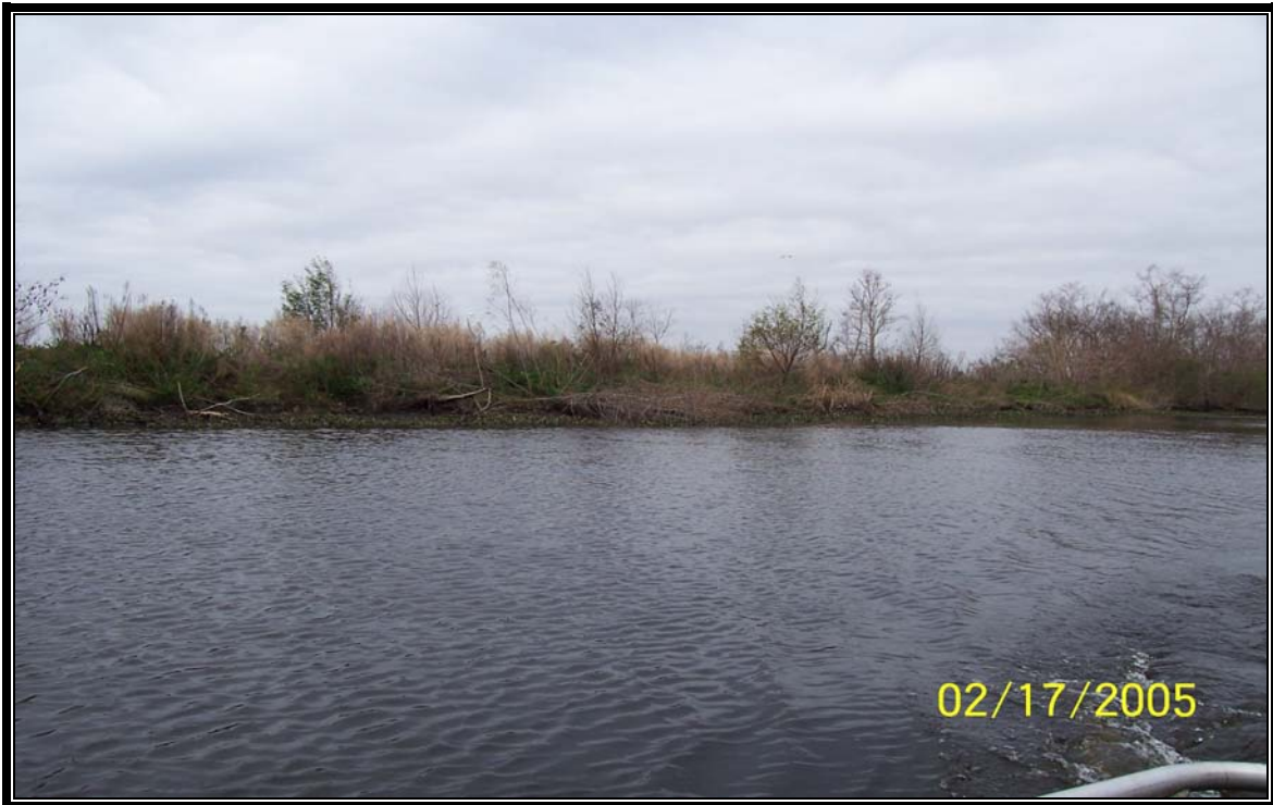
Breach 9 – Earthen embankment refurbished along Superior Canal completed under the 2003 Maintenance Project (Photo 12, looking west)
