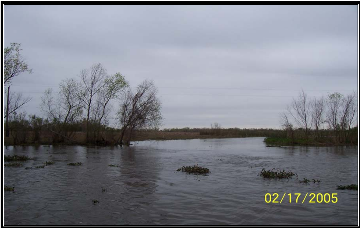
Large breach located along the south bank of Brady Canal southwest of the Apache camp. Breach connects to a second breach located along Bayou Penchant. (Photo 75, looking southeast)
