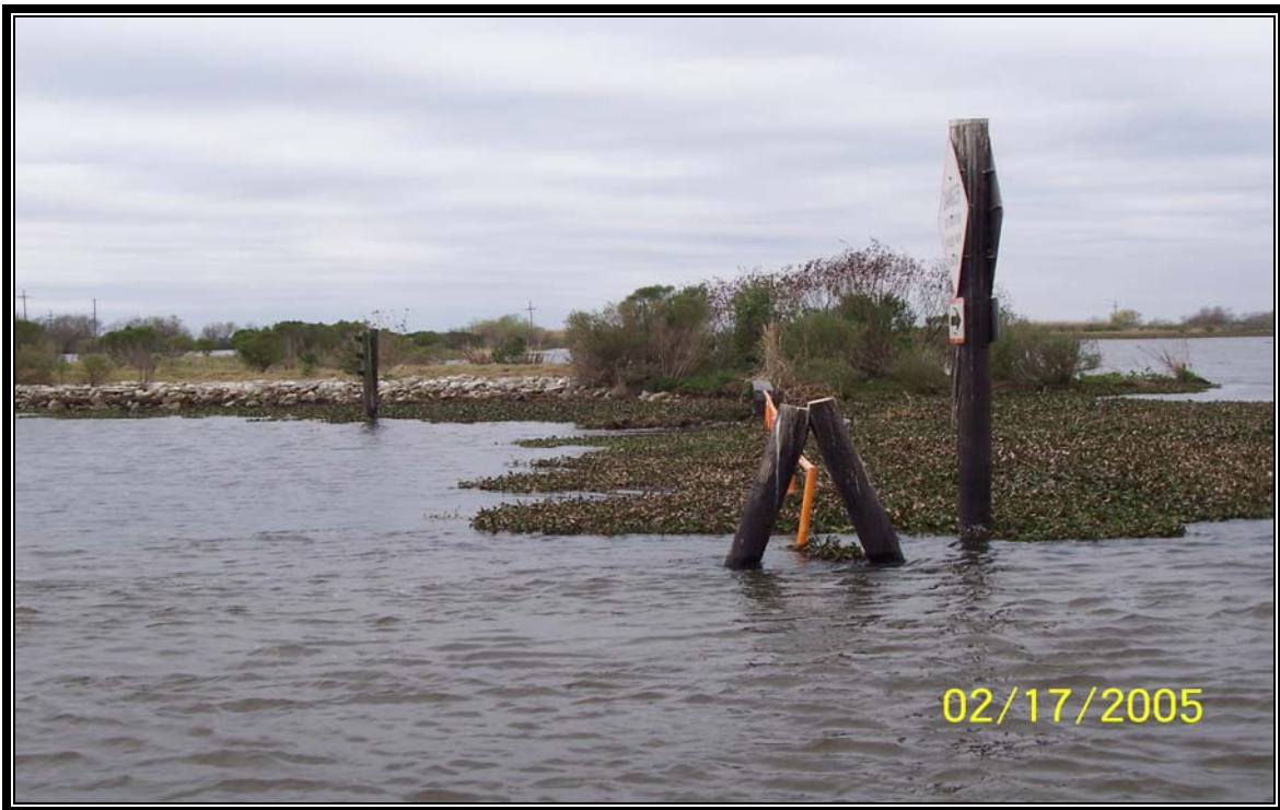
Structure No.6 – steel sheet pile wall on the west side of the structure located along Bayou Decade south of Bayou Loutre. Slight damage to guard rail and timber piling (Photo 53, looking west)
