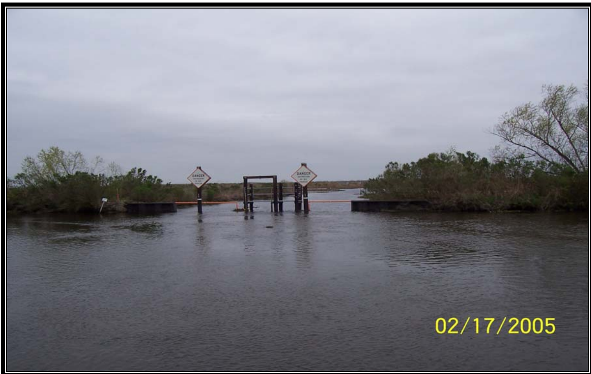
Structure No.14 – fixed crest weir structure with a single variable crest section located along the east bank of Carencro Bayou just south of the “Better Livin” camp (Photo 72, looking east)
