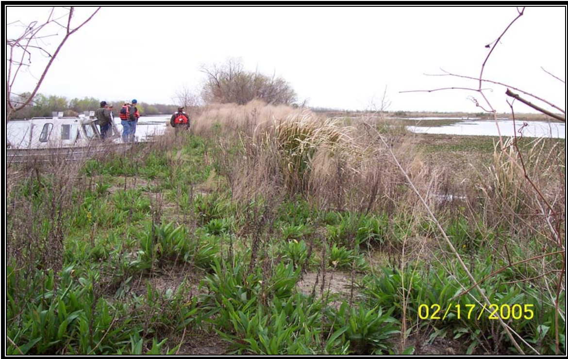
Breach 8 – Earthen embankment refurbishment along Superior Canal completed under the 2003 Maintenance Project (Photo 10, looking south)
