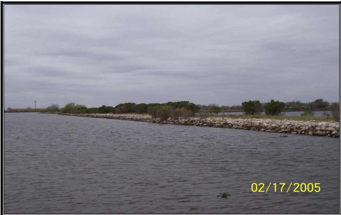
Earthen embankment with rock revetment located along the north bank of Bayou Decade. (Photo 55, looking northwest)
