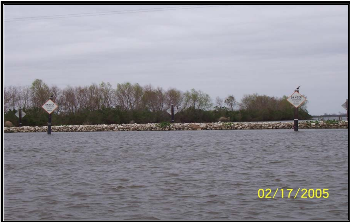
Structure No.7 – rock riprap plug located along the north bank of Bayou Decade south of Bay Long. (Photo 59, looking north)
