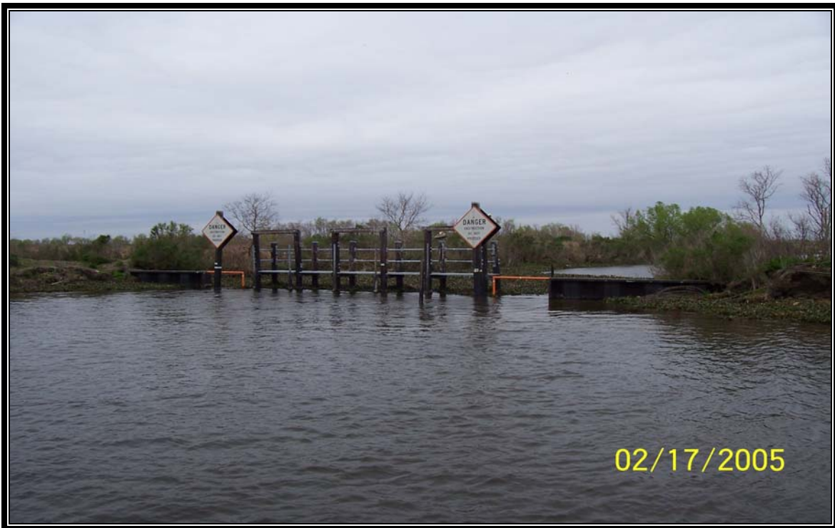
Structure No.21 – fixed crest weir structure with three (3) variable crest sections located along the northwest bank of Jug Lake. (Photo 38, looking west)
