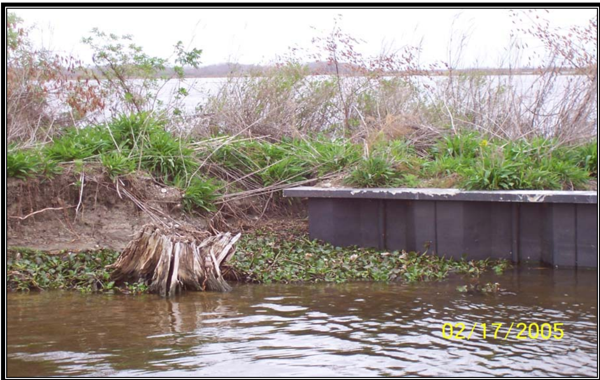
Structure No.23 – earthen embankment tie-in on the north side of the structure were erosion around the sheet pile wall is evident (Photo 37, looking east)
