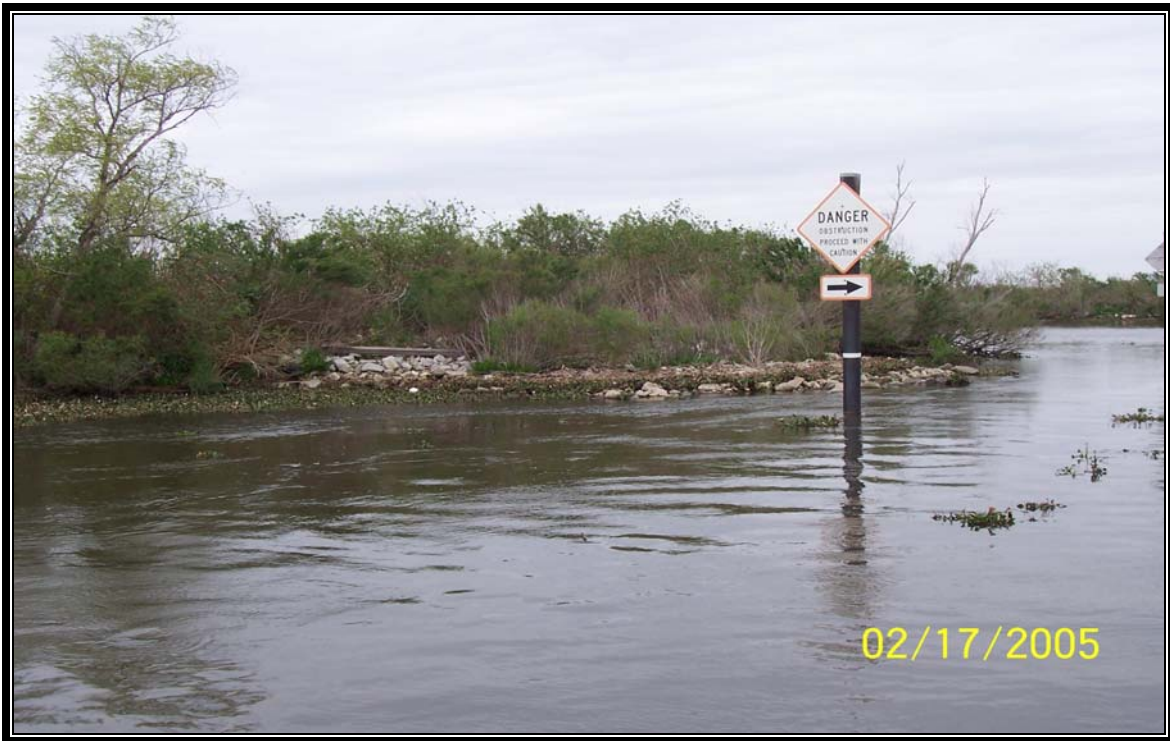
Structure No.20 – south side of riprap lined channel section across Bayou Loutre entering Jug Lake (Photo 49, looking west)
