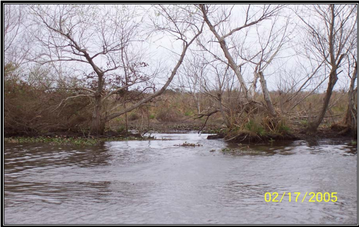
Small breach located along Carencro Bayou south of Structure No. 14 near an existing power line. (Photo 71, looking east)
