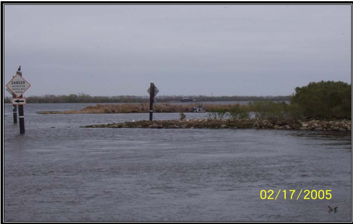
Structure No.10 – south bank tie-in of rock riprap lined channel entering Bay Long from Voss Canal (Photo 68, looking east)
