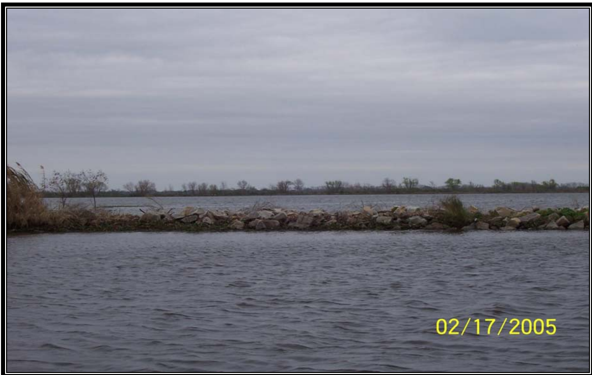
Breach 1 thru 4 – rock dike constructed under the 2003 Maintenance Project to shore up an existing earthen embankment along Bayou Decade between Jug Lake and Turtle Bayou which was breached in several locations (Photo 22, looking north)
