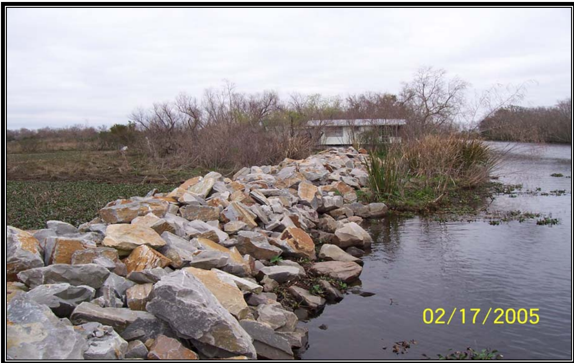
Breach 7 – Existing breach repair under 2003 Maintenance Project located at the end of an oil field location canal west of Superior Canal (Photo 3, looking east)
