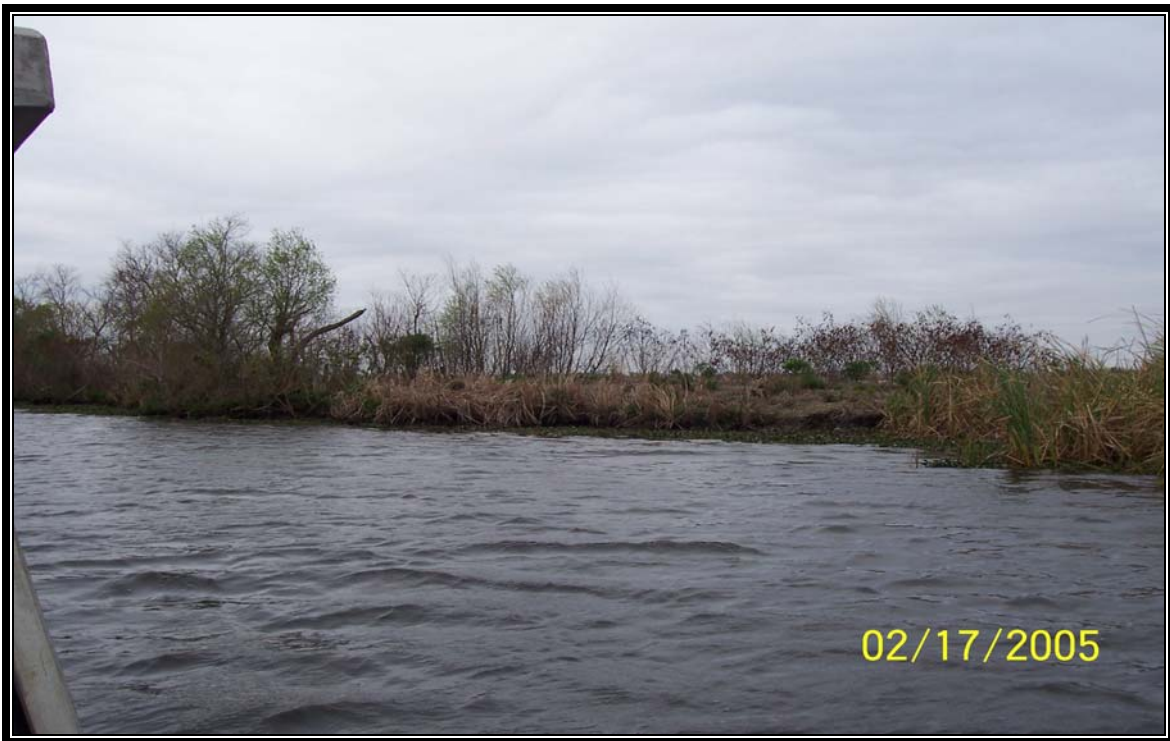
Location of breach repaired by Apache Corporation along the west bank of Turtle Bayou (Photo 21, looking west)
