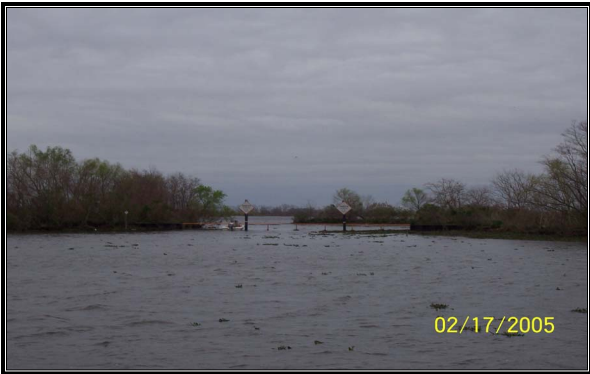
Structure No.24 – fixed crest weir structure located along the east bank of Jug lake (Photo 25 – looking east)
