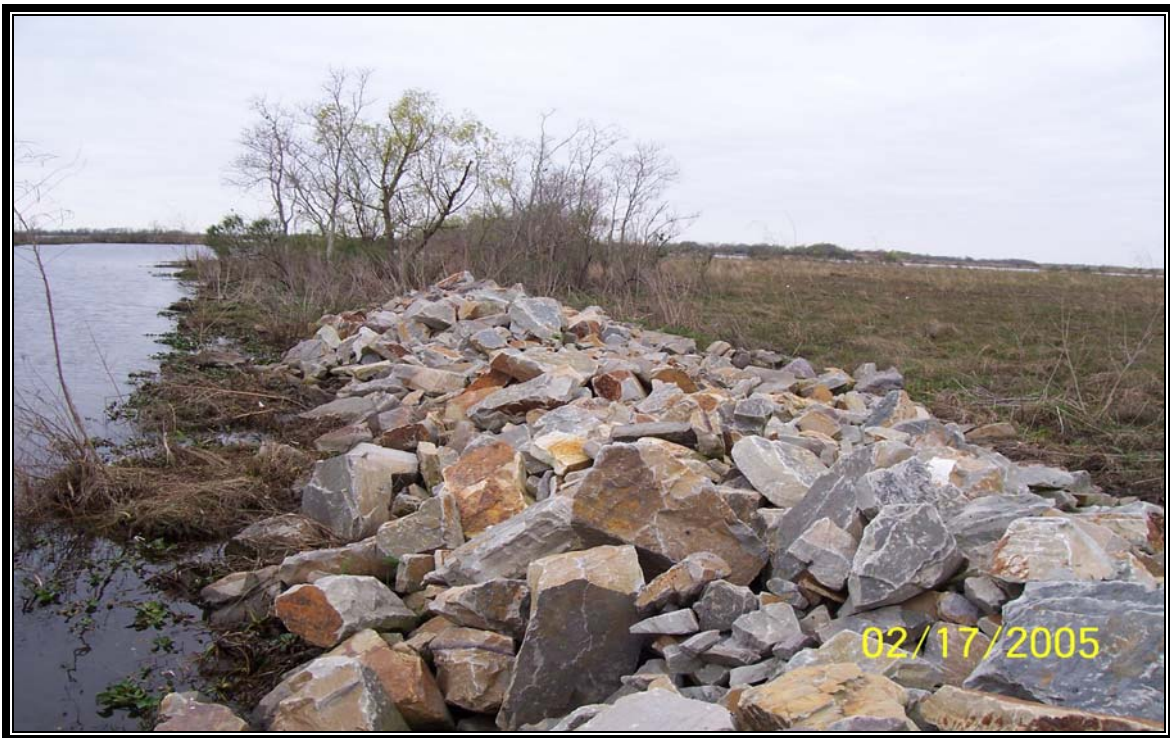
Breach 7 – Existing Breach repair under 2003 Maintenance Project located at the end of an oil field location canal west of Superior Canal. (Photo 2, looking west)
