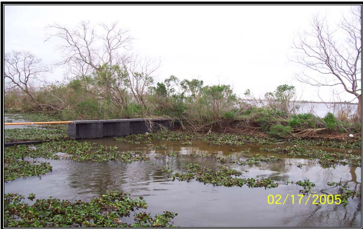
Structure No.24 – south bank tie-in of the fixed crest weir structure looking southeast (Photo 26).
