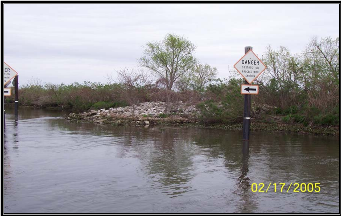
Structure No.20 – north side of rock riprap lined channel across Bayou Loutre entering the west bank of Jug Lake. (Photo 48, looking west)
