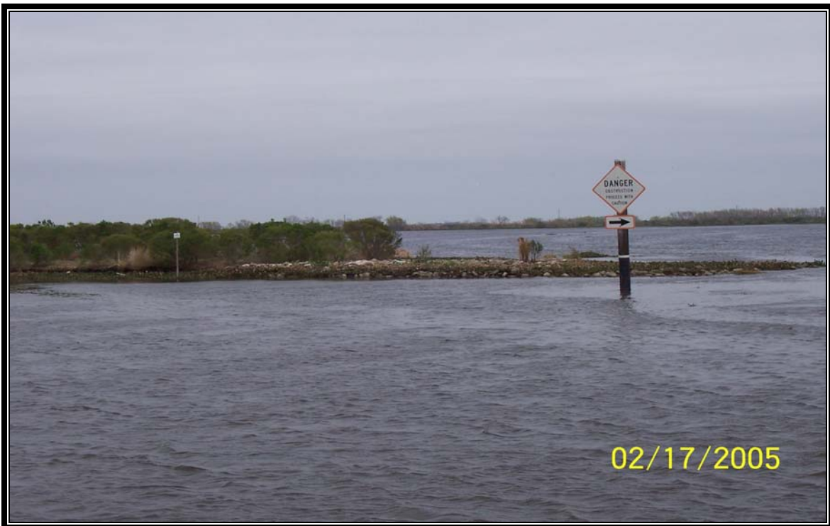
Structure No.10 – north bank tie-in of rock riprap lined channel located at the entrance to Bay Long from Voss Canal. (Photo 69, looking east)
