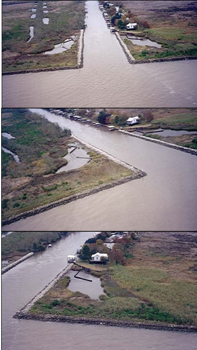
Figure 10. Boston Canal/Vermilion Bay Shoreline Stabilization (TV-09) rock dike and sediment fences at the mouth of Boston Canal (January 2001).
