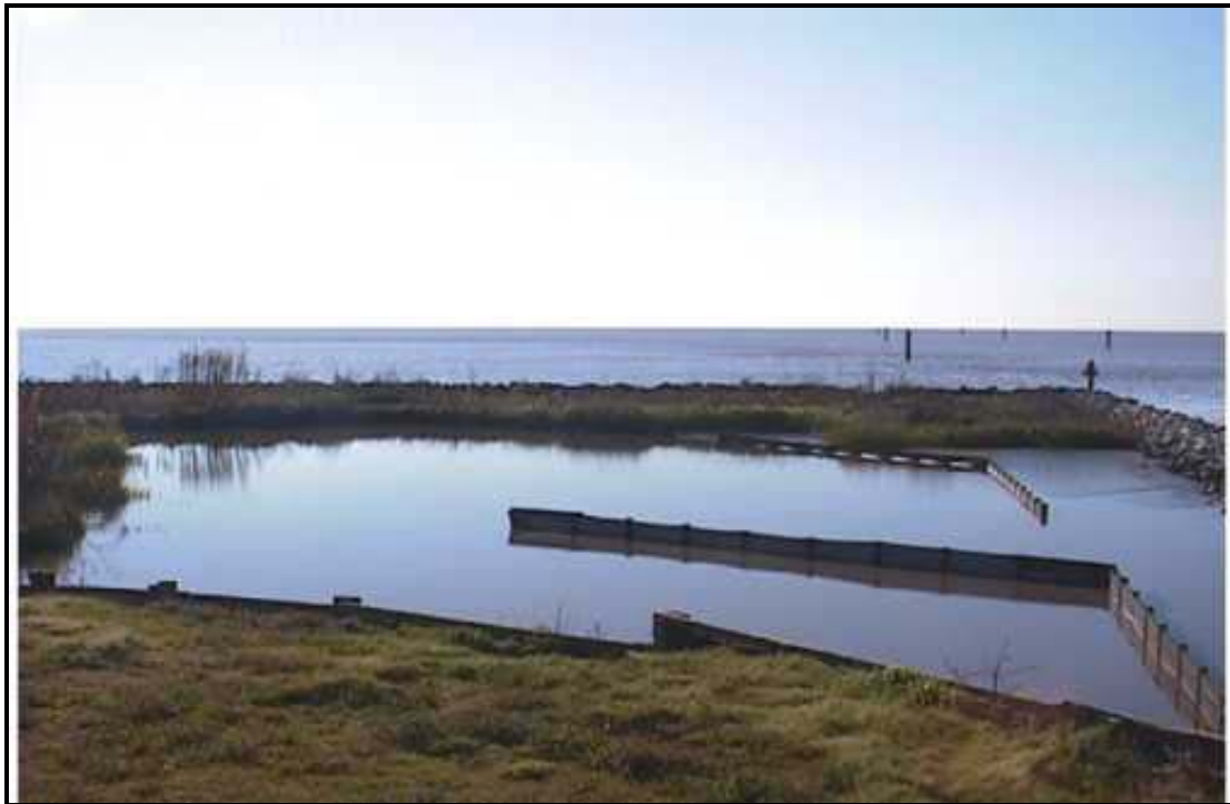
Figure 11. Boston Canal/Vermilion Bay Shoreline Stabilization (TV-09) photographs: (Upper) sedimentation behind the dike December 1994; (Lower) vegetation growing behind the dike in February 1998.
