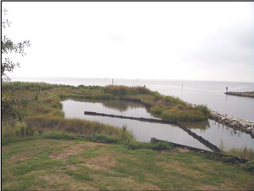
Figure 12. Boston Canal/Vermilion Bay Shoreline Stabilization (T/V-09) photographs: (Upper) vegetation behind the dike (July 1999); (Lower) vegetation behind the dike in October 2001.
