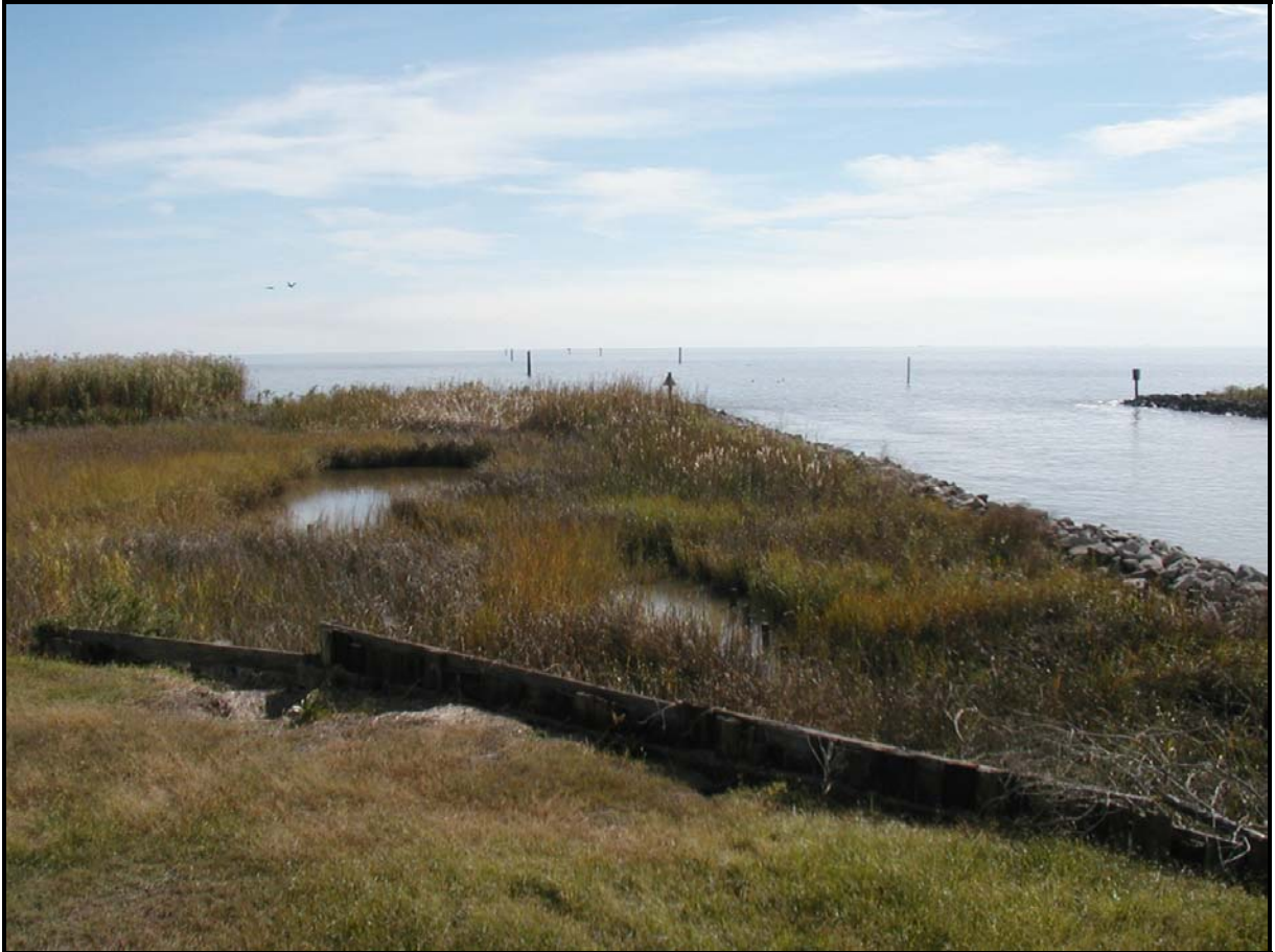
Figure 13. Boston Canal/Vermilion Bay Shoreline Stabilization Project (TV-09) behind the eastern rock dike, November 9, 2004.
