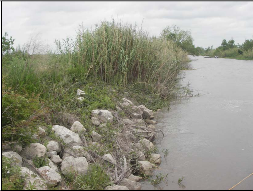
Photo 3, Tie-in to North Prong Ditch
