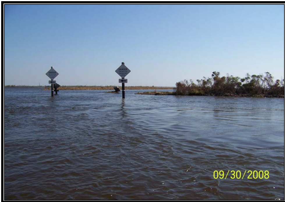
Photo No.8 – view of the south side of the rock channel liner (Structure No.10) along Voss Canal. The warning signs in the background of the photo are leaning over as a result of strong winds from Hurricanes Gustav and Ike.
