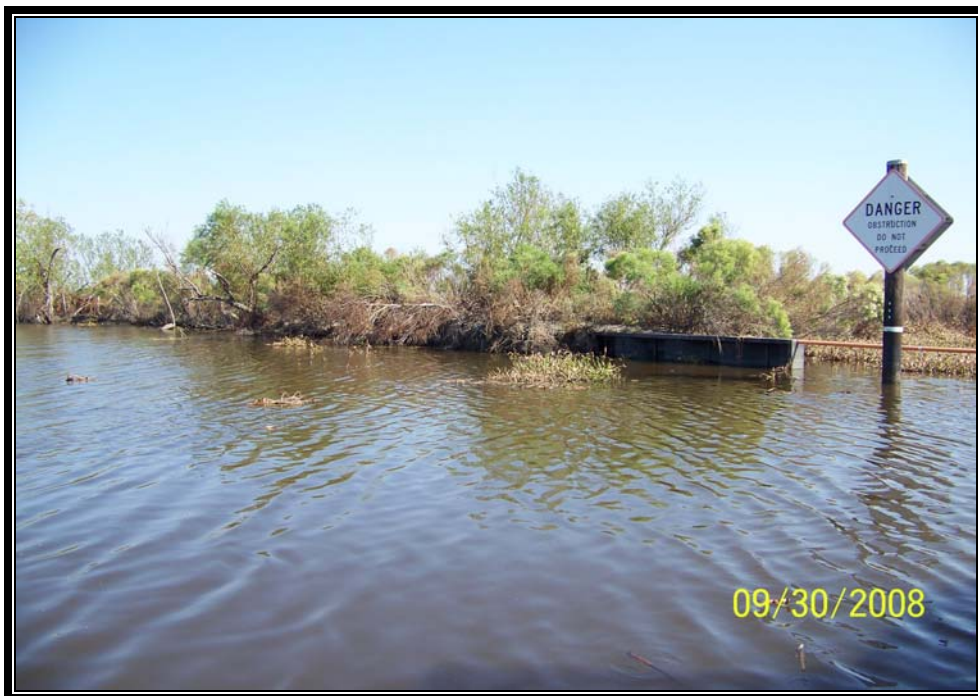
Photo No. 14 – View of the steel bulkhead on the north side of the variable crest weir (Structure 14) along Little Carencro Bayou.
