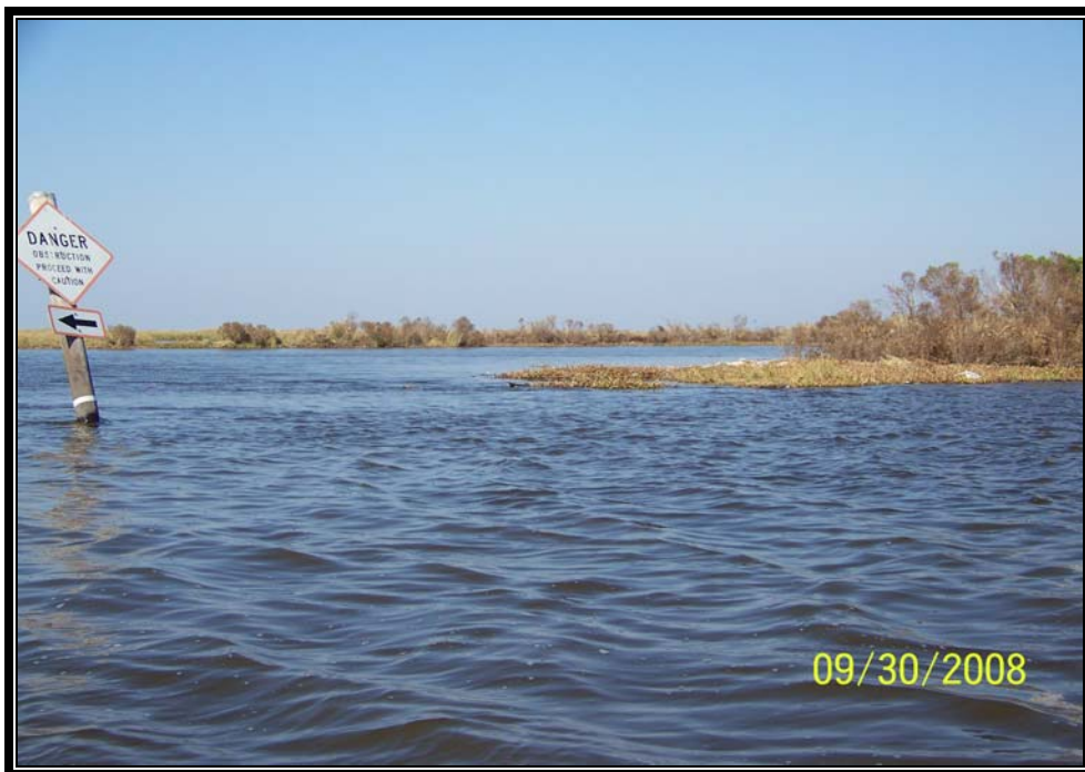
Photo No.10 – The interior warning sign on the north side of the rock channel liner (Structure No.10) along Voss Canal.
