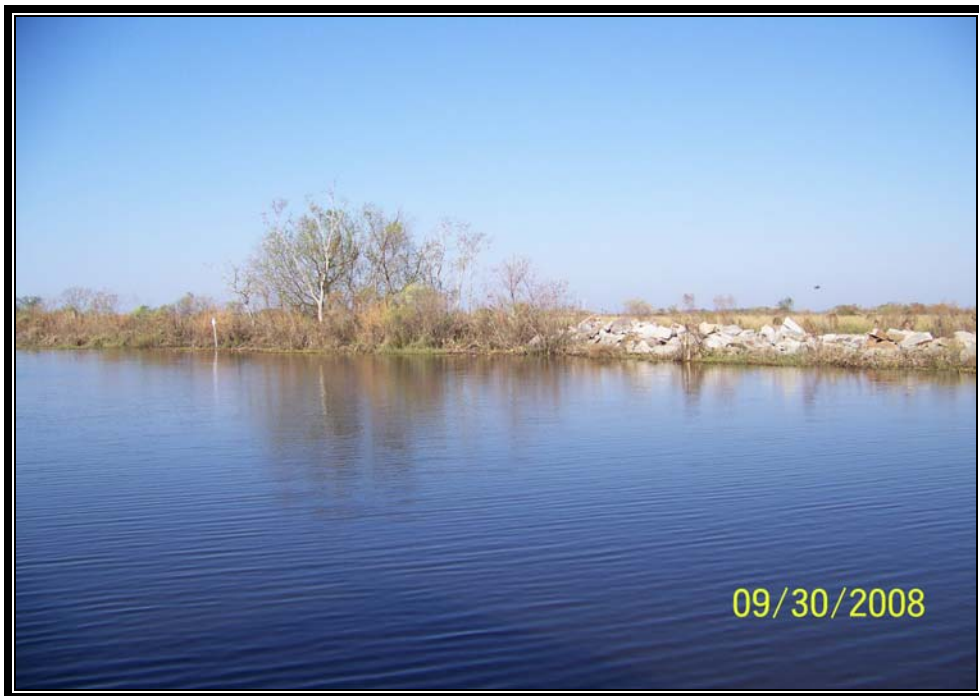
Photo No.34 - View of rock plug (Breach 7) to bank tie-in on the southwest side of the structure.
