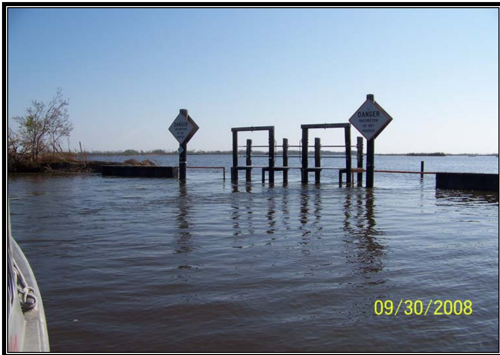
Photo No.22 – An overall view of the two (2) bay variable crest weir (Structure No.23) looking north.
