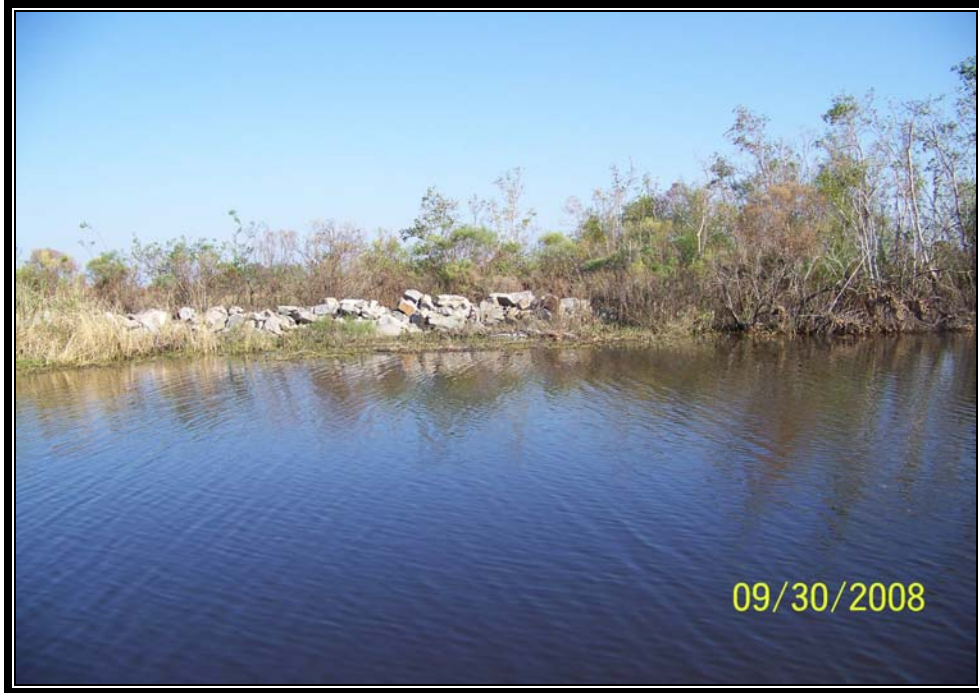
Photo No. 33 – View of rock plug (Breach 7) to bank tie-in on the northeast side of the structure.
