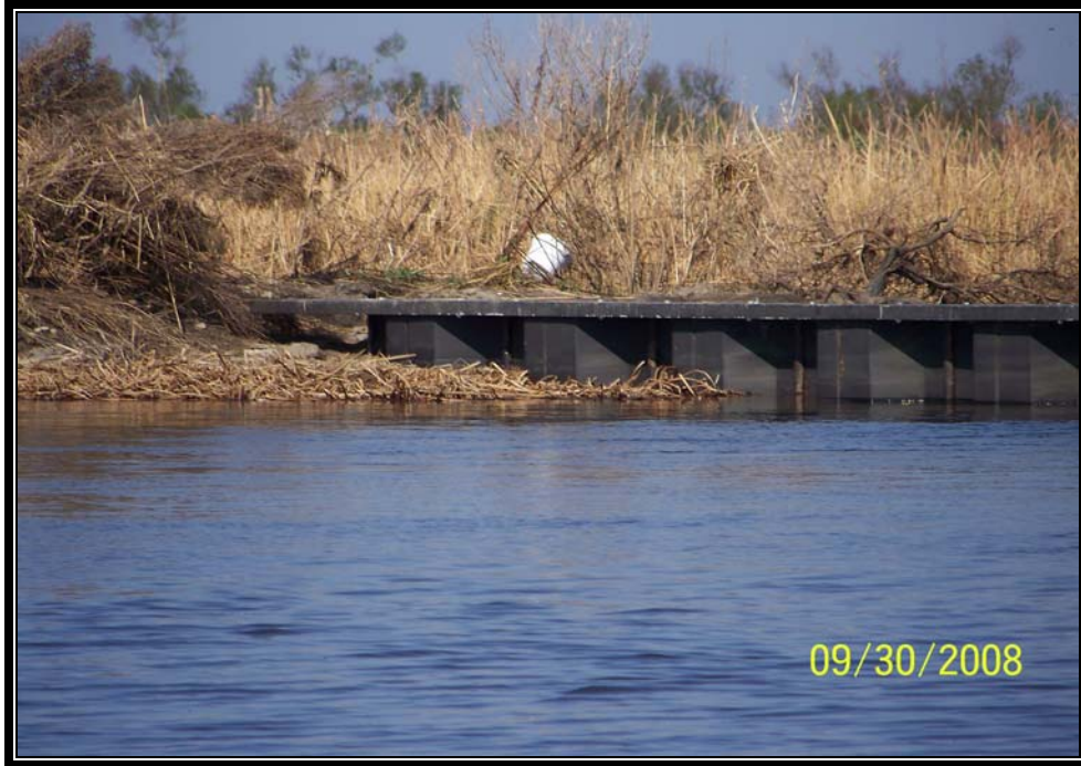
Photo No.19 – View of the southern end of the steel bulkhead at Structure No. 21. Observed moderate erosion of the earthen embankment exposing the end of the bulkhead.
