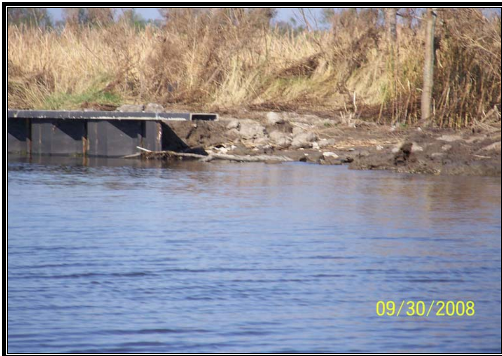
Photo No. 18 – View of the northern end of the steel bulkhead at Structure No.21. Although there was no breach present, the earthen embankment had eroded back beyond the face of the bulkhead exposing the end of the structure.
