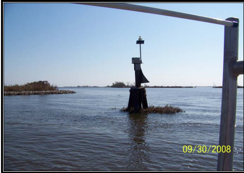
Photo No. 3 – View of the timber navigational structure on the southwest side of Structure No.6.
