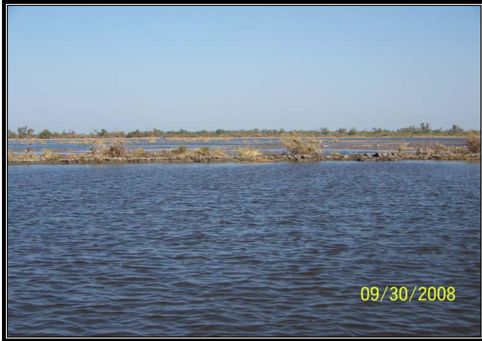
Photo No. 43 – View of shoreline on the west side of Jug Lake between Structures No. 20 and 21.
