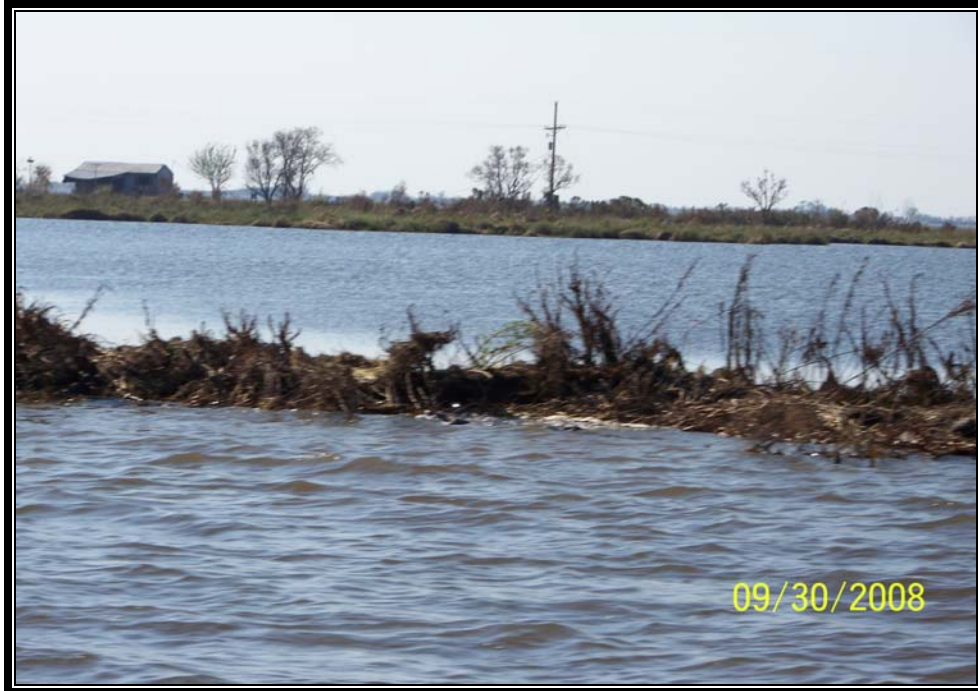
Photo No.37 – View of the existing bank along the southeast shoreline of Jug Lake south of Structure No.24. As evident in the photo, the existing bank line sustained extensive damage from Hurricane Ike. There is very little bank line remaining in this area.
