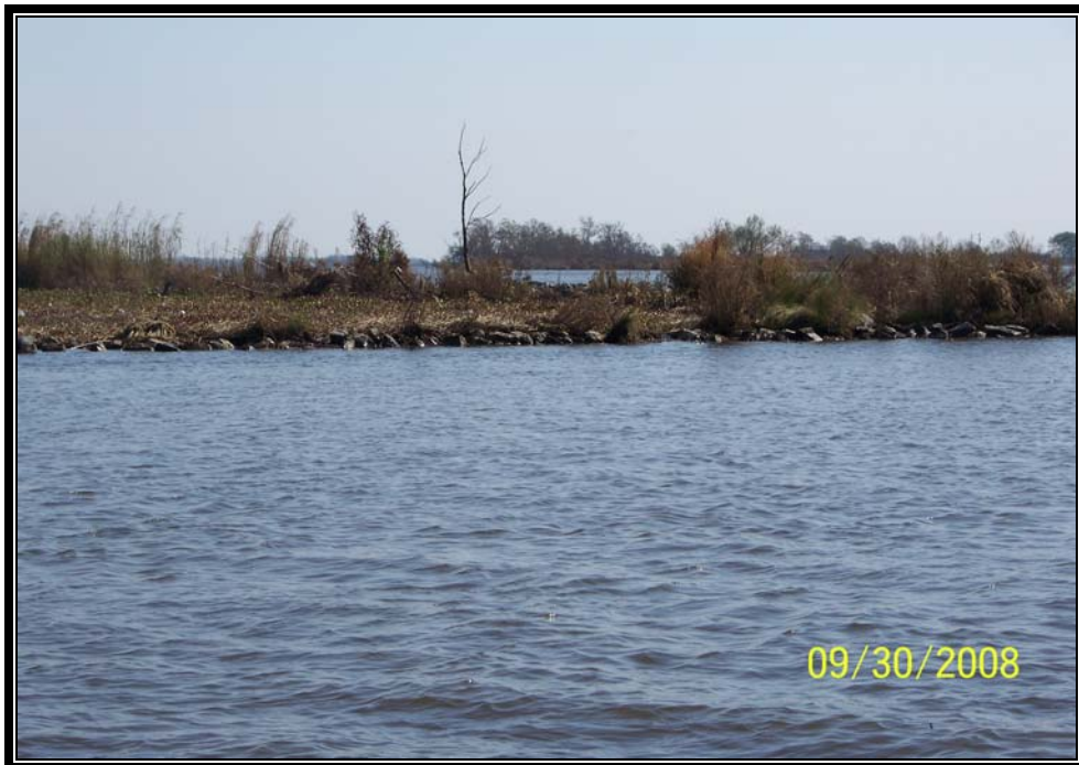
Photo No.6 – view of the north bank of Bayou Decade west of Structure No.6
