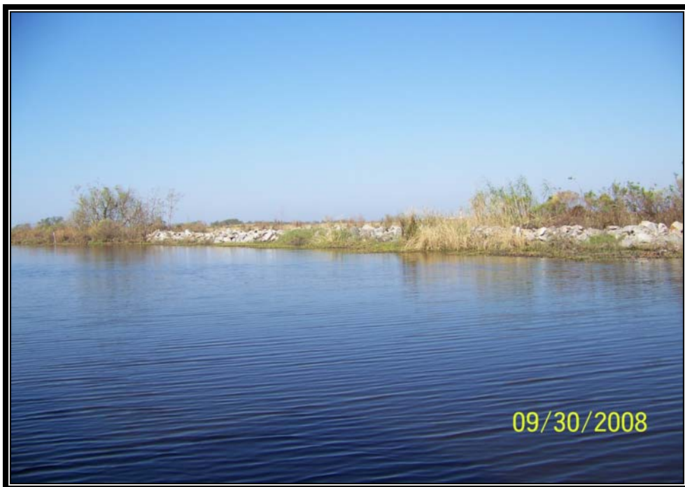
Photo No. 32 - View of the rock plug constructed in 2003 (Breach 7) along the north bank of an existing oilfield access canal off of Superior Canal.
