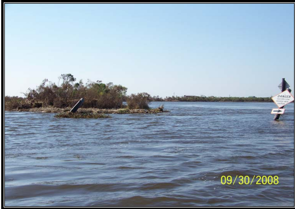
Photo No.11 – A closer view from the interior marsh area showing the damaged warning signs on the south side of Structure No.10.
