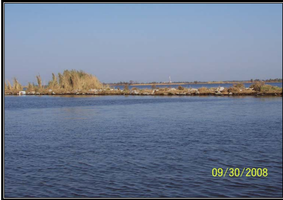
Photo No.27 - Rock dike construction in 2003 along the north bank of Bayou Decade between Turtle Bayou and Jug Lake. There appears to be a fair amount of displacement of rock from Hurricanes Katrina, Rita and Ike.
