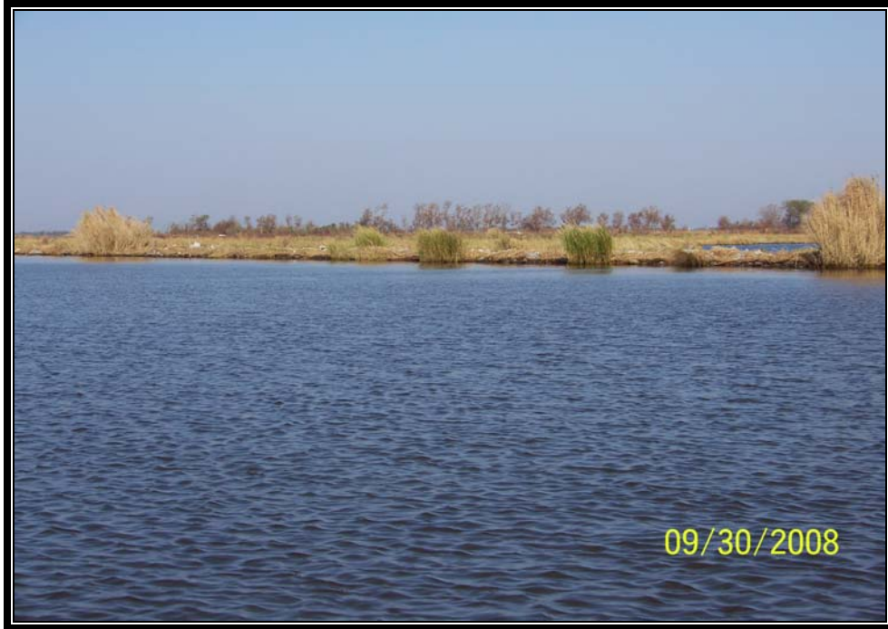
Photo No. 29 – View of rock dike along the north bank of Bayou Decade near Jug Lake.
