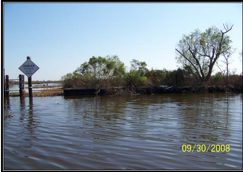
Photo No.13 – view of the steel bulkhead on the south side of the variable crest weir (Structure 14) along Little Carencro Bayou.
