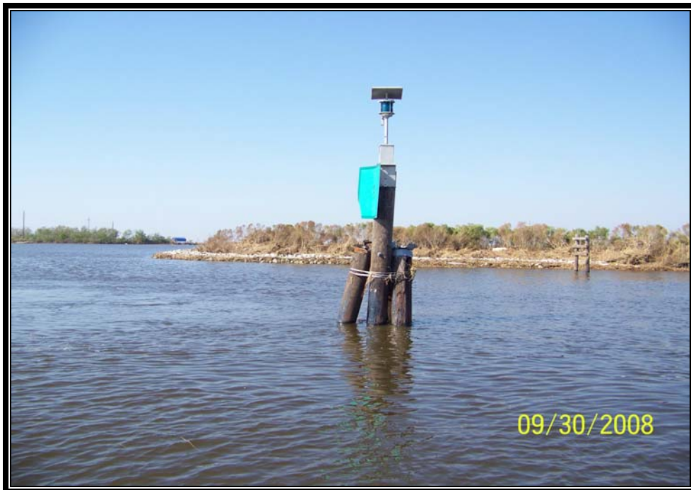
Photo No. 2 – View of the timber navigational aid structure on the southeast side of Structure No.6. The center pile of this structure was replaced in 2003.
