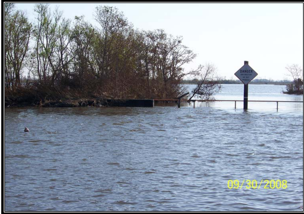
Photo No.25 – view of the northern tie-in to the earthen embankment at Structure No. 24.
