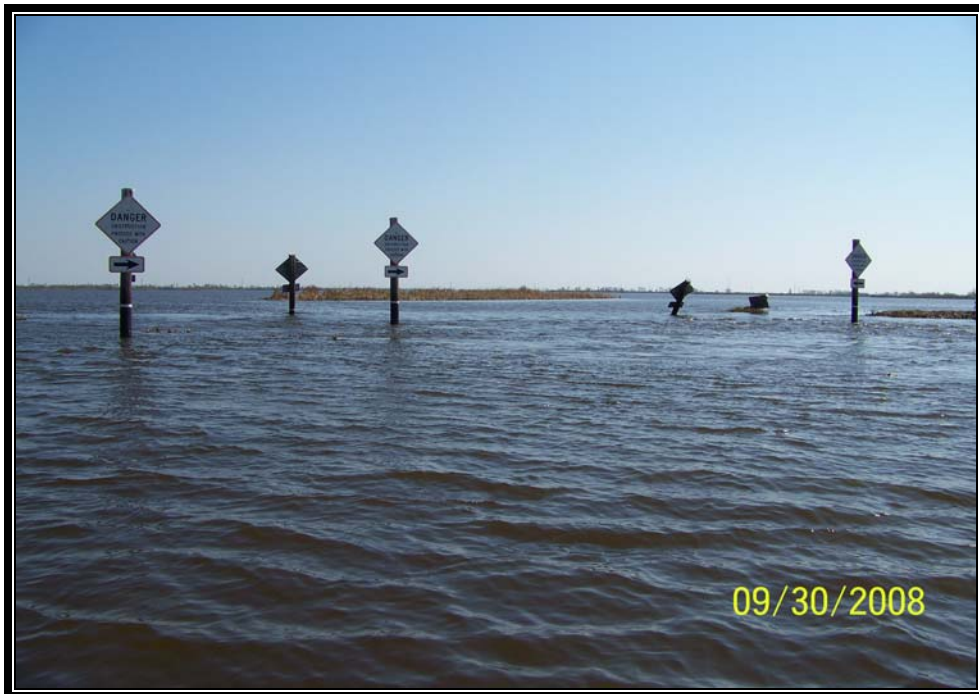
Photo No.12 – An overall view of the rock channel liner (Structure No.10) and existing warning signs.
