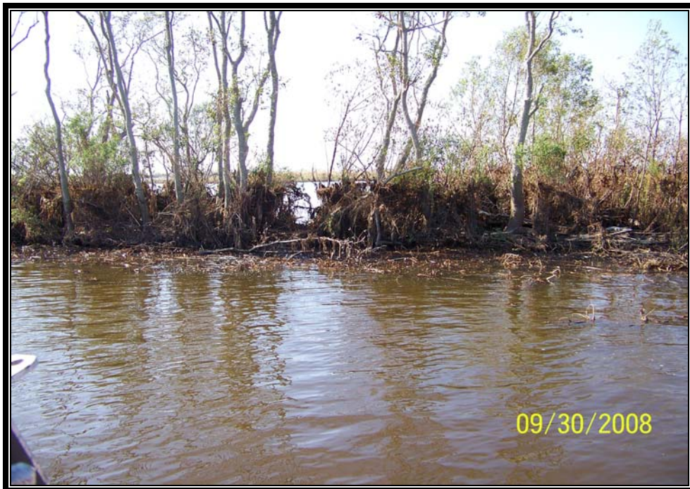
Photo No. 36 – Area along Superior Canal where the existing bank line is narrow and low.
