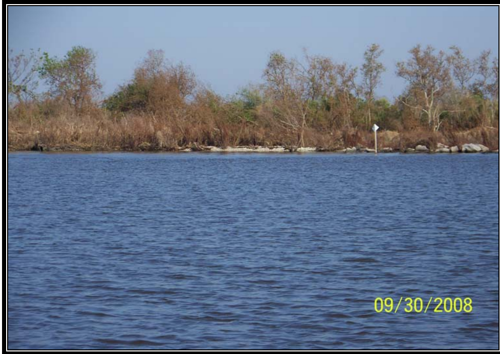
Photo No.31 – The very end of the rock dike along Bayou Decade near the mouth of Jug Lake.
