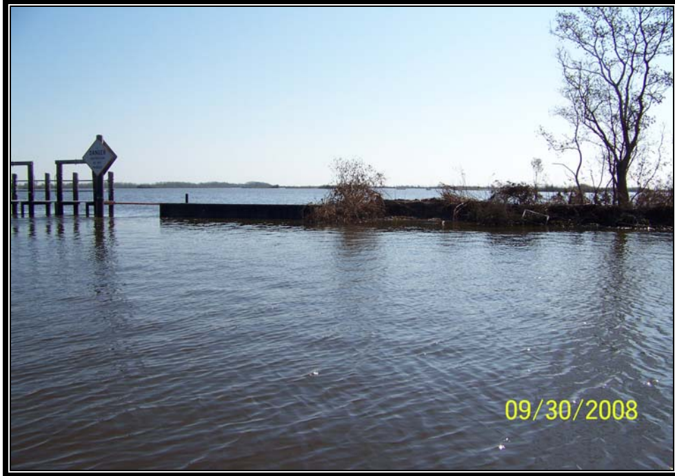
Photo No. 21 - View of the bulkhead tie-in to the earthen embankment on the south side of Structure No. 23.
