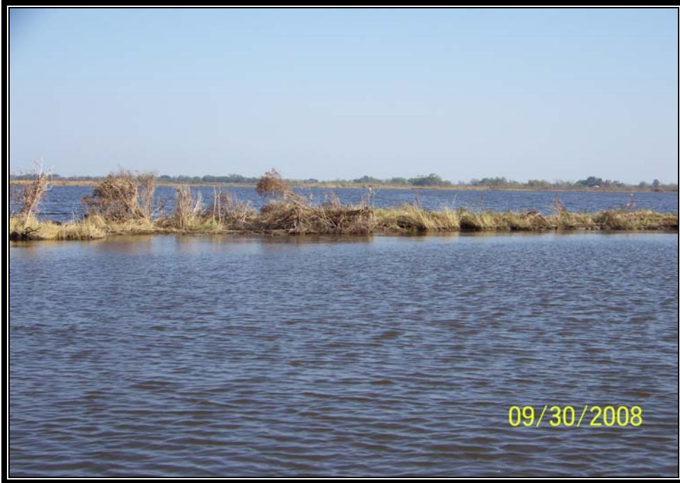
Photo No. 41 – Section of thin bank line along the north bank of Jug Lake between Structures 23 and 21.
