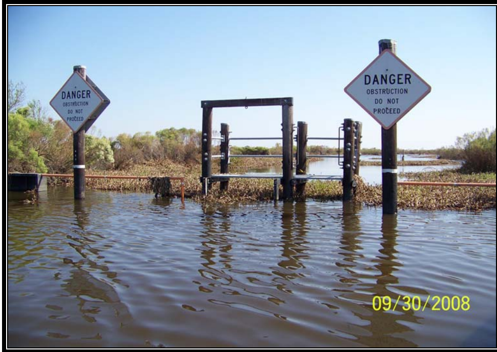
Photo No. 15 – View of the variable crested weir section at Structure 14 along Little Carencro Bayou.
