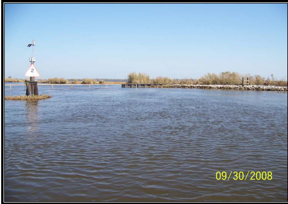
Photo No. 1 - View of timber navigation aid structure and steel bulkhead on the east side of the barge bay of Structure No.6 along Bayou Decade.
