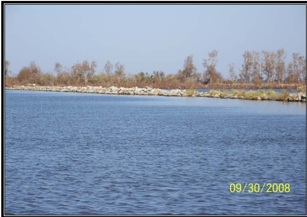
Photo No.30 – View of the rock dike along Bayou Decade near the mouth of Jug Lake.
