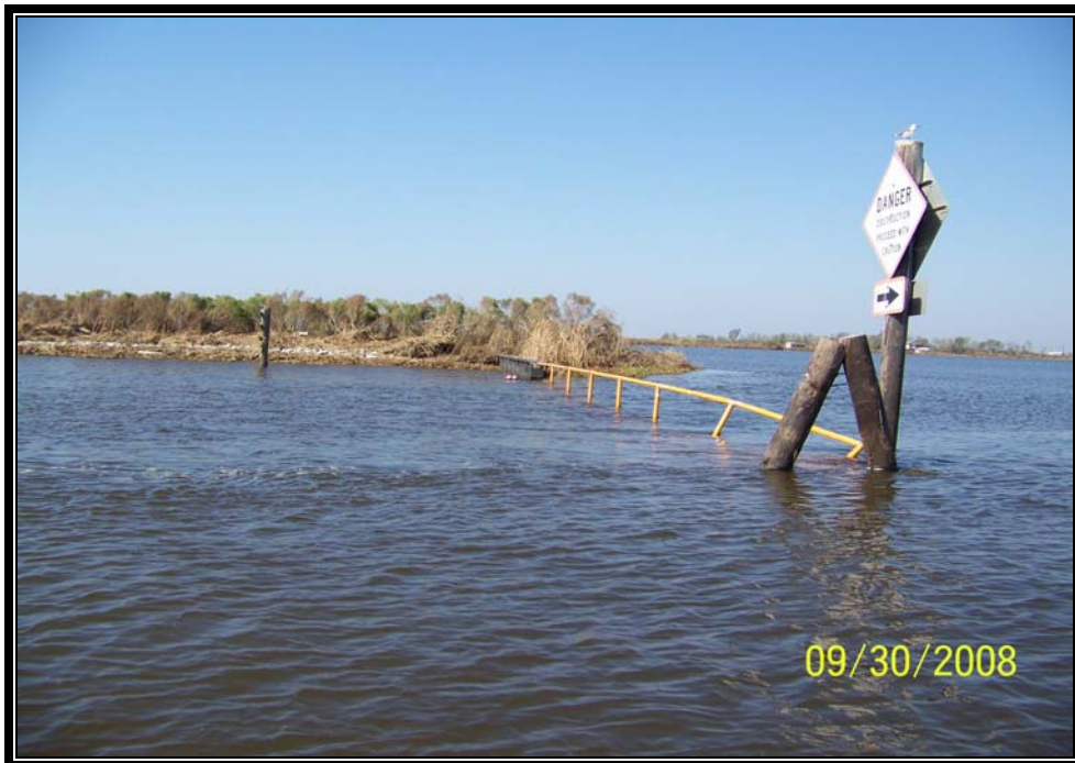
Photo No. 4 – View of the steel bulkhead and timber bumper guards on the west side of the barge bay of Structure No.6. The timber bumper guards were recently replaced by the oilfield service contractor at the request of the landowner.
