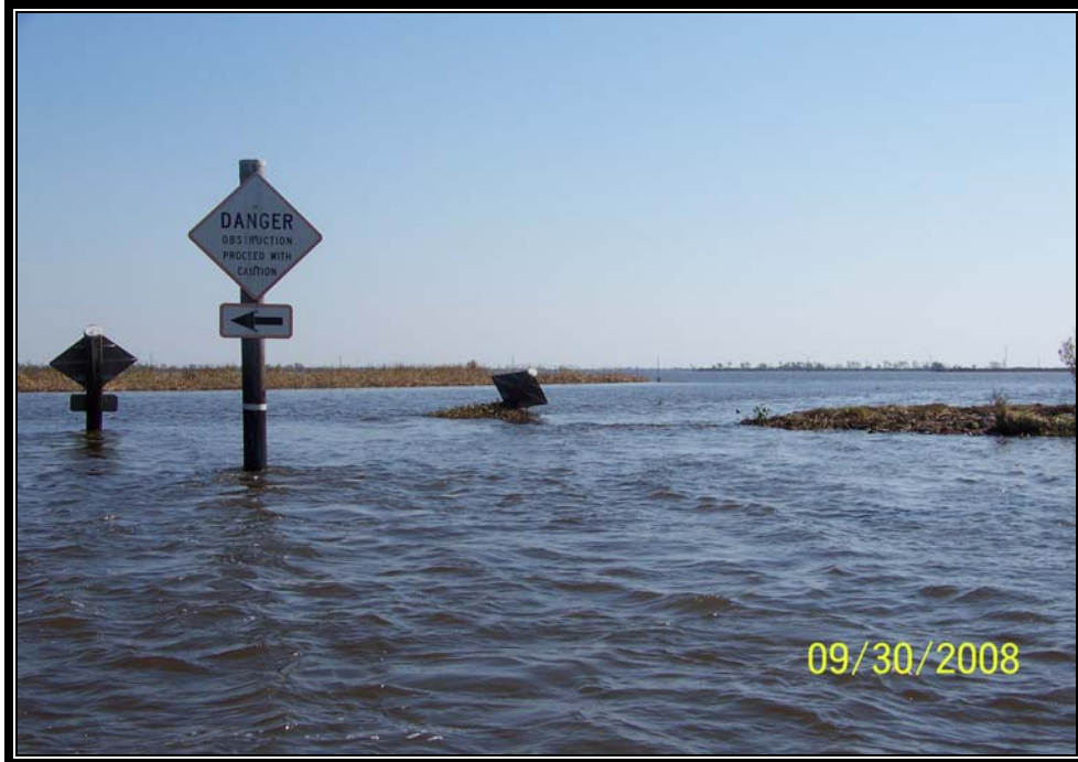
Photo No. 9 – A closer view of the damaged warning signs at Structure No.10 shown in the previous photo.
