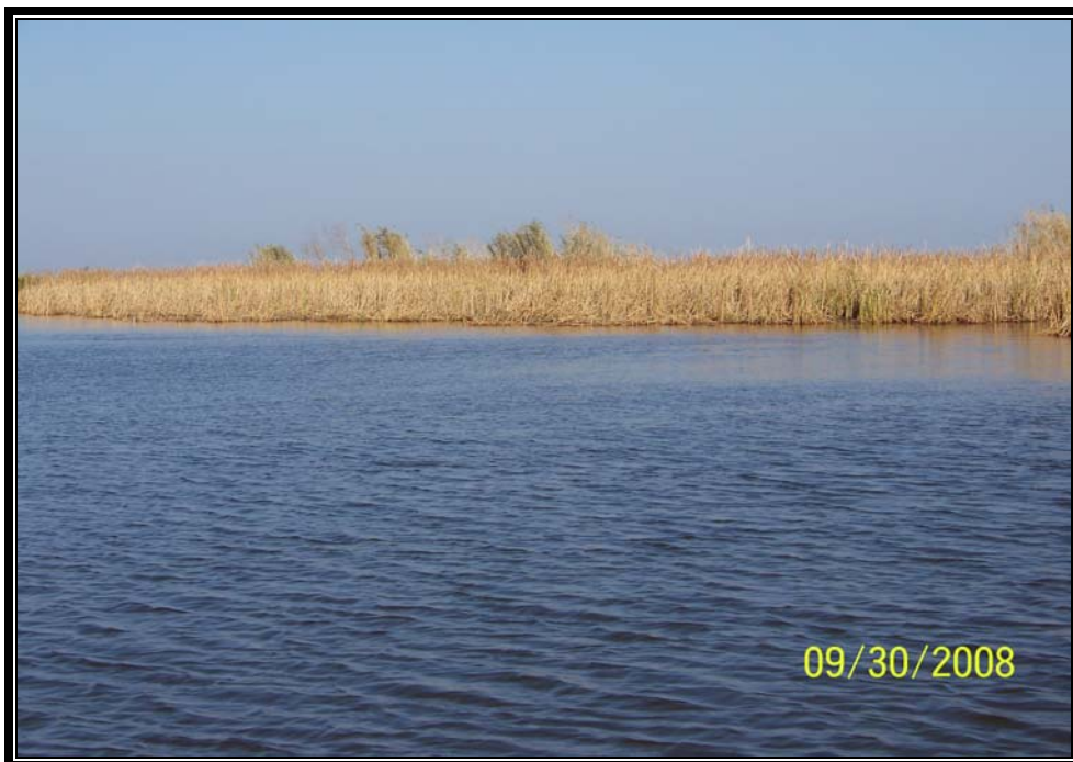
Photo No. 28 – Heavy concentration of cut grass in front of the rock dike along the north bank of Bayou Decade between Jug Lake and Turtle Bayou. This section of dike is concealed by the grass.
