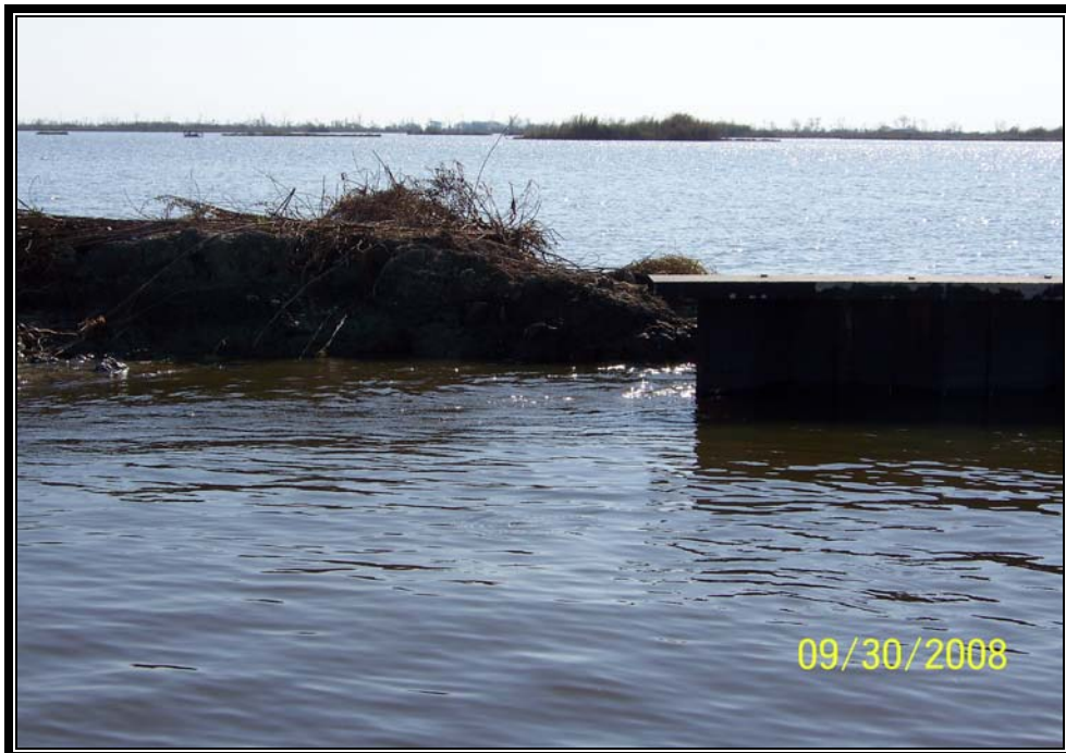
Photo No.24 – Another view of the breach around the north end of Structure No.23.
