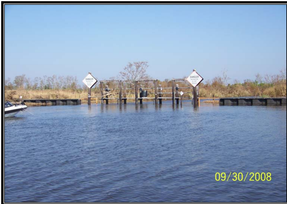
Photo No.20 – An overall view of the three (3) bay variable crest weir at Structure No.21.
