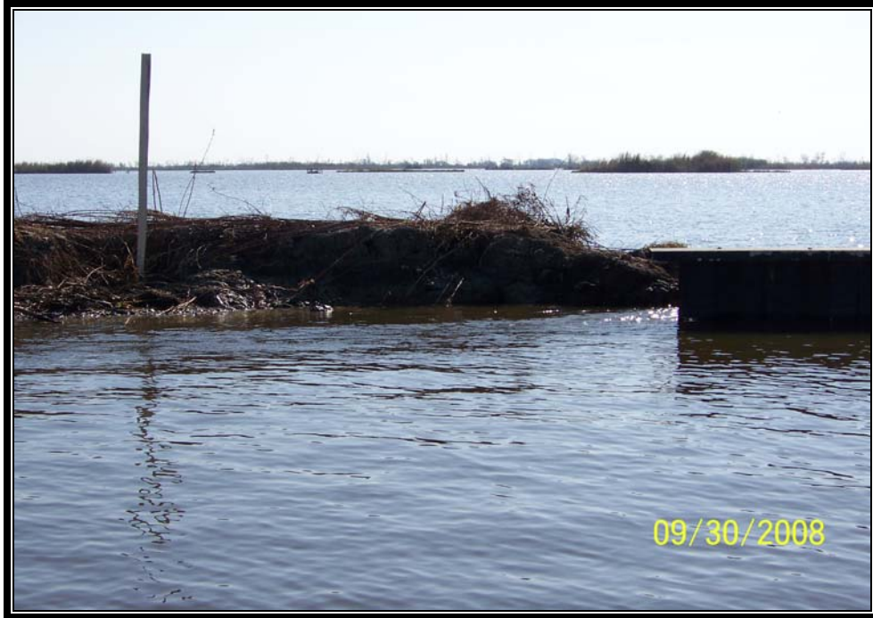
Photo No.23 – View of the northern end of the bulkhead of Structure No.23. The earthen embankment had eroded around the end of the bulkhead forming a breach.
