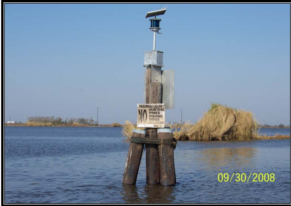
Photo No.5 – View of the timber navigational aid support and light on the northeast side of Structure No.6
