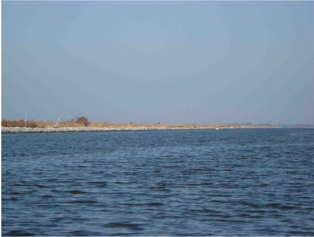
Photo #1 – Shoreline Protection Looking North.
