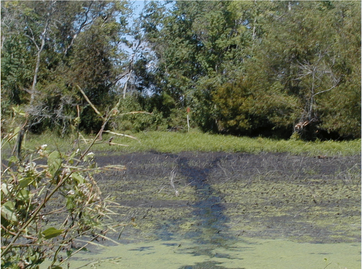
Figure 6. Photograph of the Cameron Prairie Refuge Protection (ME-09) project 6 years following construction in September 2000, showing shoreline advance between the rock breakwater and original shoreline at project station 11.
