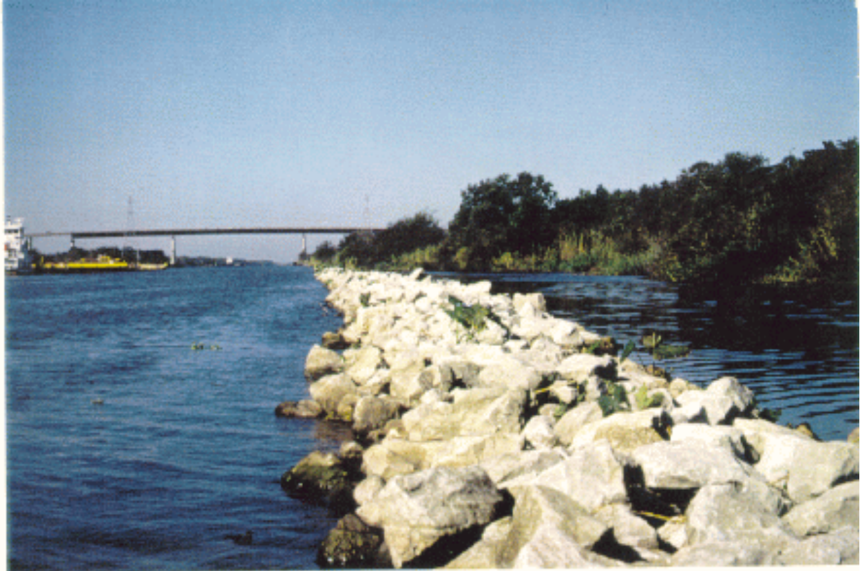
Figure 2. Photograph of the Cameron Prairie Refuge Protection (ME-09) project following construction in August 1994, illustrating the shoreline of the GIWW and the installed rock breakwater.
