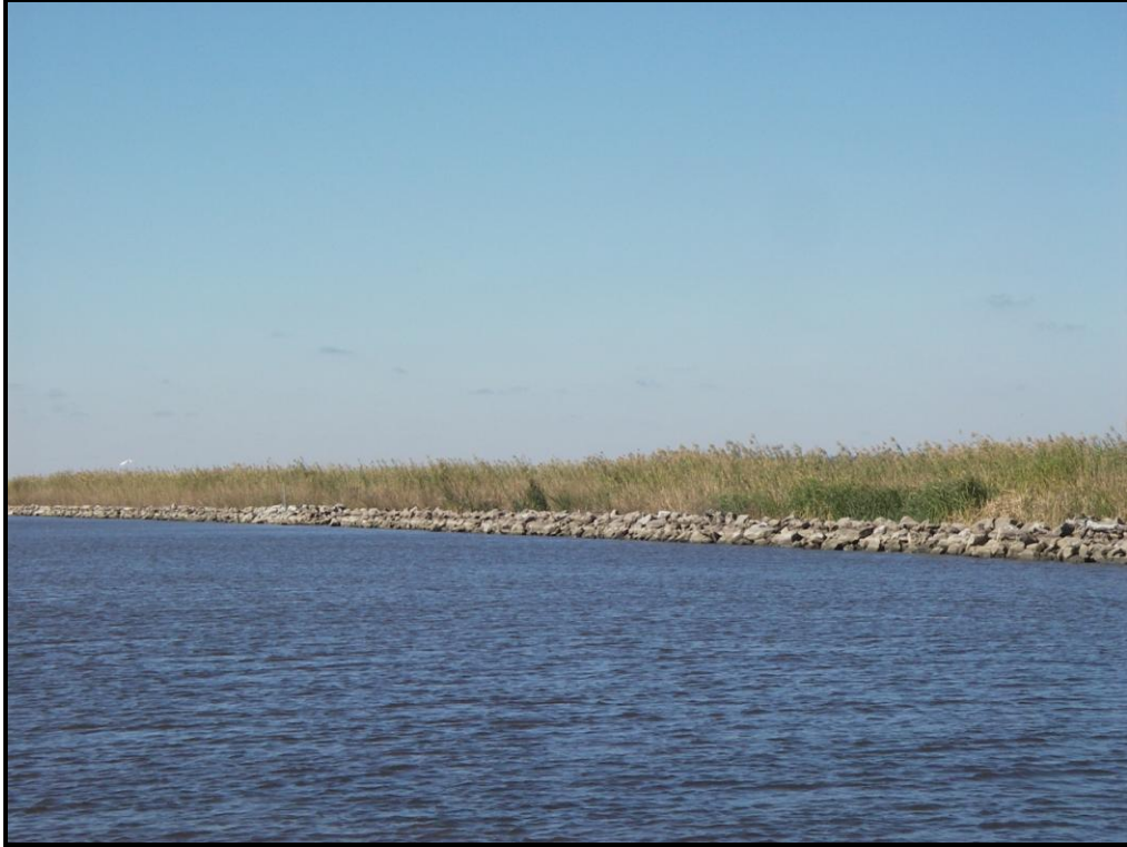
Photo 1 , Typical rock dike.
