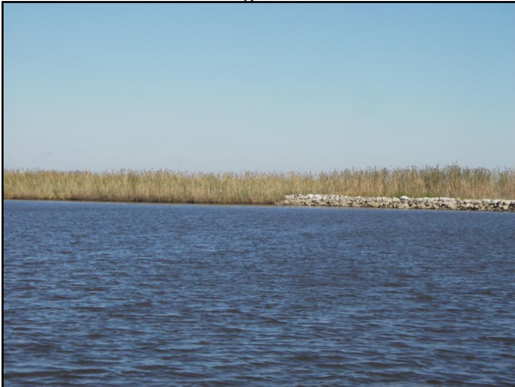
Photo 2 , Rock dike, view showing western tie-in to existing marsh.
