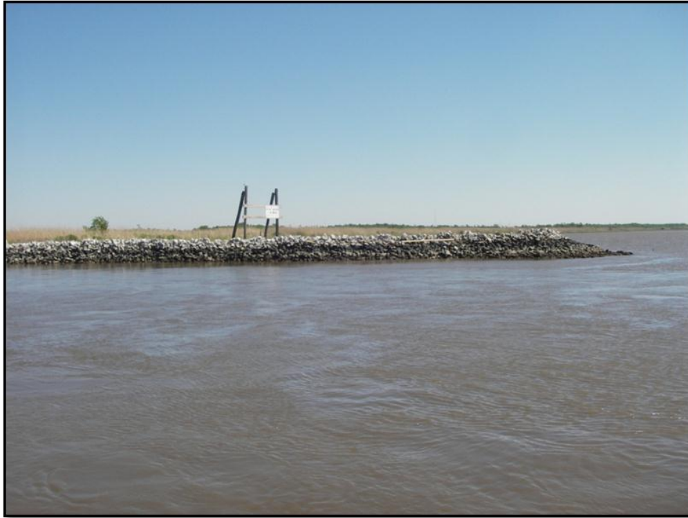
Photo No. 3 , Additional rock dike built by ChevronTexaco to protect existing pipelines, located and connected to rock dike on east side of Oaks Canal
