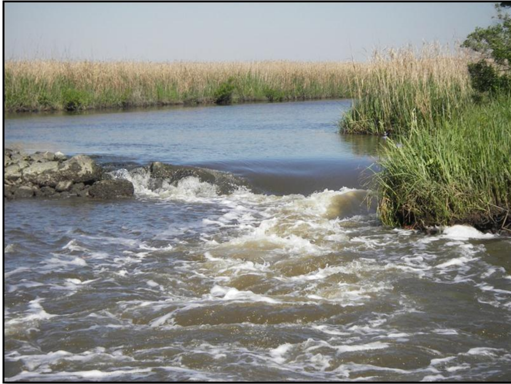
Photo No. 5, The difference in head between the adjacent water bodies forcing water through the breach in the rock plug.
