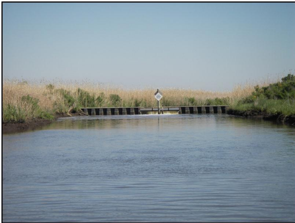
Photo No. 4 , Cow Path Structure
