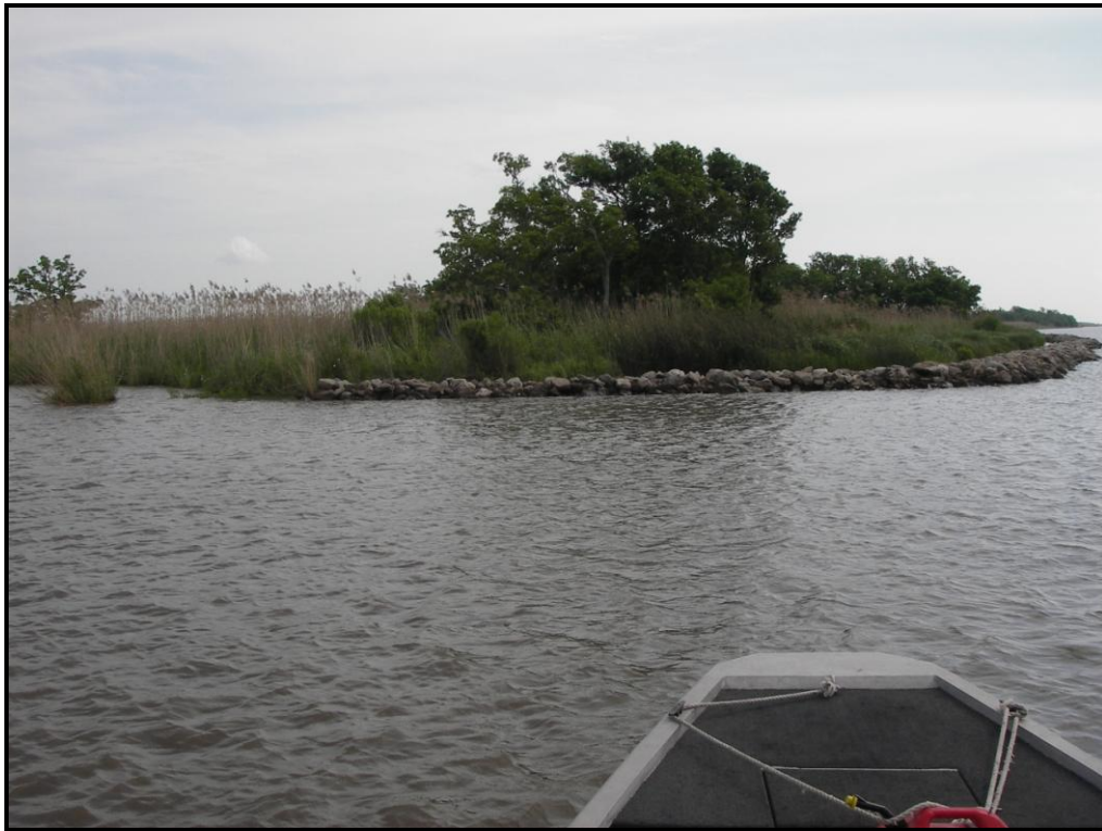
Photo 1 — rock dike on north bank of GIWW; west tie in
