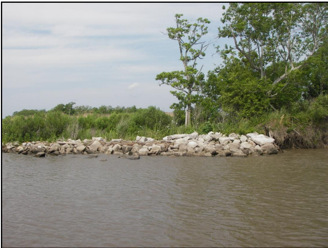
Photo 3-- rock dike on north bank of GIWW; east tie in
