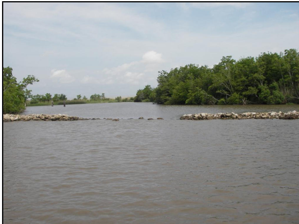
Photo 2 —settled rock on north bank of GIWW at barge slip
