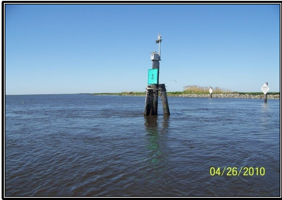
Photo No.25 – view the timber dolphin support and navigational aid on the southeast side of the barge bay at Structure 14A.
