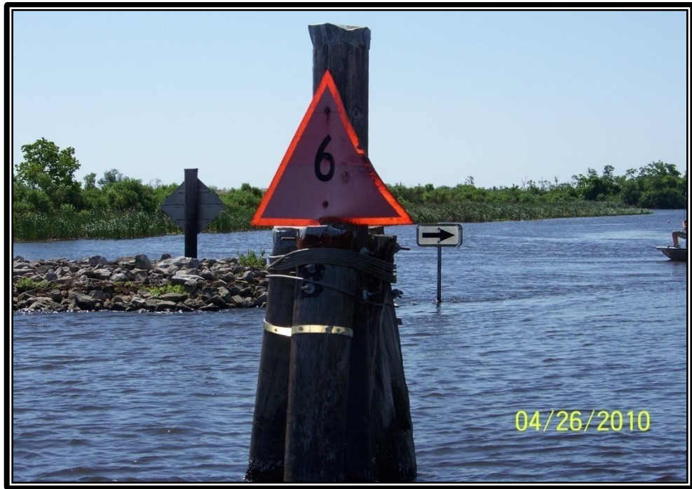
Photo No.15 – view of timber pile dolphin on the northeast side of the barge bay entrance of Structure No.1.
