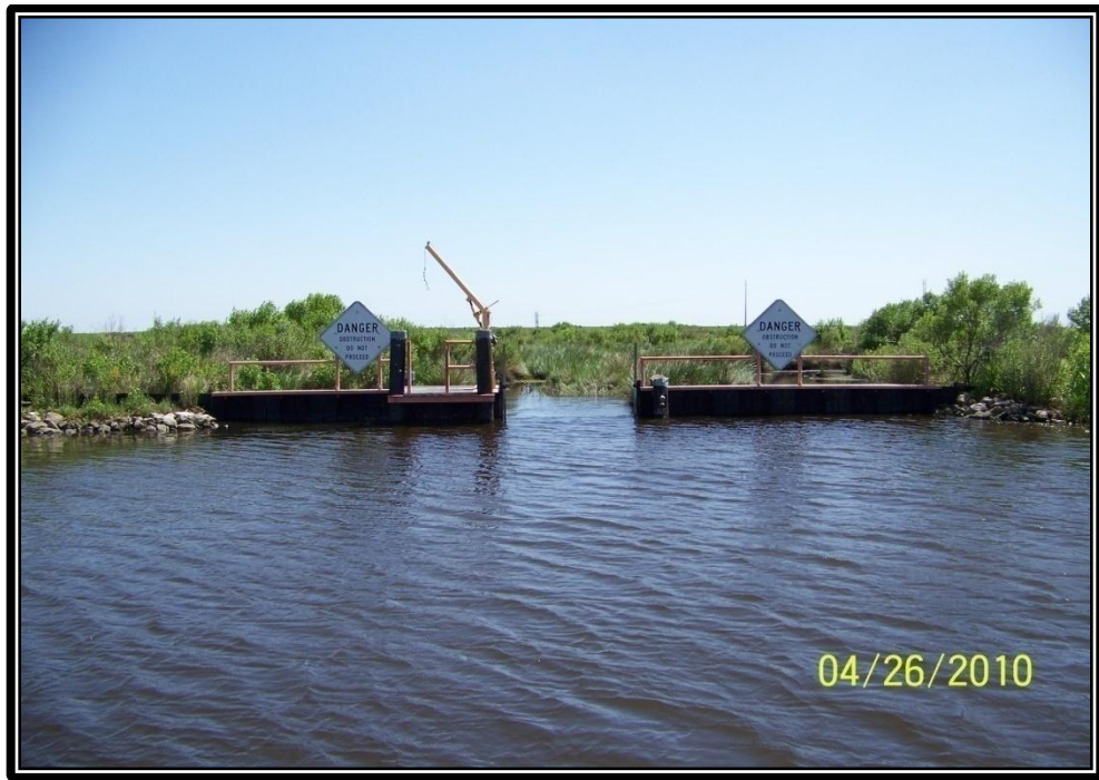
Photo No.36– view of variable crest weir Structure No.35 along north bank of location canal on the east side of Breton Canal.
