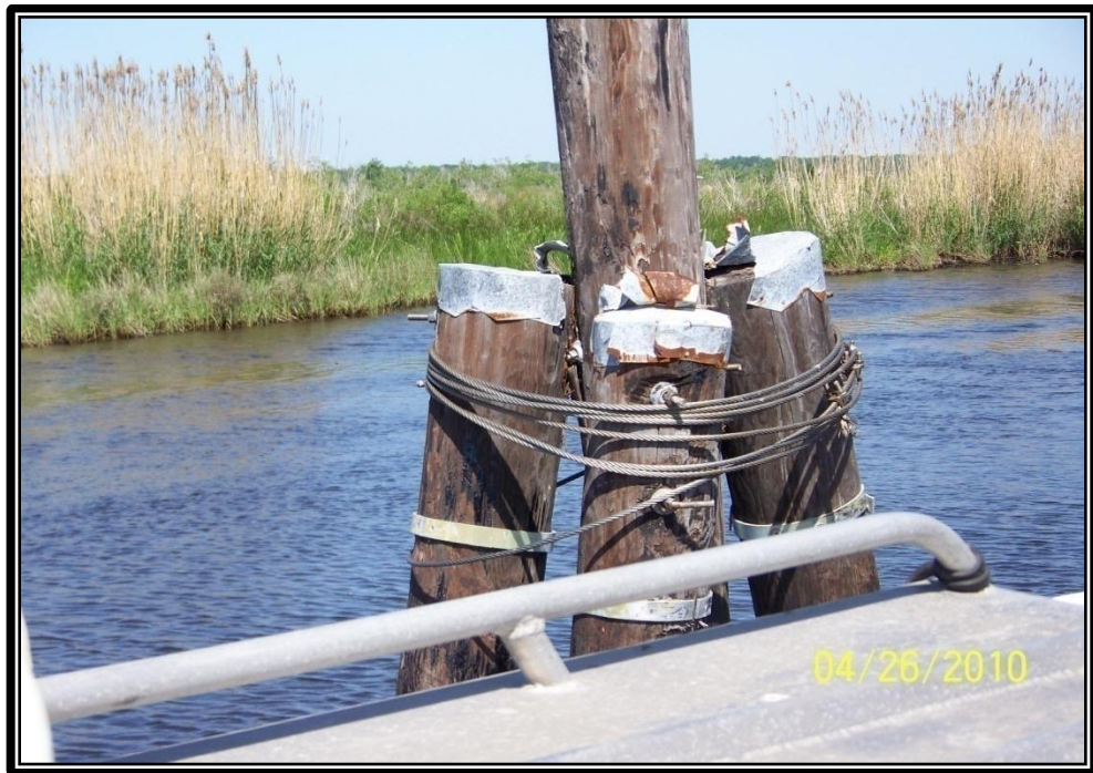
Photo No. 16 – another view of damaged timber dolphin structure at the barge bay entrance of Structure No.1.
