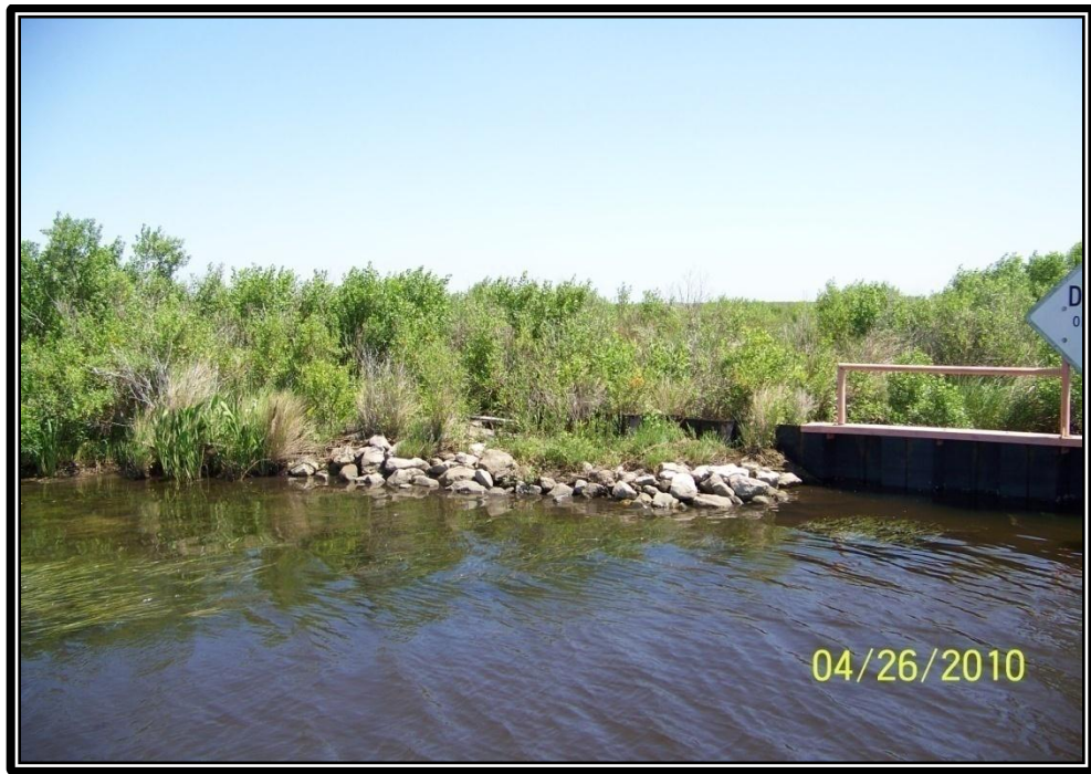
Photo No.38 – view of steel bulkhead and bank tie-in on the north side of Structure No.35.
