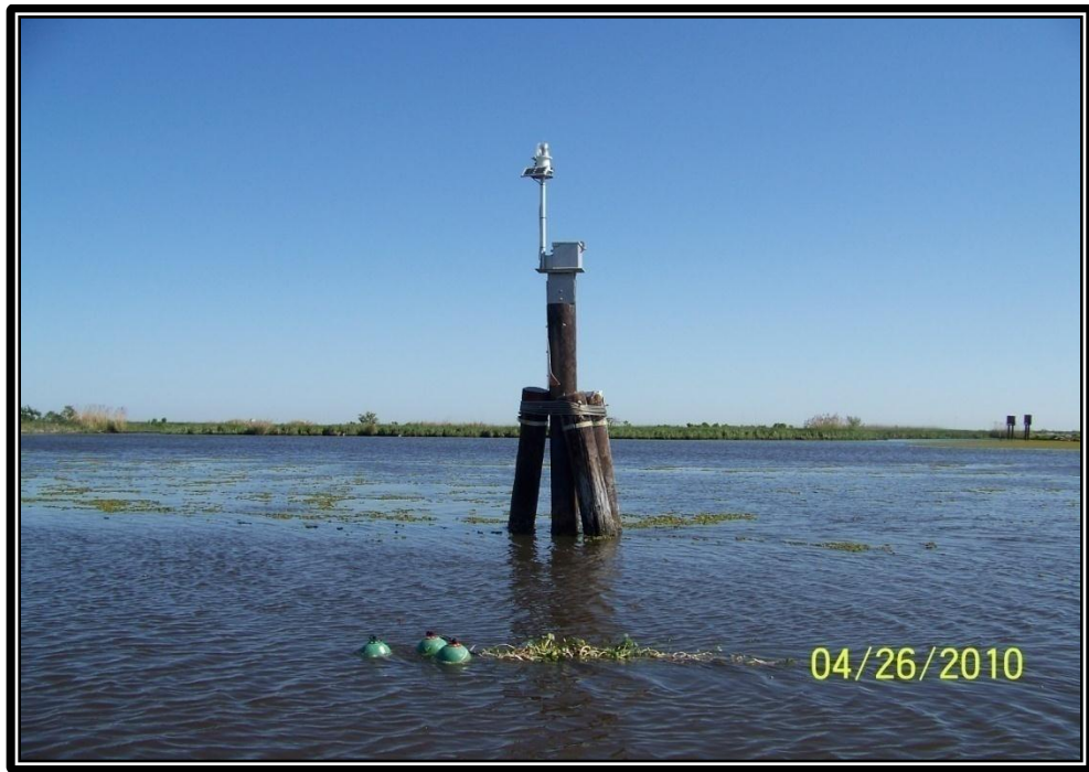
Photo No.22 – view of timber dolphin support structure and navigational aid on the northwest side of Structure No. 14A.
