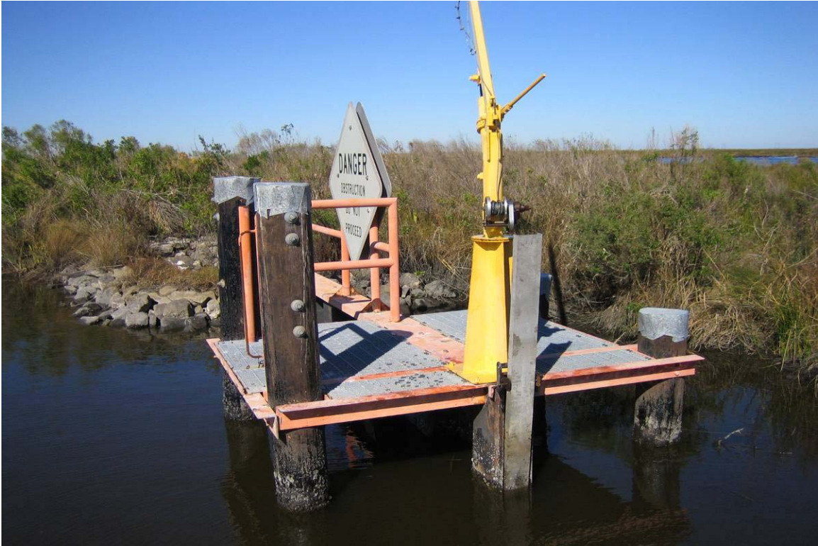
North Side Structure Condition (11-25-08)
