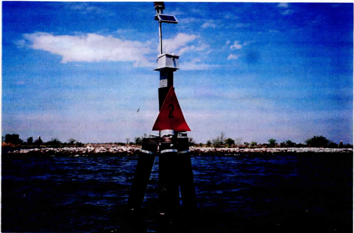
Photo 2 – Navigation Light No. 2 (Site 14a).
