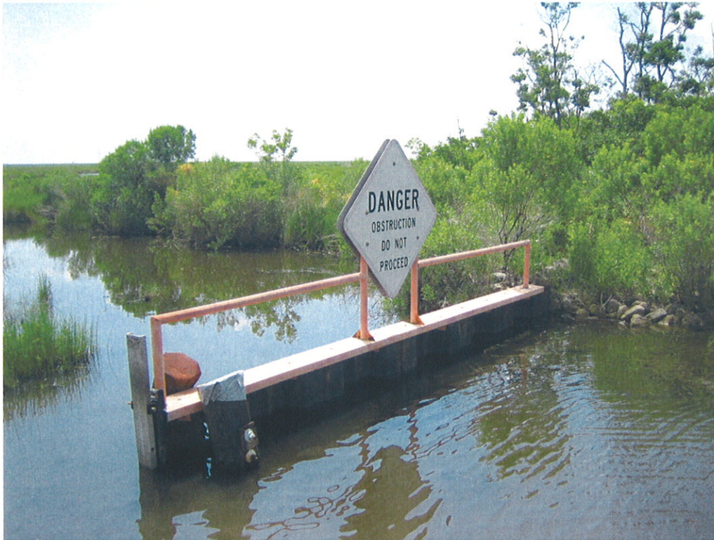
South Side Structure Condition (05-14-09)
