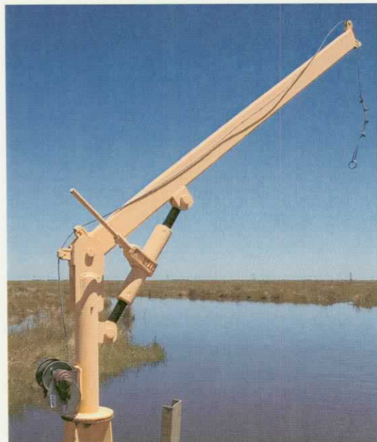
Crane, Winch & Hoist Condition (4/12/05)
