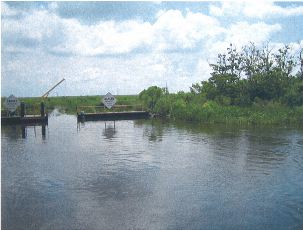
Overall Structure Condition (05-14-09)
