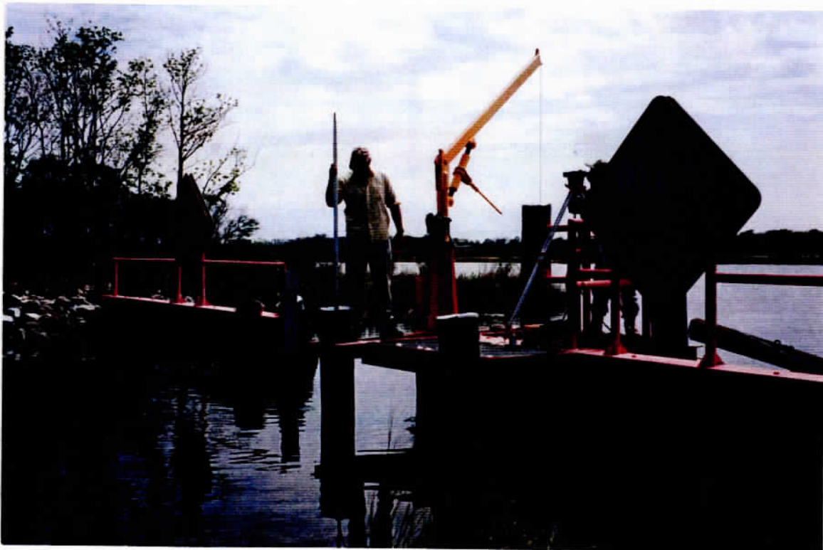
Photo 10 – Variable Crest Weir (Site 35), view of control survey in progress
