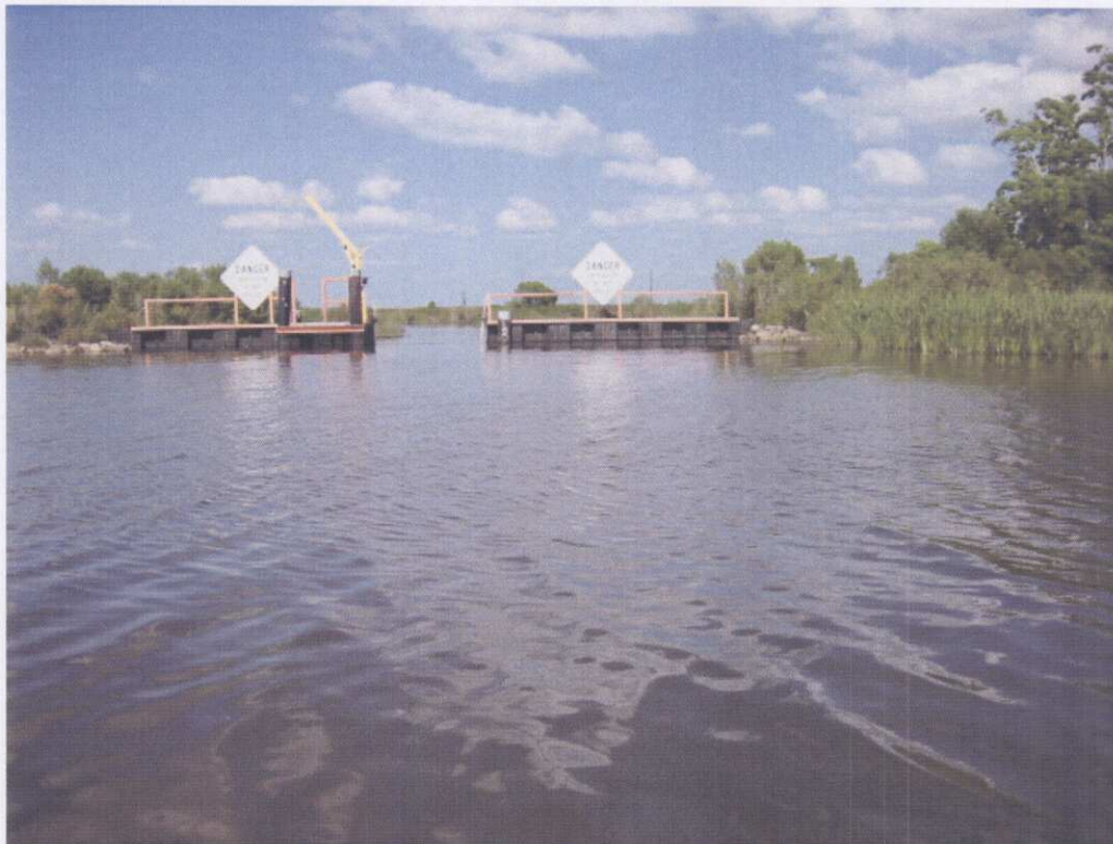
Overall Structure Condition (4-30-08)
