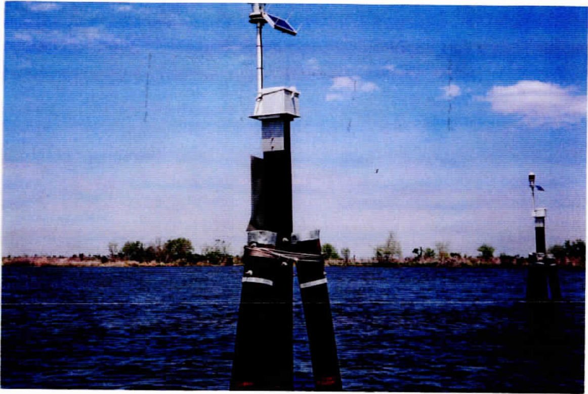
Photo 1 – Navigation Light No. 1 (Site 14a).
