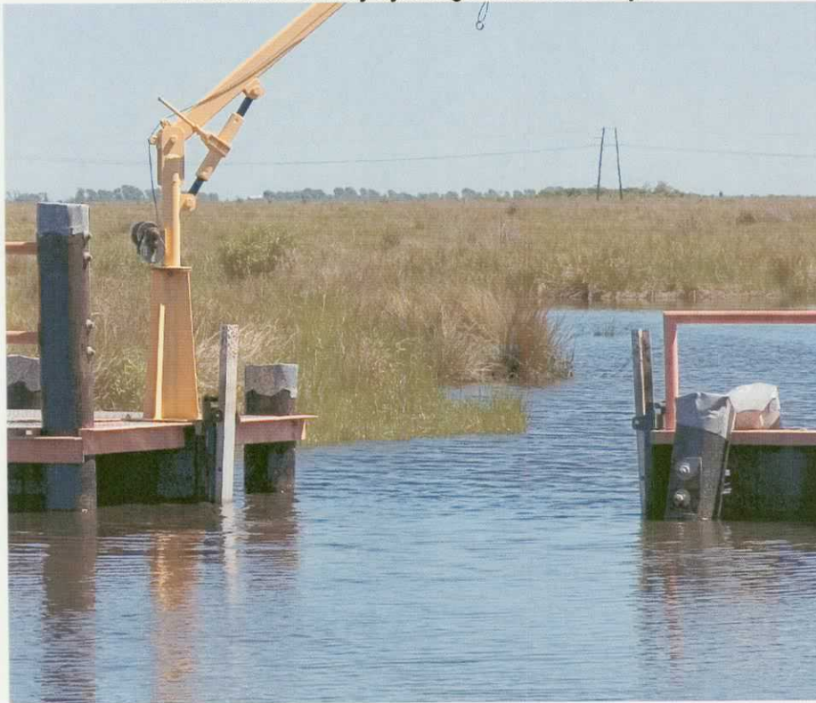
Pre Stop Log Installation (4/12/05)
