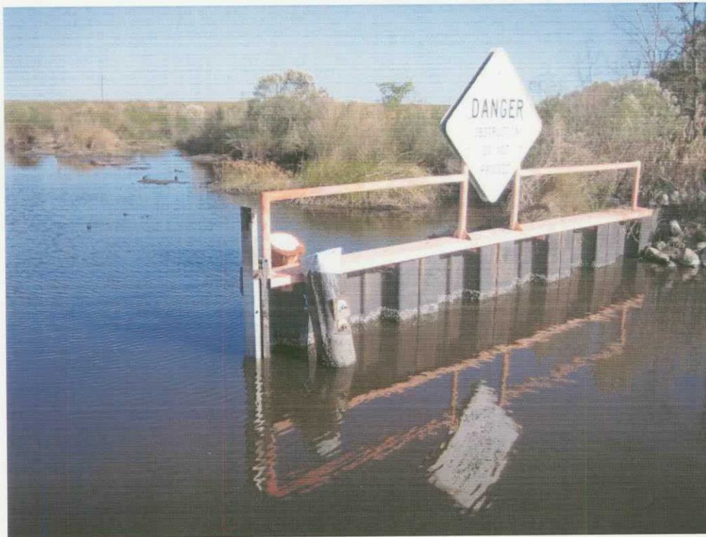
South Side Structure Condition (11-8-07)
