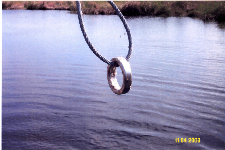
BA-02 Missing Eye Hook on End Lifting Cable
