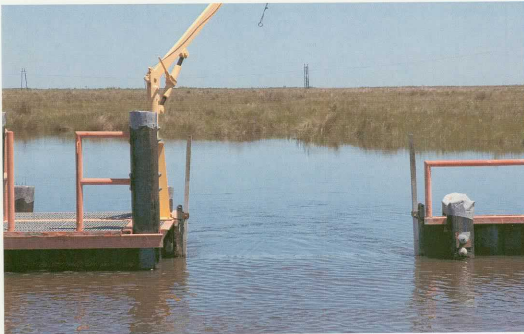
Post Stop Log Installation (4/12/05)
