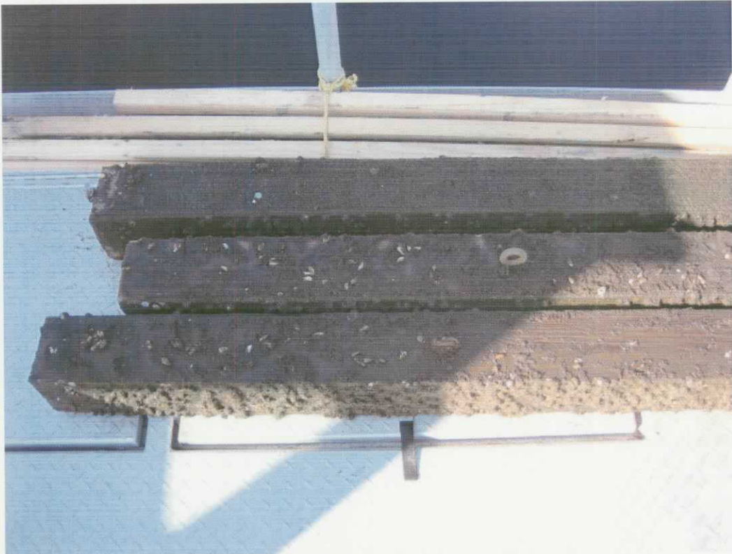
Stop Log Condition Post-removal (11-8-07)
