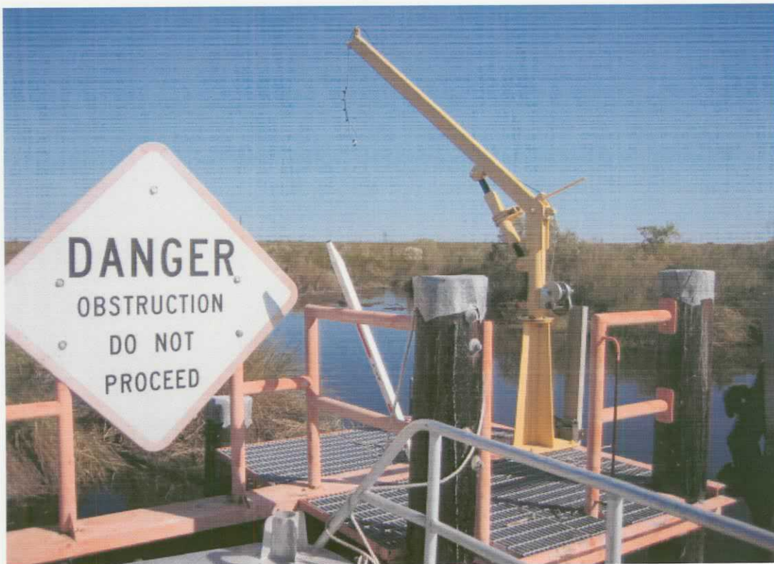
Structure Condition: Winch, Crane, Hoist, and Pile Caps (11-8-07)
