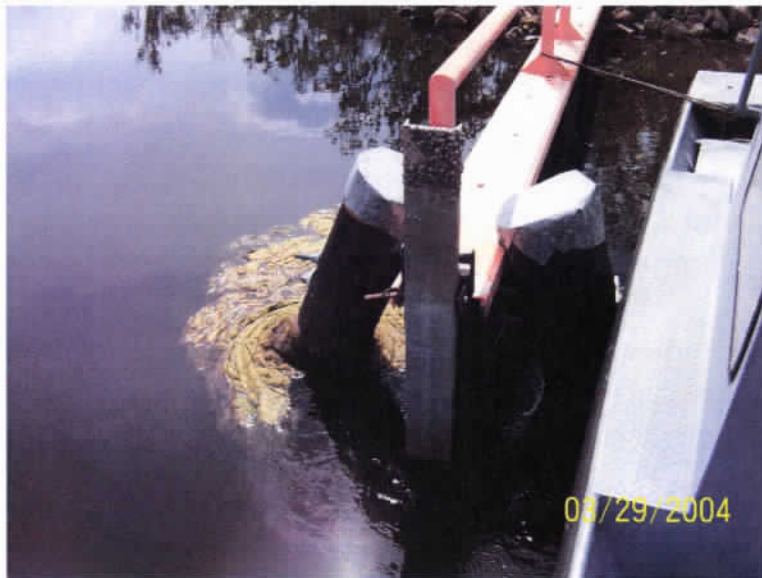
Pre Stop Log Installation with Old Lock and Bent Lock Pin
