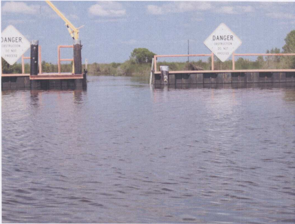
Overall Structure Condition (4-30-08)
