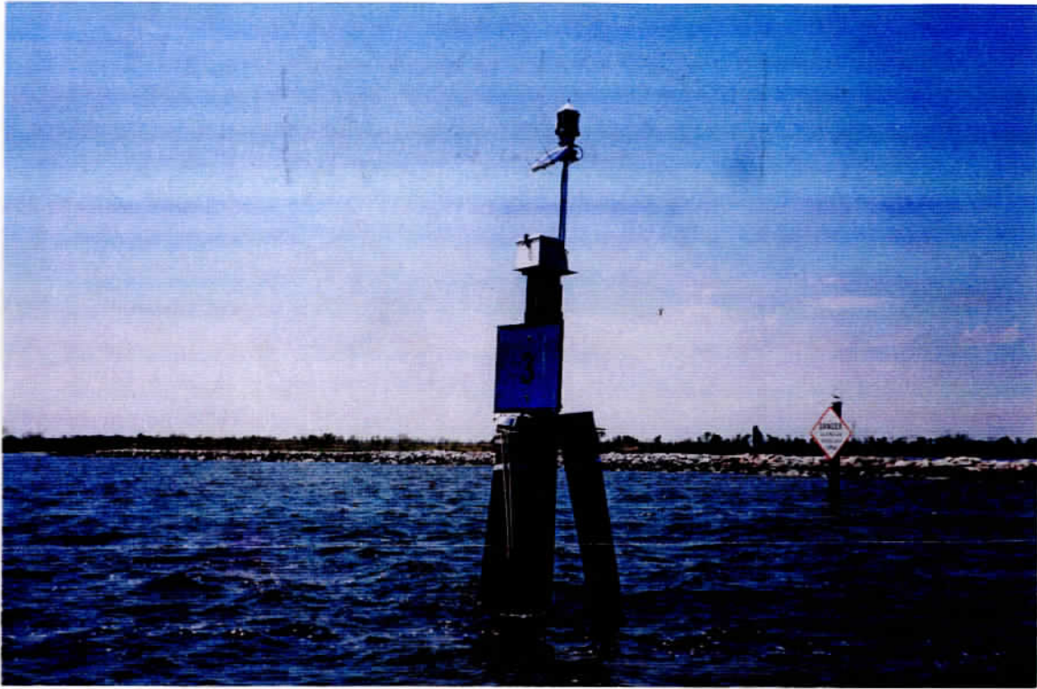
Photo 3 – Navigation Light No. 3 (Site 14a).
