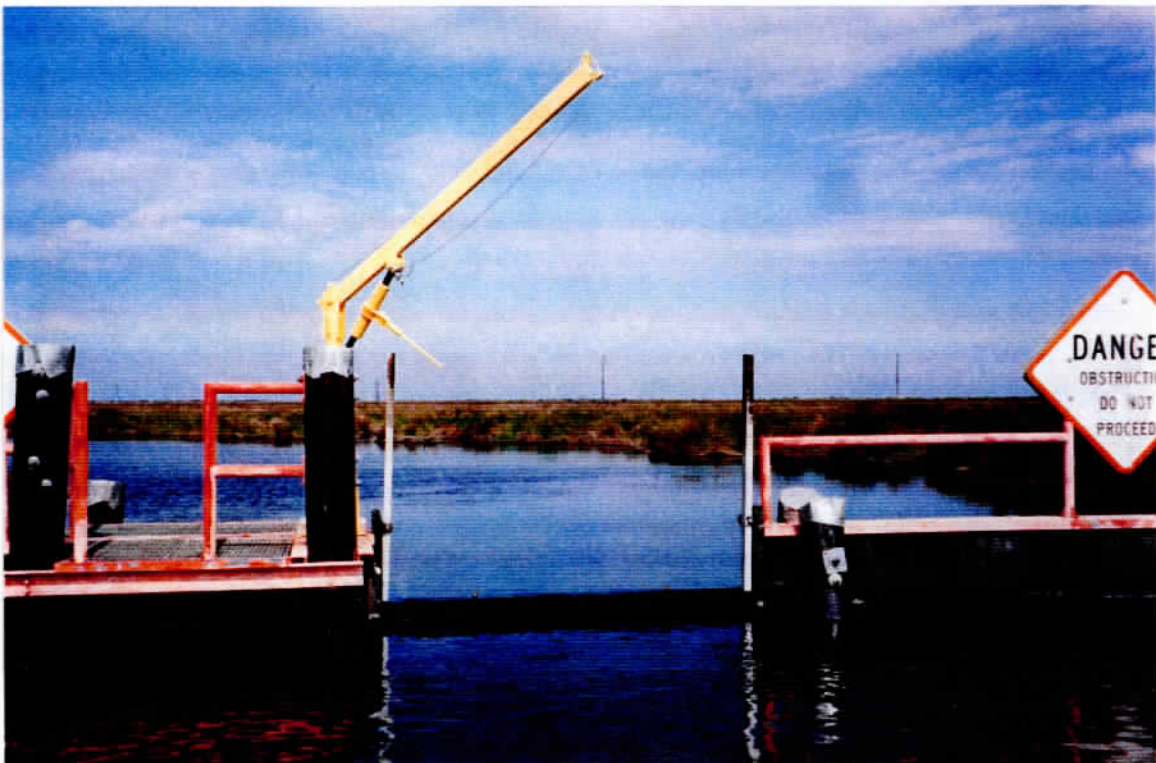
Photo 16 – Variable Crest Weir (Site 35), looking east at the temporarily secured weir structure.
