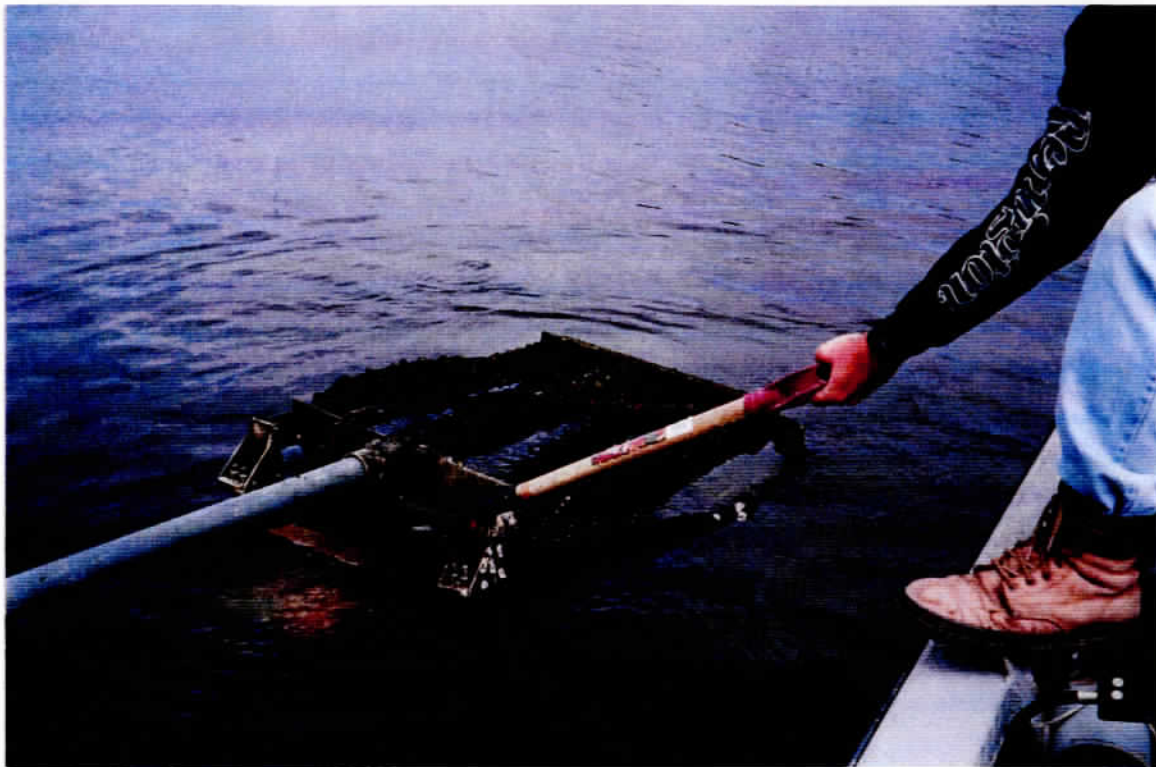
Photo 6 – Operating the Flapgated Culvert Structure (Site 91) and scraping barnacles off the flapgate hinge system.
