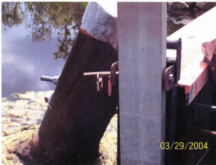
Post Stop Log Installation with New Lock
