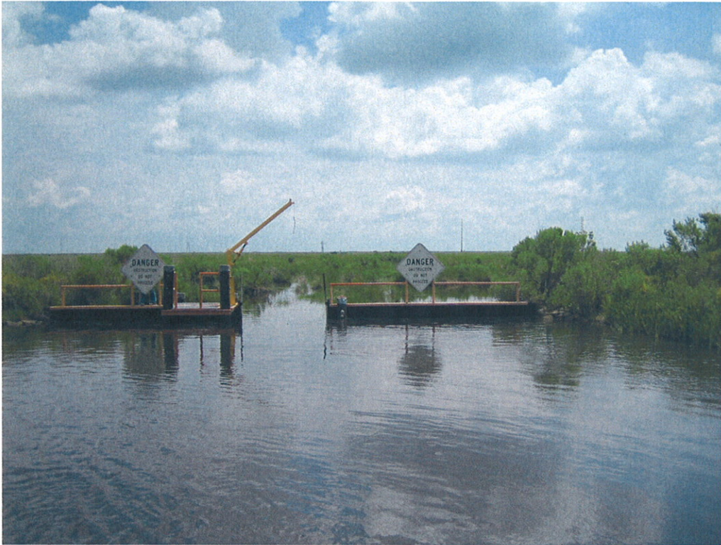
Overall Structure Condition (05-14-09)
