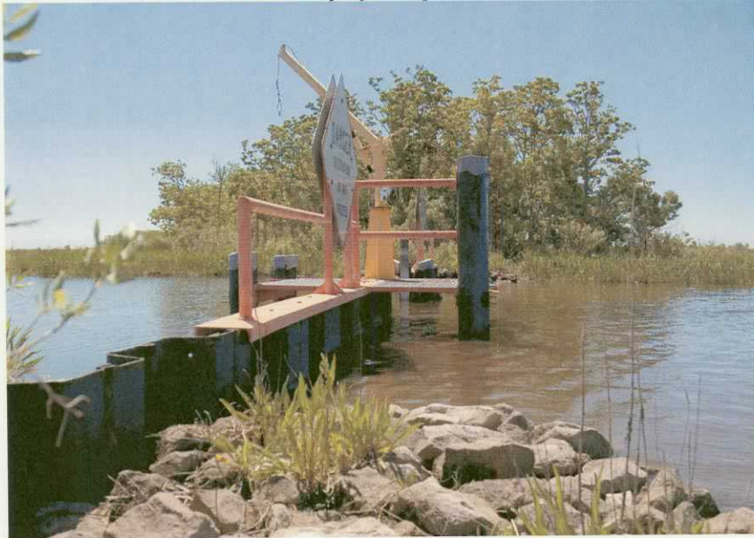
Water Control Structure Condition (4/12/05)
