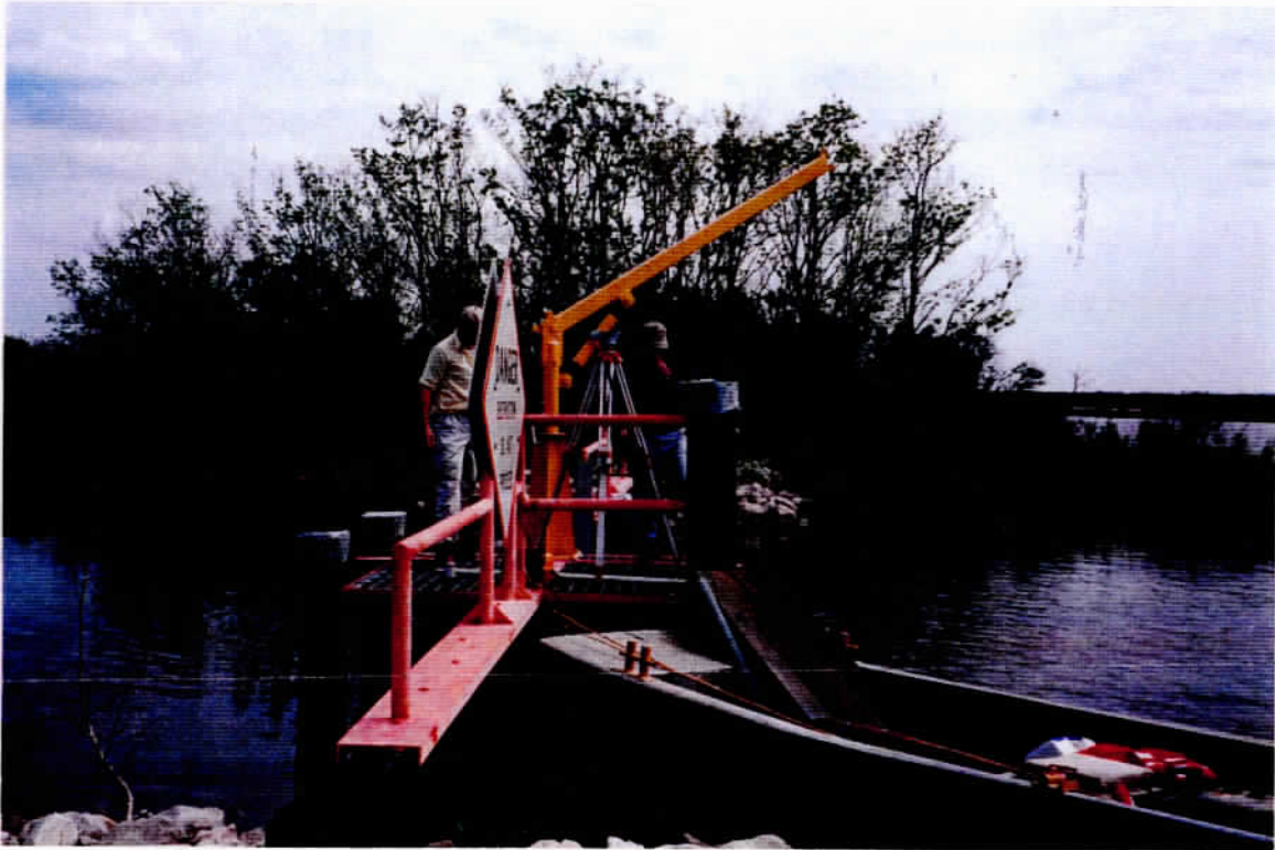
Photo 9 – Variable Crest Weir (Site 35), side view of weir structure and lifting boom.
