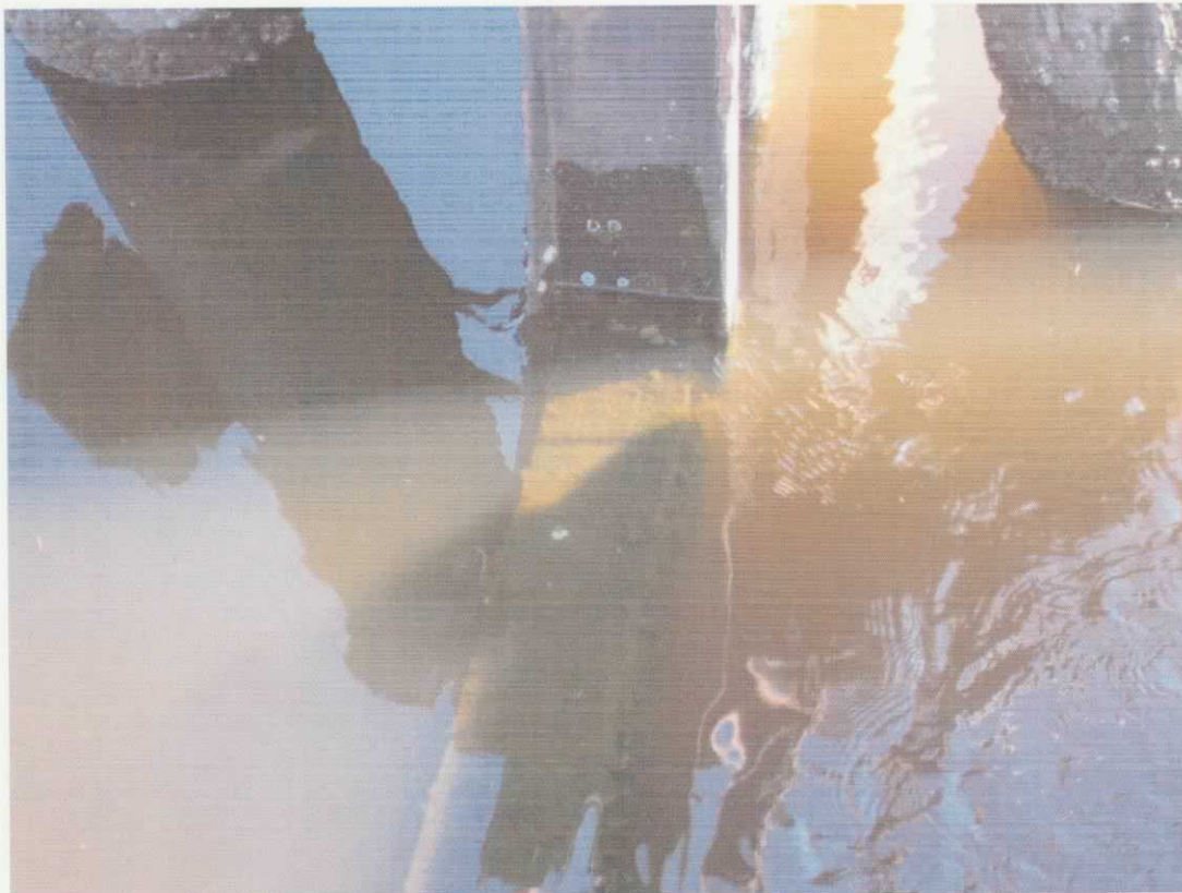
Condition of Stop Logs Pre-removal (11-8-07)
