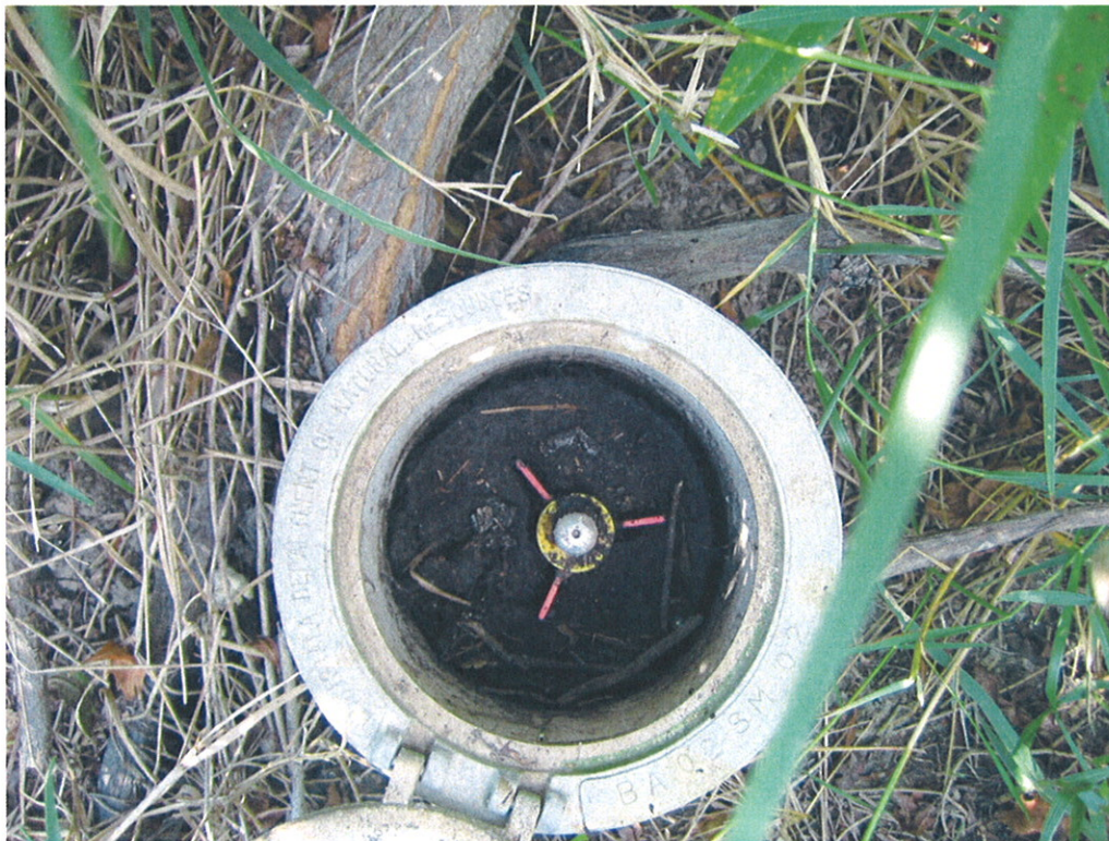
Benchmark Overall Condition (05-14-09)
