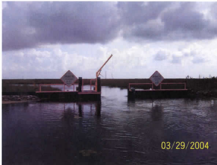
Pre Stop Log Installation
