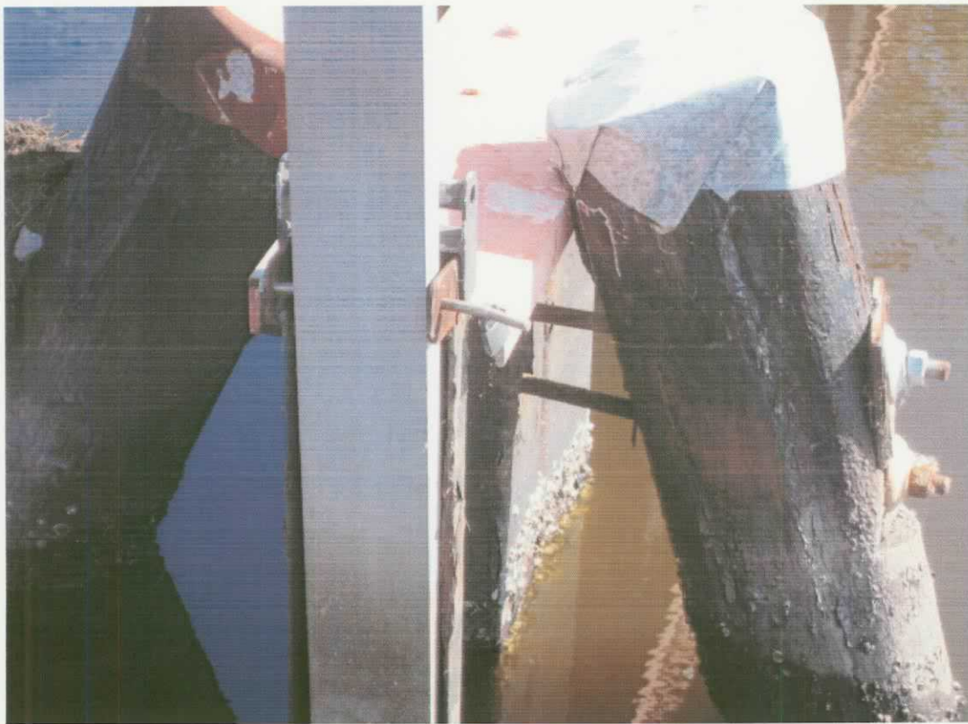
Bent Pin and Pile Cap (11-8-07)
