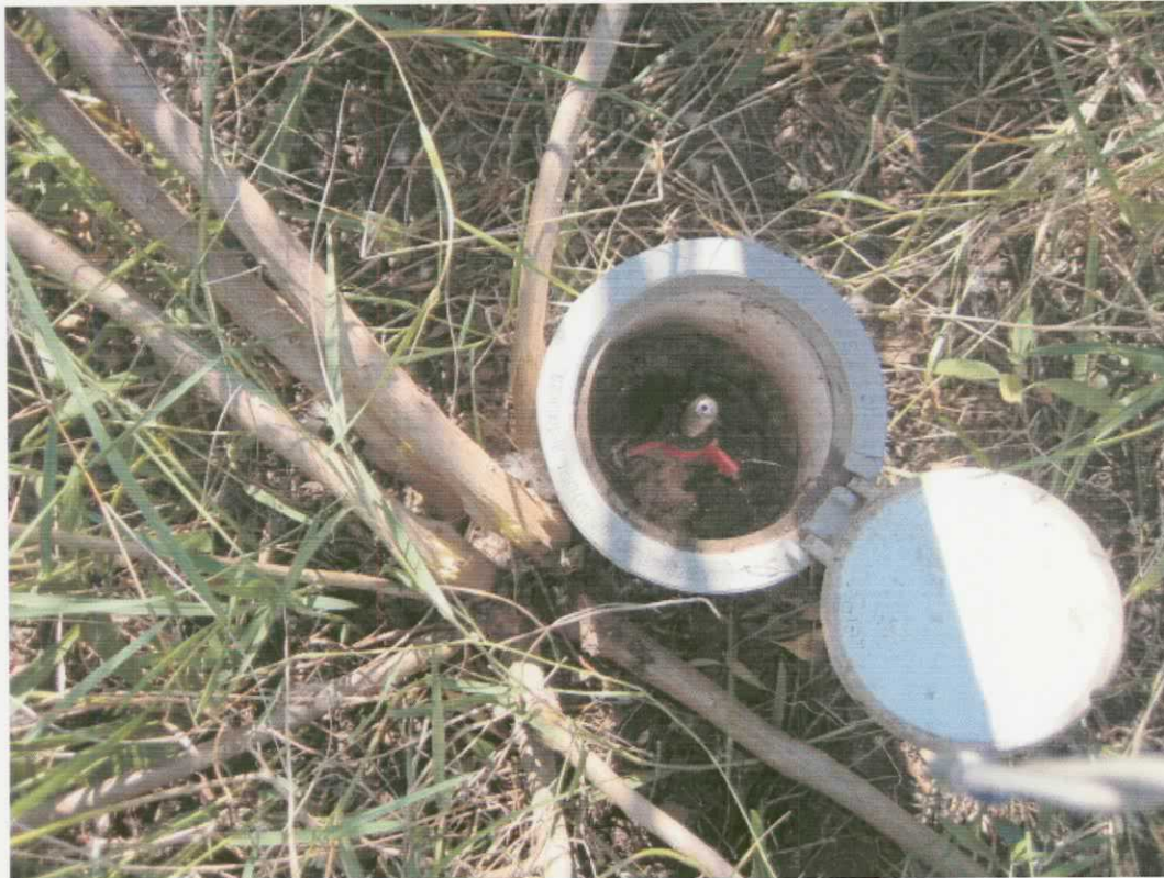
Benchmark Overall Condition (11-8-07)
