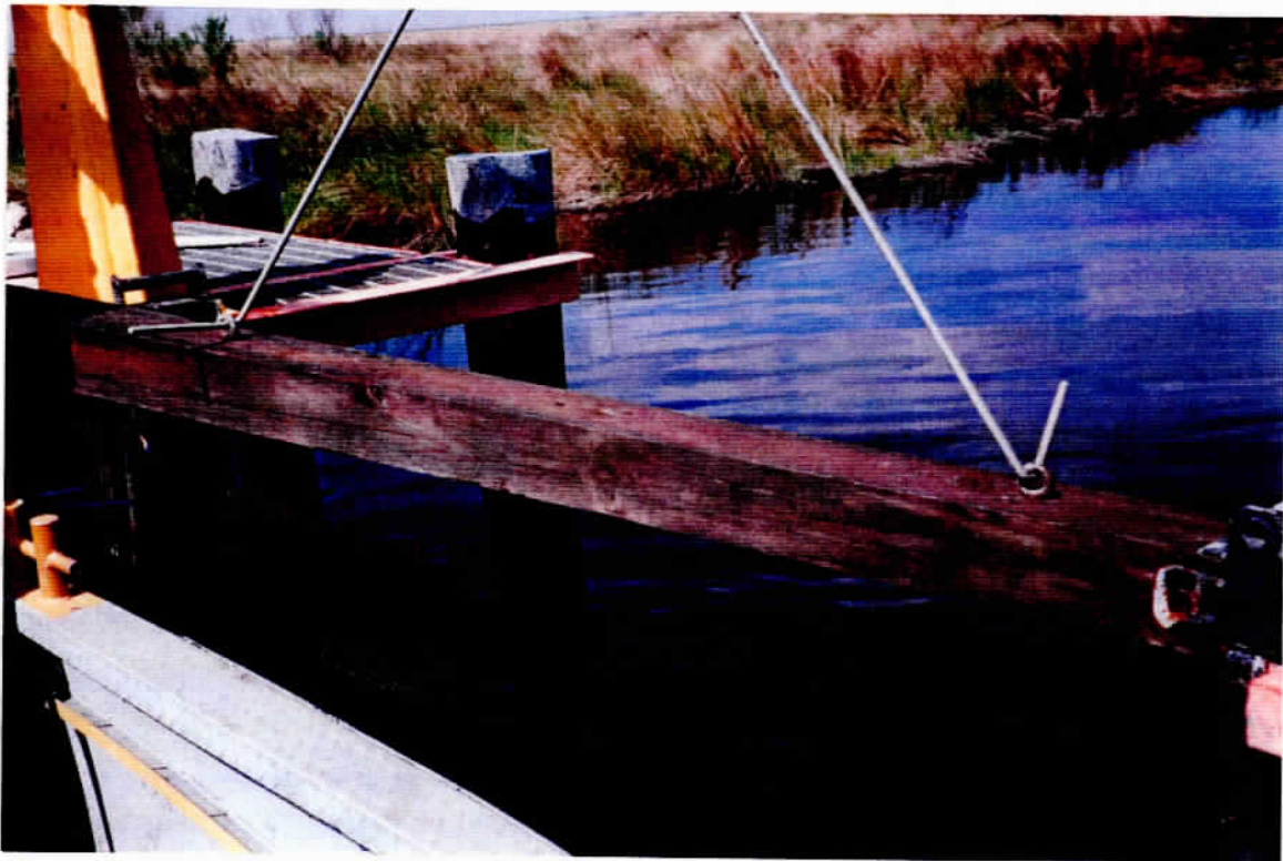
Photo 14 – Variable Crest Weir (Site 35), view of stoplogs being installed.
