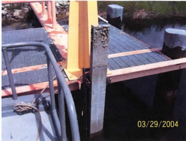
Pre Stop Log Installation with Old Lock and Slightly Bent Lock Pin
