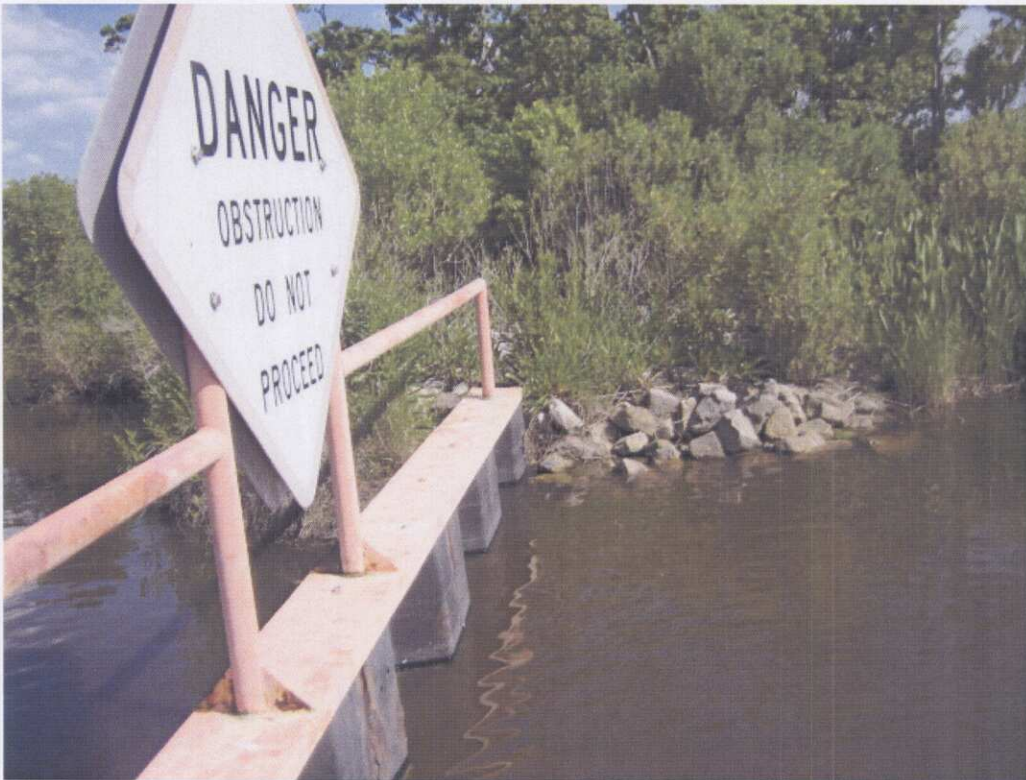
South Side Structure Condition (4-30-08)
