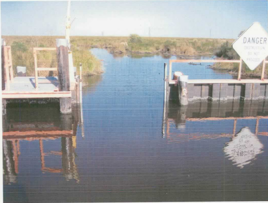
Overall Structure Condition (11-8-07)
