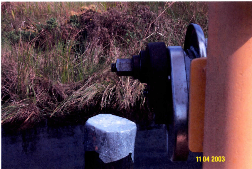
BA-02 Missing Crank Handle on Crane Hoist
