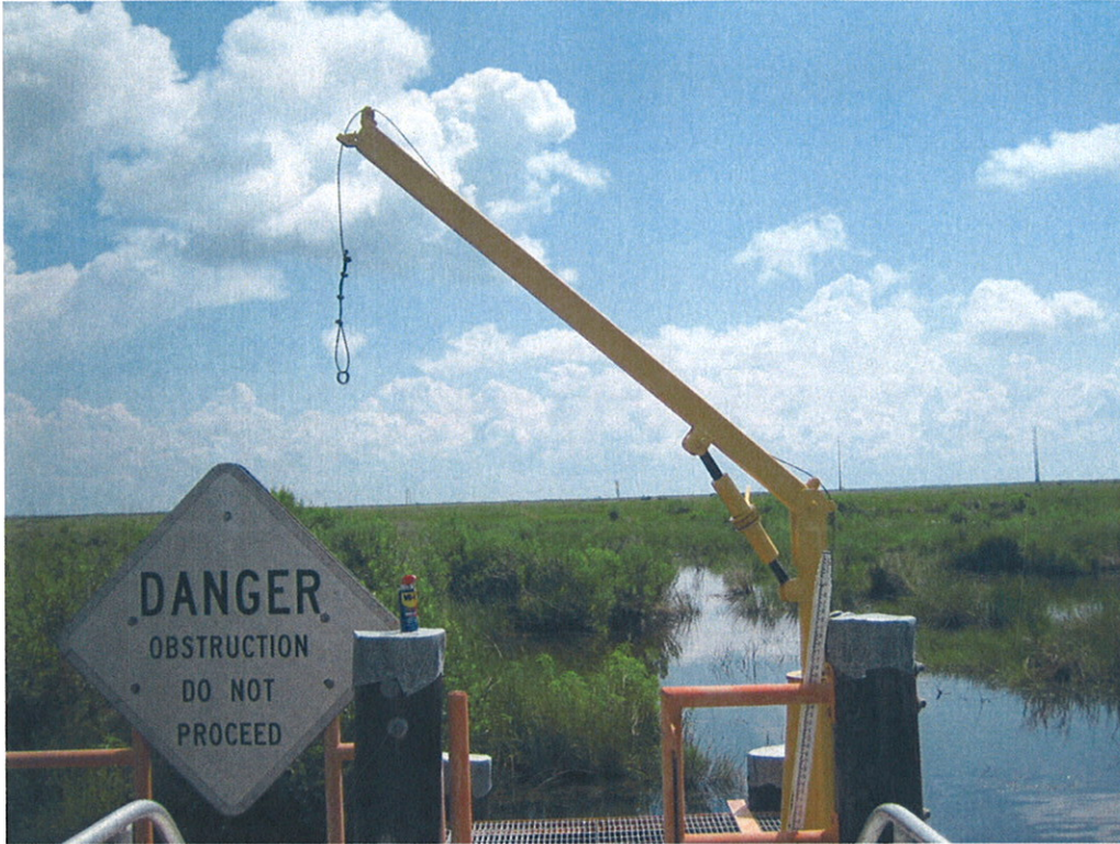
North Side Structure Condition (05-14-09)
