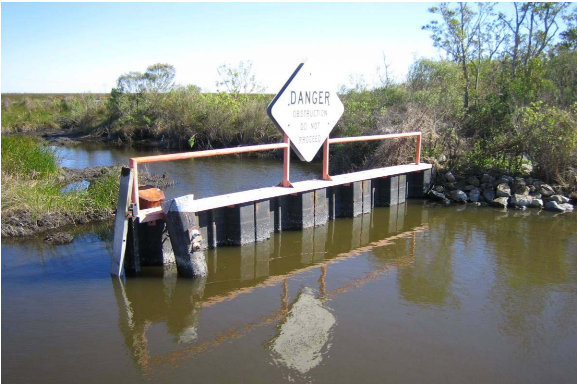
South Side Structure Condition (11-25-08)
