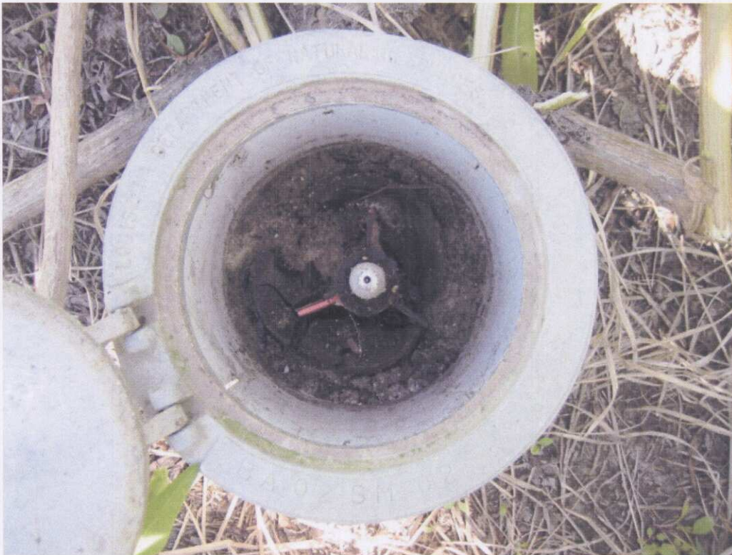
Benchmark Overall Condition (4-30-08)
