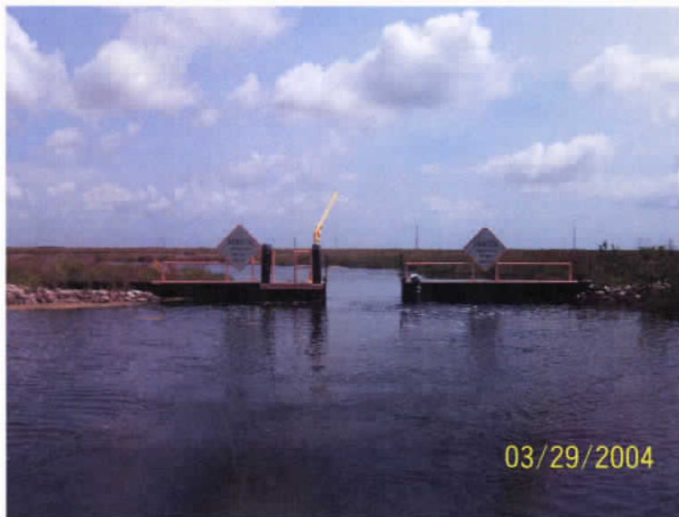
Post Stop Log Installation
