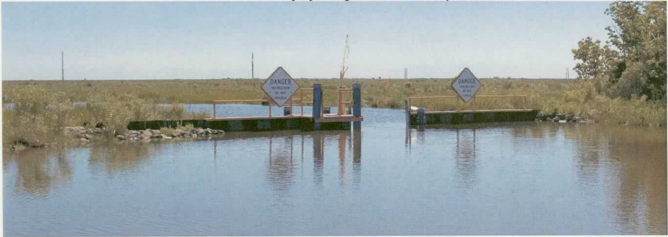
Water Control Structure Condition (4/12/05)
