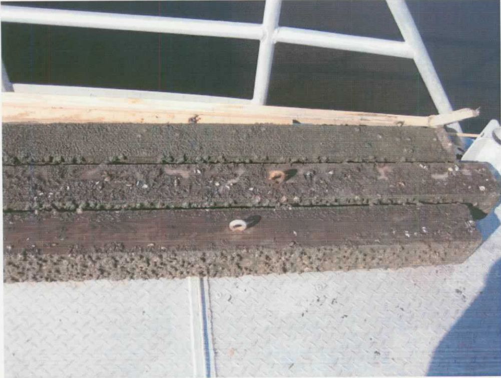
Stop Log Condition Post-removal (11-8-07)
