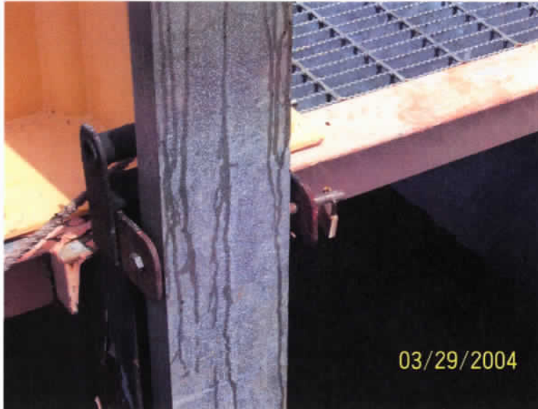
Post Stop Log Installation with New Lock
