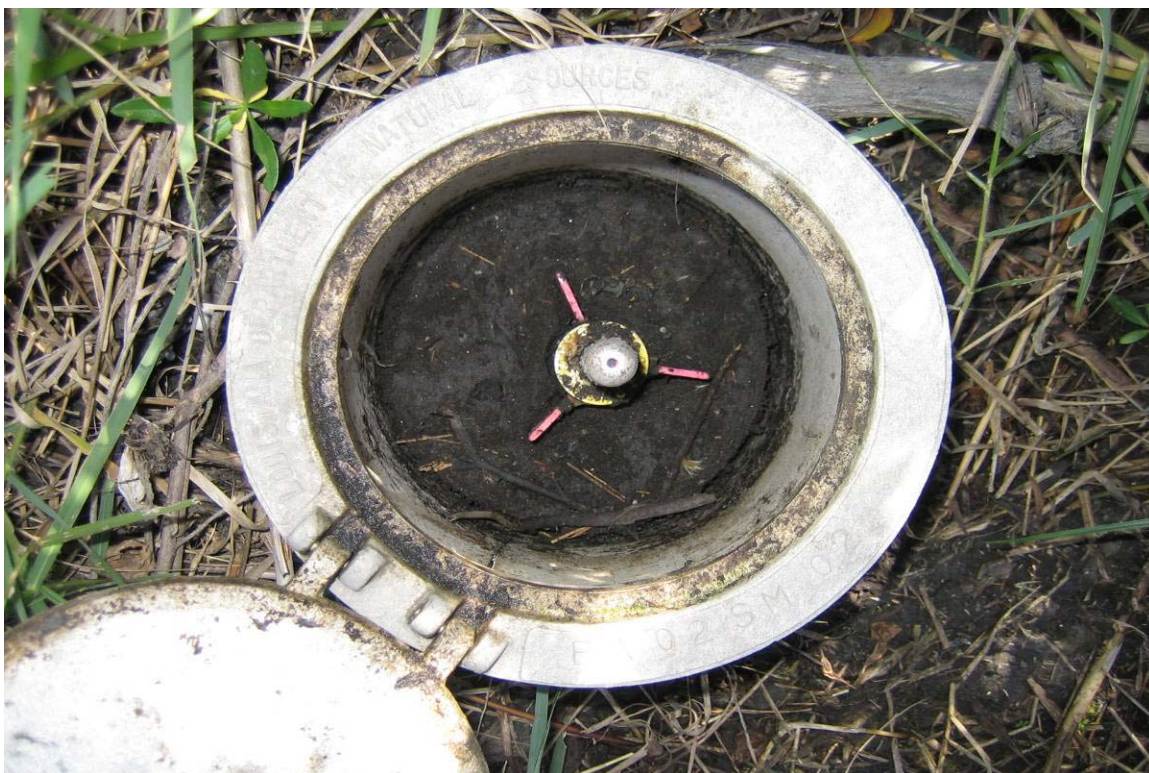
Benchmark Overall Condition (11-25-08)
