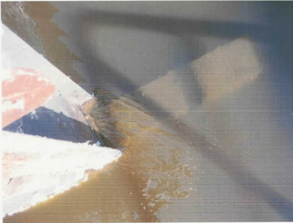
Condition of Stop Logs Pre-removal (11-8-07)
