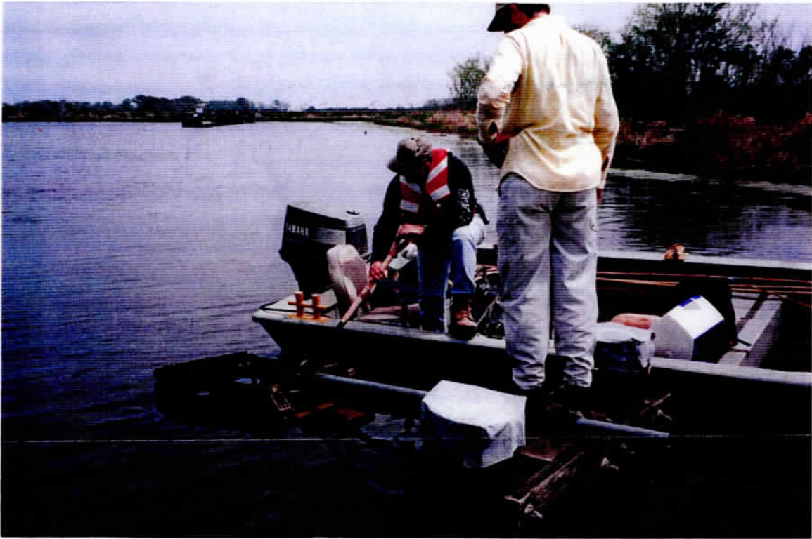
Photo 7 – Flapgated Culvert Structure (Site 91), view of operation check.
