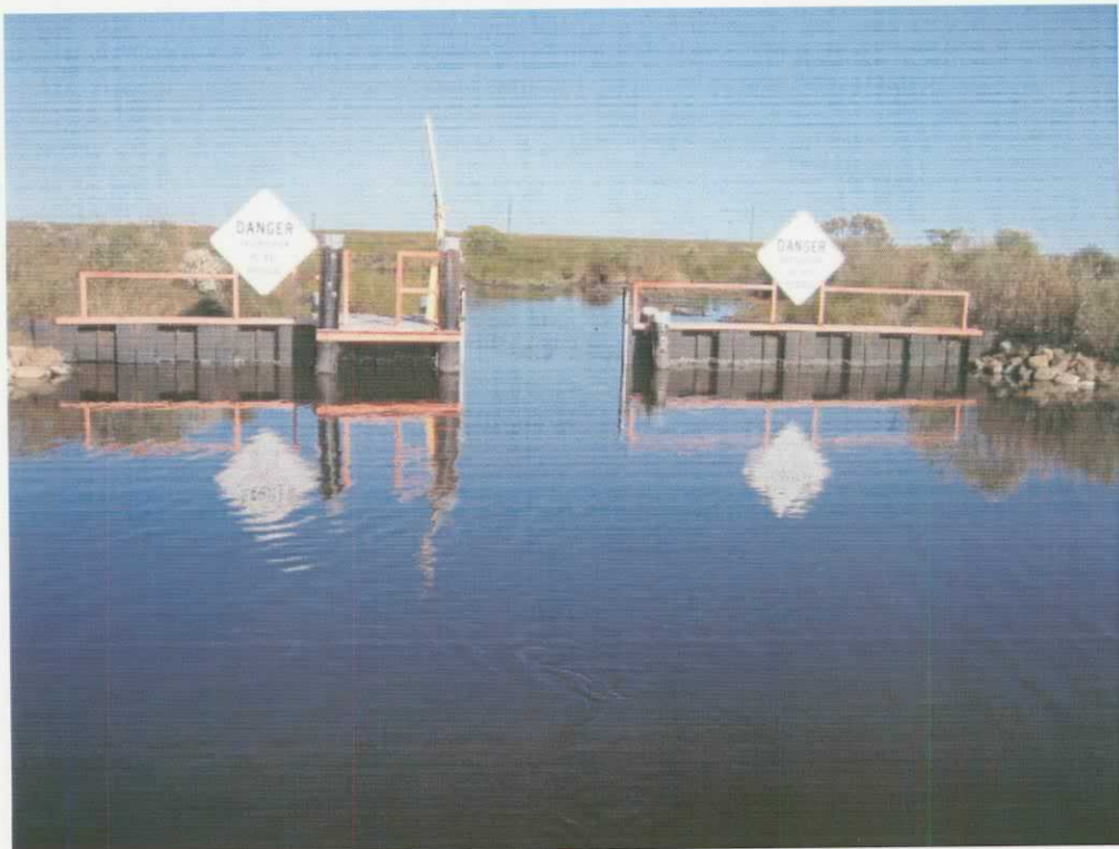
Overall Structure Condition (11-8-07)
