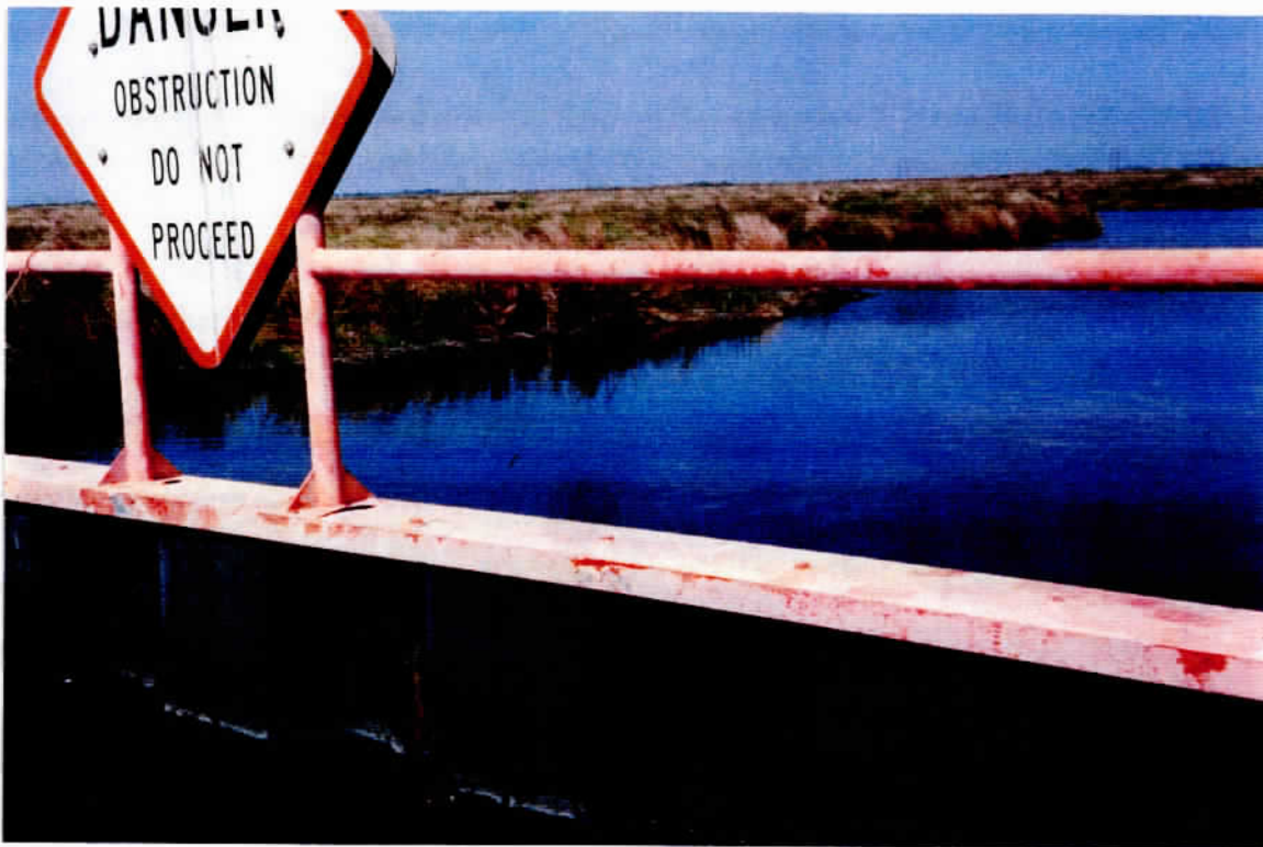
Photo 12 – Variable Crest Weir (Site 35), view of worn and chipped paint on the railing and weir.
