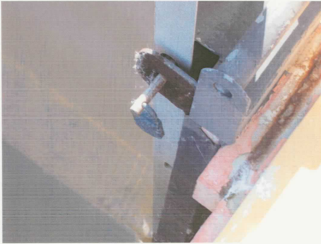
Pin and Lock Condition (11-8-07)
