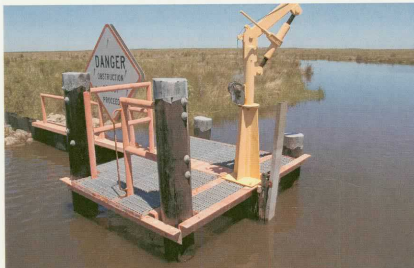
Grating/Metal Components & Pile Caps Condition (4/12/05)
