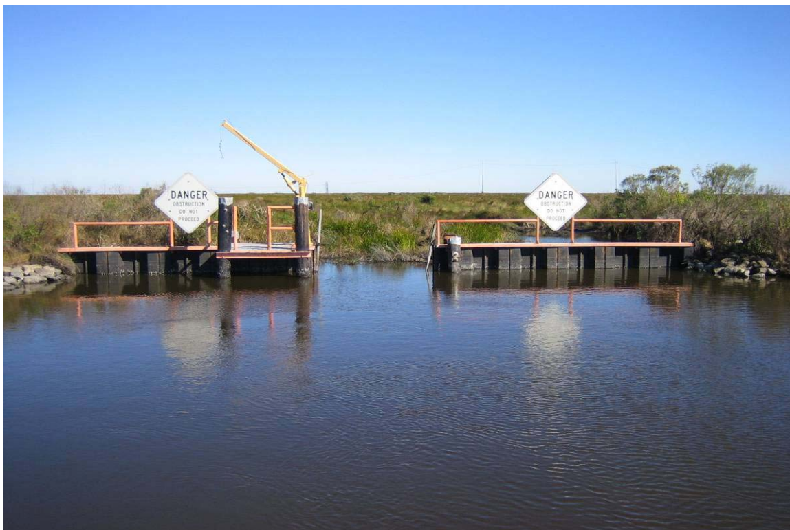
Overall Structure Condition (11-25-08)
