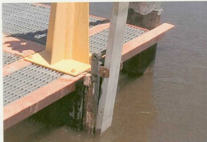
Lock & Slightly Bent Lock Pin (4/12/05)
