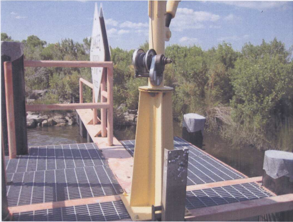
North Side Structure Condition (4-30-08)
