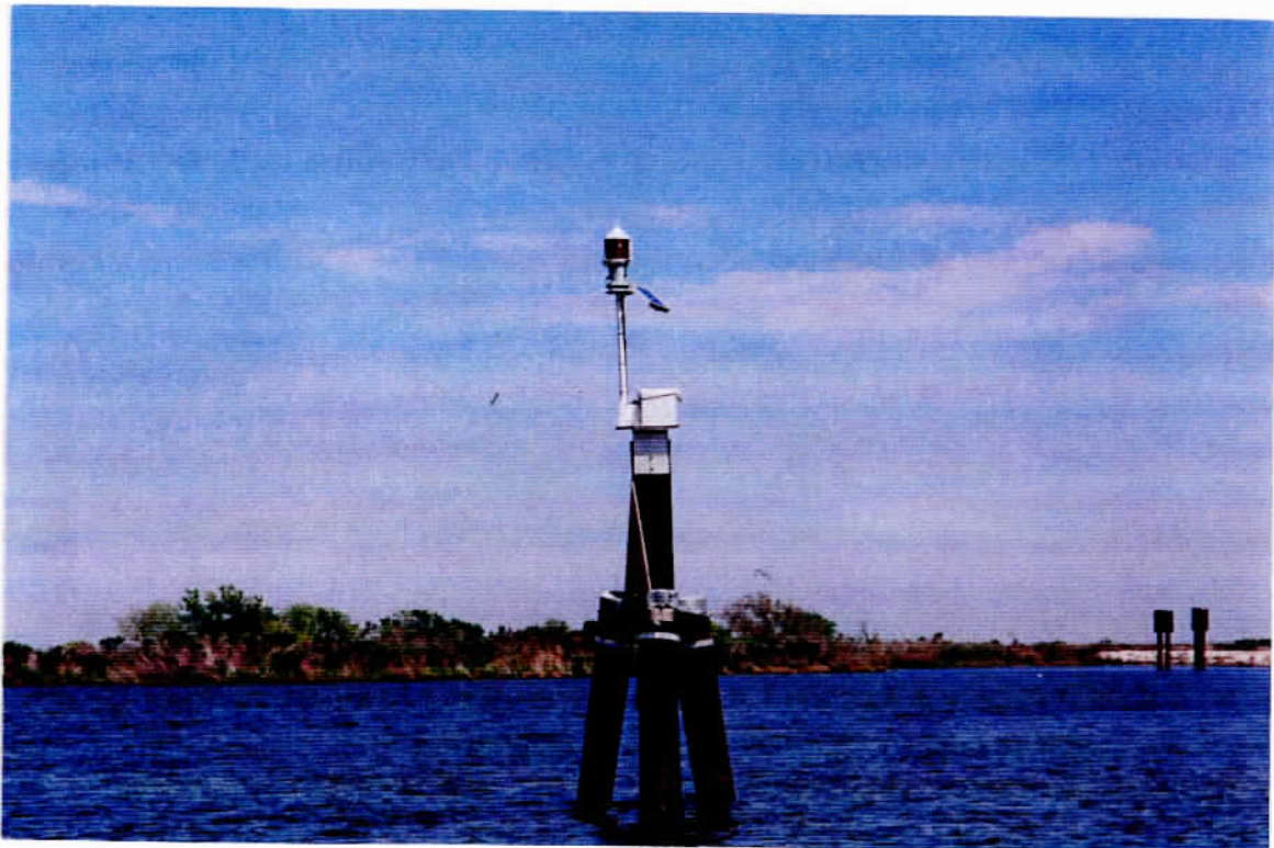
Photo 4 – Navigation Light No. 4 (Site 14a).
